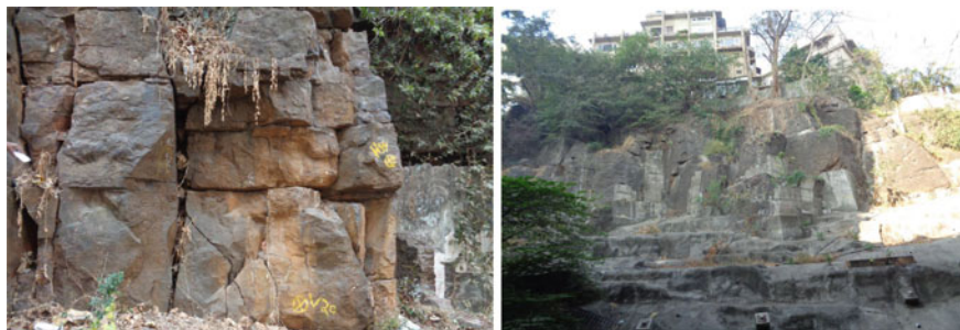
Fig. 1 Present rock slope appearance on out crops from eastern to western corner of the slope a dominant joint sets, discoloration, and staining of rock material due to weathering clearly visible b already stabilized portion of the rock slope
