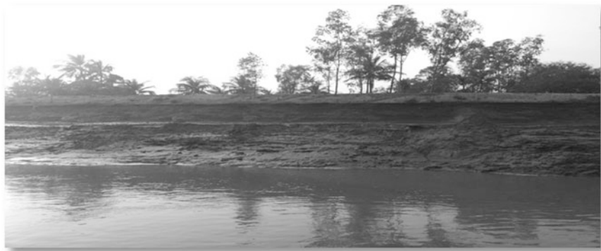
Fig. 1 Typical Sunderban embankment at Sonakhali
