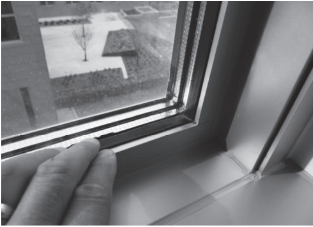
Figure 6-1. Windows with a very low U-value, like this triple pane window, are required to get the heat loss from a space down to a level that it may be maintained by solar heat. (Photo by the author)
