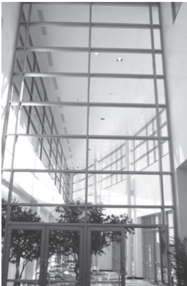
Figure 6-15. Passive solar heating is provided by a sunspace at the Solar Energy Research Facility Building, NREL, Golden, Colorado. (Photo by Warren Gretz, courtesy of DOE/NREL, PIX# 02194)
