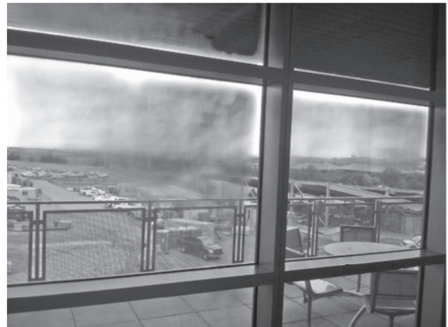
Figure 6-3. The thermochromic glass in these east-facing windows change their transmissivity in response to a change in temperature. The appearance during transition from clear to tinted state is due to temperature differences. Once the transition is complete the appearance is uniform. (Photograph by the author)
