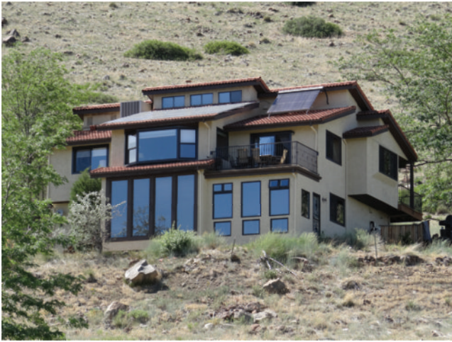
Figure 7-1. Photograph of solar home in Golden, Colorado, with roof-mounted photovoltaics, solar water heating and passive solar features. (Photo by author)
