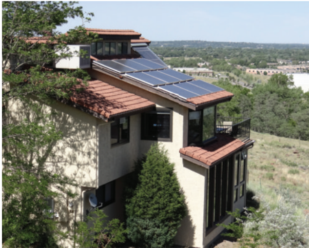
Figure 7-3. Photograph of 2.7 kW STC photovoltaic array on solar home in Golden Colorado. (Photo by the author).
