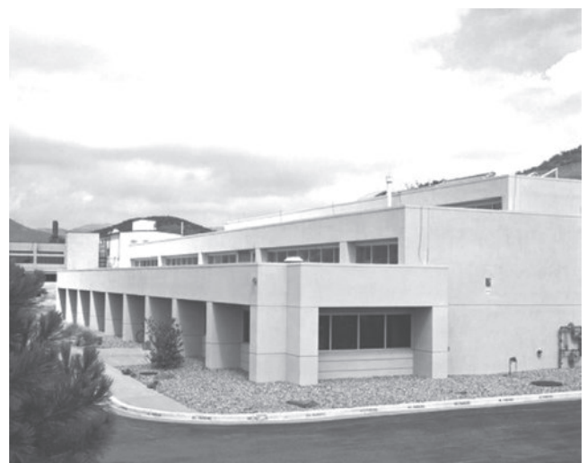
Figure 6-14. Direct-gain passive solar heating at the Thermal Test Facility Building, NREL, Golden, Colorado. (Photo by Warren Gretz, courtesy of DOE/NREL, PIX# 12637)
