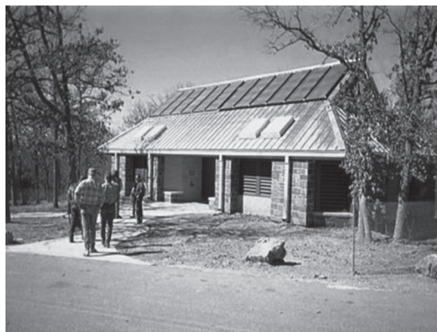
Figure 4-20. Flat-plate solar collectors mounted flush on the roof of a shower and laundry facility at a campground in Oklahoma (Photo by the author)
