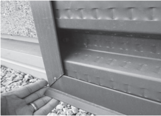
Figure 5-8. Drip edge at the bottom of transpired solar collector. (Photo by the author).
