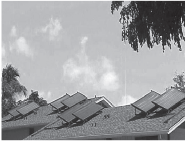
Figure 4-31. Photograph of four of the direct, active, residential solar water heating systems in Honolulu, Hawaii, described in the case study example. (Photograph by the author)
