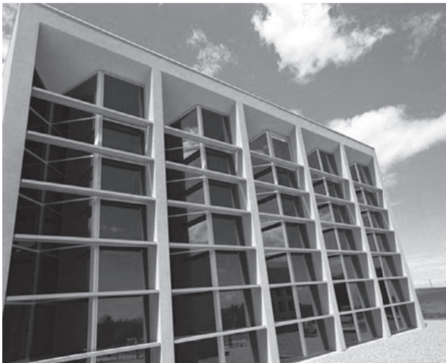
Figure 6-16. Thermal storage wall at the NREL Visitor Center, Golden, Colorado, is articulated with direct gain through view east facing windows and west-facing thermal storage wall elements. (Photo by Warren Gretz, courtesy of DOE/NREL, PIX# 12637)
