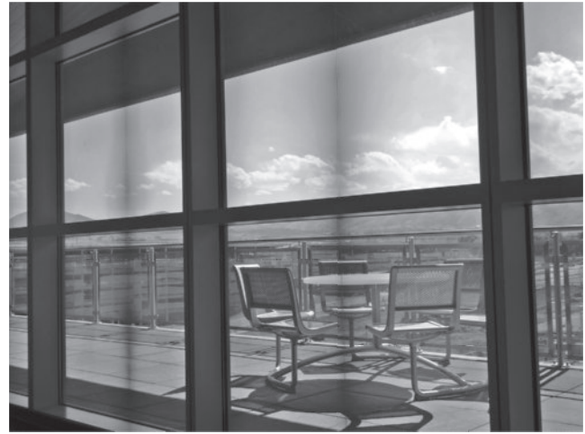
Figure 6-2. The electrochromic glass in these west-facing windows is shown just beginning its transition from clear to tinted state. The change occurs starting in the electrode visible at the center of each pane, once the transition is complete, the appearance is uniform. (Photo by the author)
