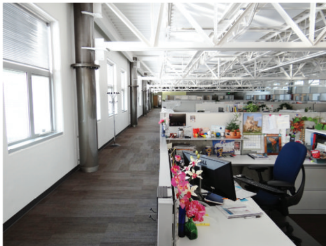
Figure 7-20. Interior offices in RSF1. Direct solar heat gain from the view windows may impinge on the walkway in winter, but not on the work spaces. Daylight through the daylighting windows above the view windows is directed toward the ceiling and deeper into the space by reflective louvers. (Photo by the author)
