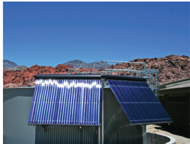
Figure 7-15. Two solar water heating evacuated tube solar collectors are mounted on a 15,000-gallon tank for harvested rainwater storage. (Photo by Henry Tom, AIA, NCARB, courtesy Line and Space LLC)
