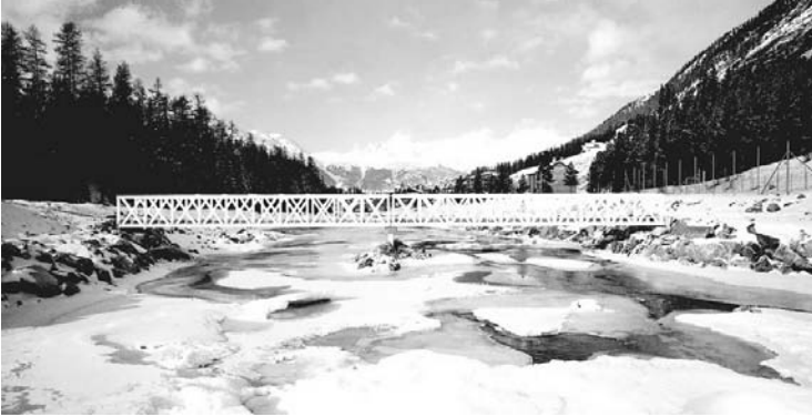
Fig. 58 Pontresina all-composite truss bridge constructed in Switzerland in 1997. (Courtesy of Fiberline Composites A/S)
