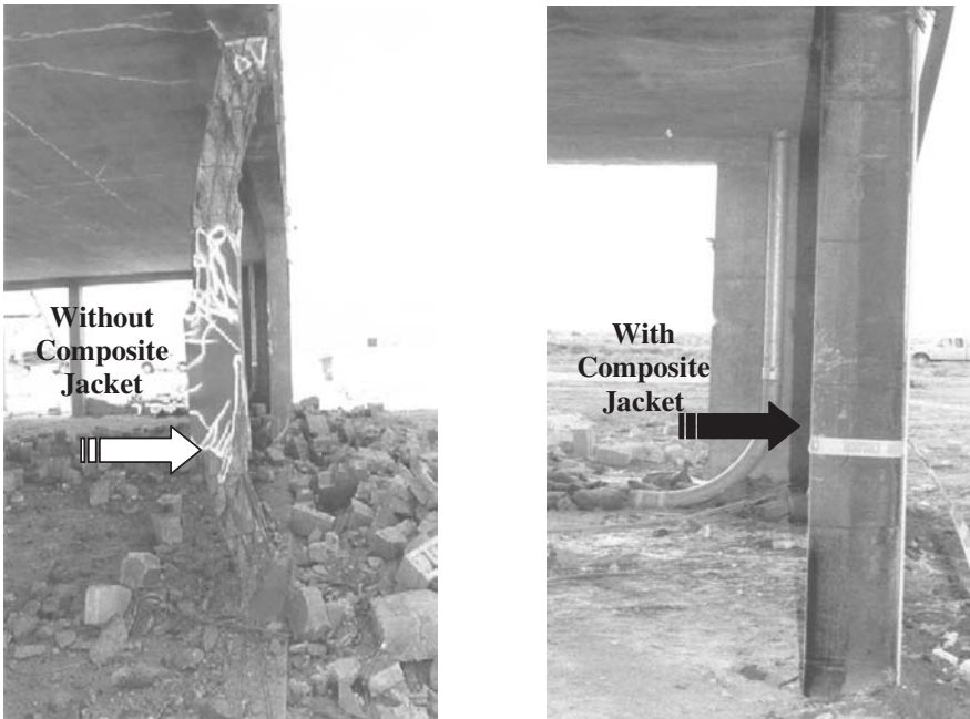
Fig. 18 Blast-resistance enhancement of reinforced concrete structures. [Courtesy of Structural Composites Construction Inc. (SCCI)]
