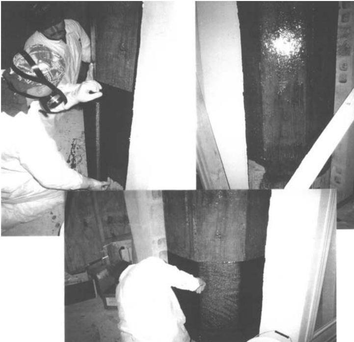
Fig. 1 Seismic upgrade of columns using composites. [Courtesy of Structural Composites Construction Inc. (SCCI)]
