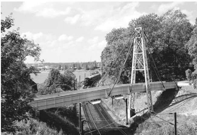
Fig. 57 Fiberline all-composite cable-stayed in Denmark. (Courtesy of Fiberline Composites A/S)
