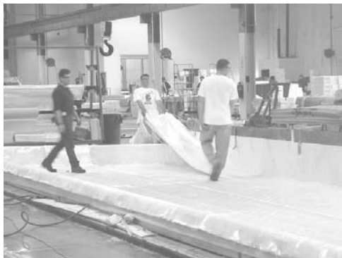
Fig. 50 Fabrication of the FRP composite bridge deck of NY 367 over Bentley Creek, Chemung County, New York. (Courtesy of New York DOT, Region 6, Hornell, NY)
