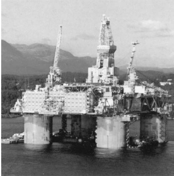
Fig. 12 Demands of the superstructures of offshore oil rigs in high humidity and water exposure are met with 5454, 5086, and 5083 Al-Mg alloy welded construction.
