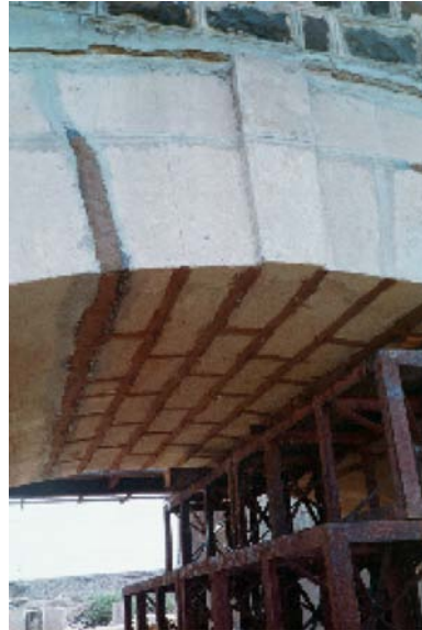
Figure 14. The crown of the arch repaired by resin-injection
