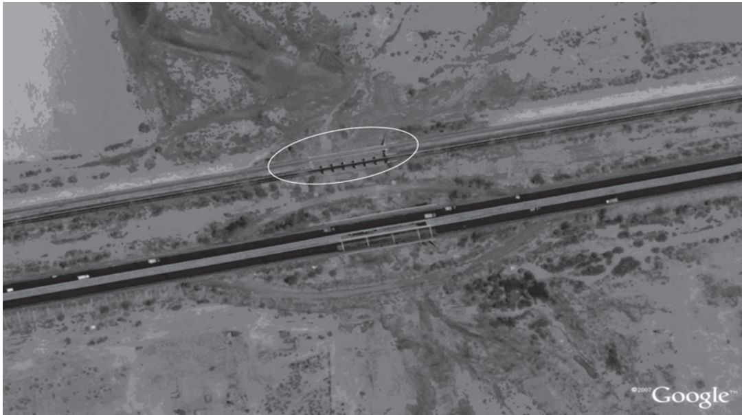
Figure 4. A satellite image of the bridge site
