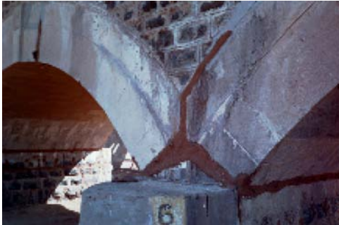
Figure 15. Cracks at thrust lines on support piers repaired by resin-injection
