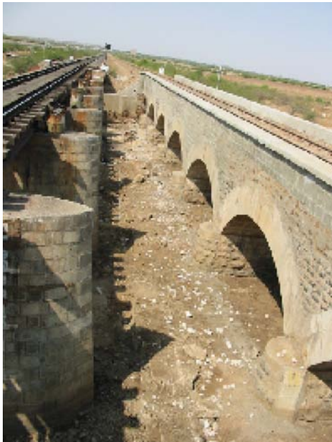
Figure 5. A view of the two railway bridges
