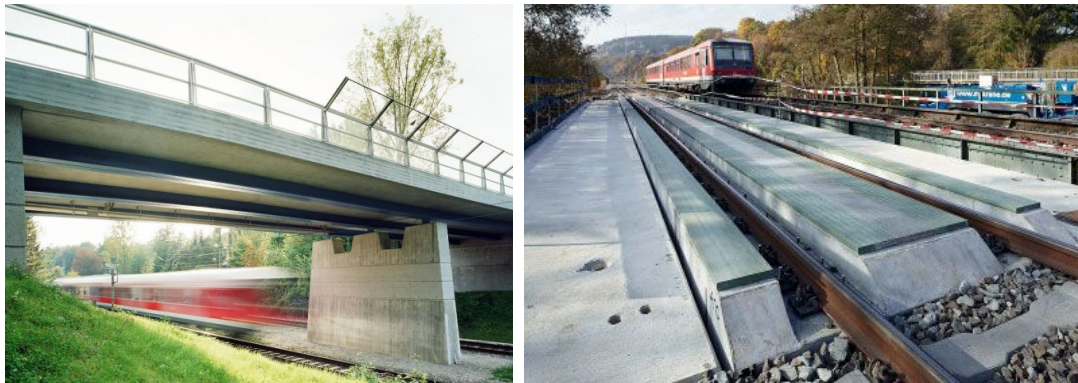
Figure 3. Bridges with composite dowels: road bridge in Pöcking [Seidl 2009] (left) and Simmerbach [Feldmann et al. 2012a] (right).
