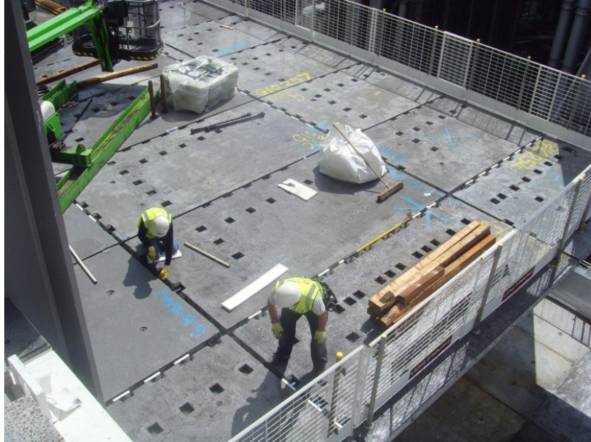
Fig. 14 - Plank assembly at the work-front
