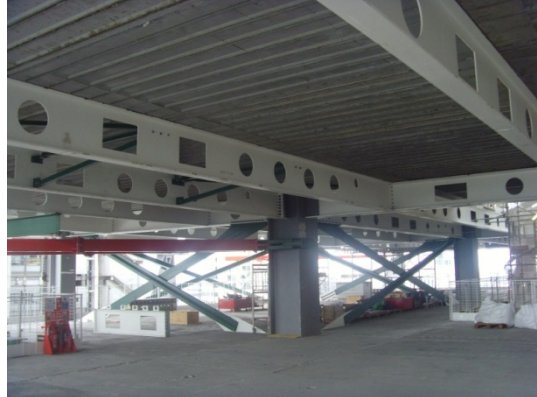
Fig. 16 - View of structural soffit
