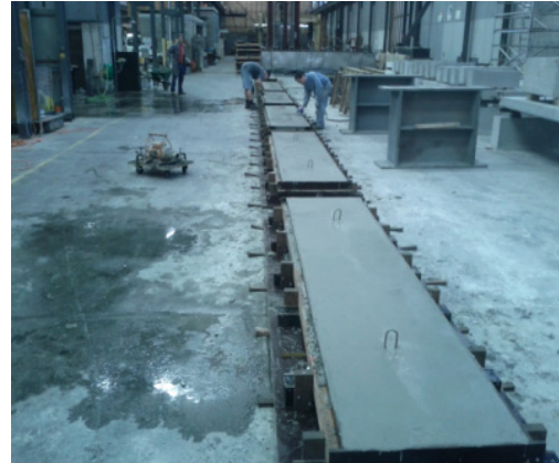
Figure 7: Formwork and slab immediately after casting.
