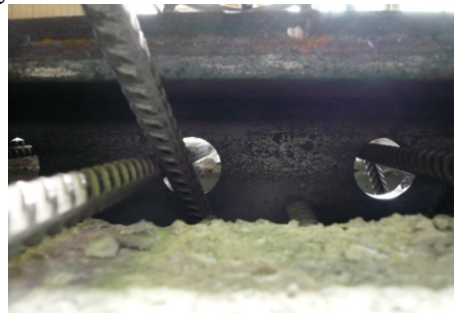
Fig. 3 - Bar through web of section
