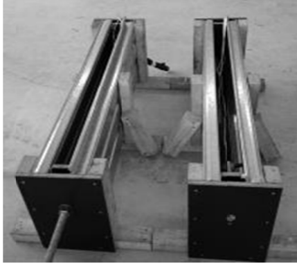
Figure 4. Formwork ready for pouring
