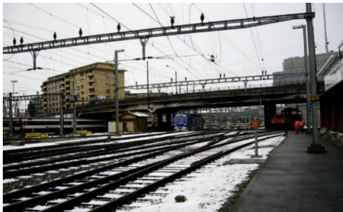
Fig. 3 - Existing old bridge
