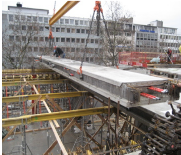
Figure 6. Floor element with sandwich cross section
