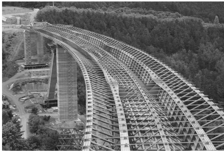
Figure 3. Bridge steel chamber with plate flanges.
