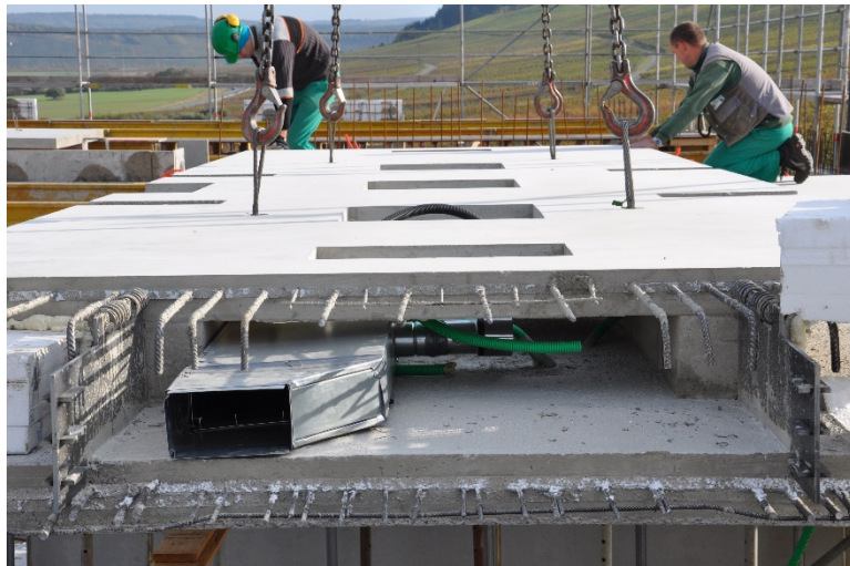
Figure 16. Placing large floor elements with integrated service lines on construction side
