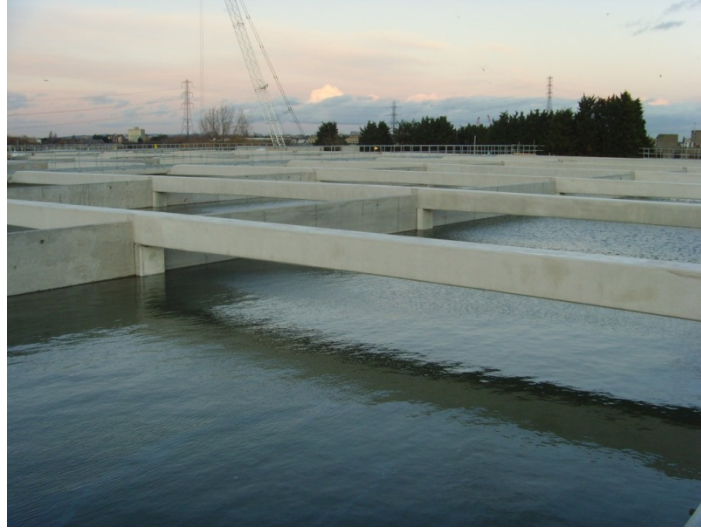
Figure 10 – Filled twinwall water tank at Beckton Sewage Treatment Works
