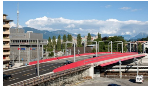
Fig. 2 - New Langensand bridge
