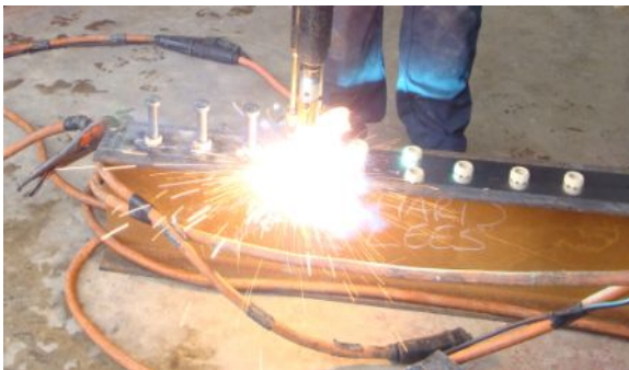
Figure 2. Through deck welding
