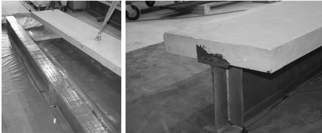
Figure 17. full scale specimen right before and after the connection
