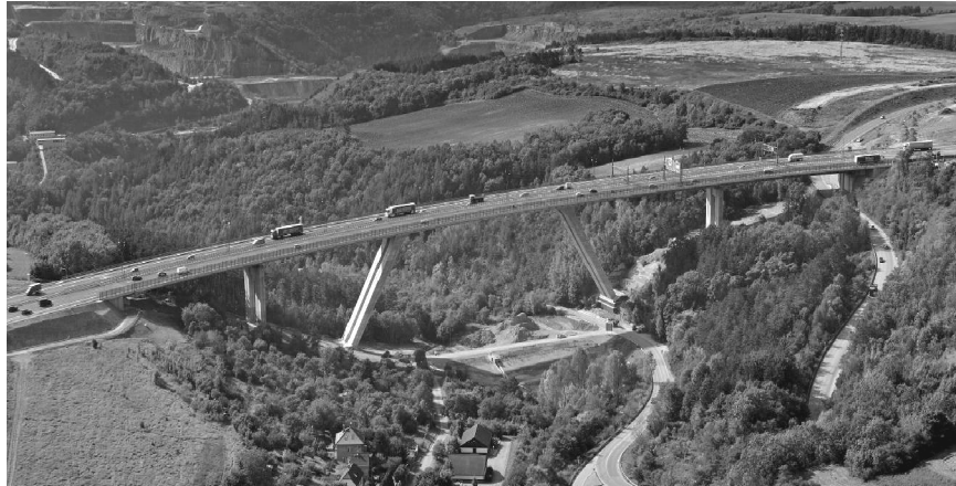
Figure 2. General view on the coupled steel-concrete bridge over the Lochkov Valley.
