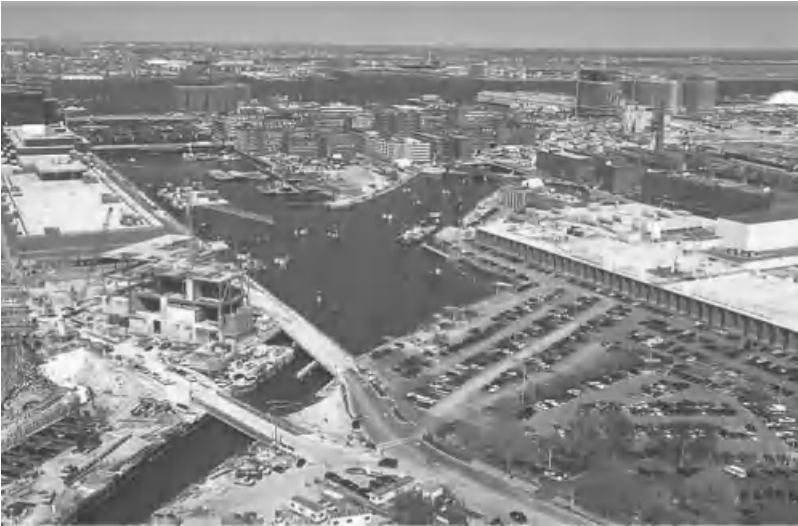
Figure 2.4 Tunnel Box Float-Out Source: Central Artery/Tunnel Project.
