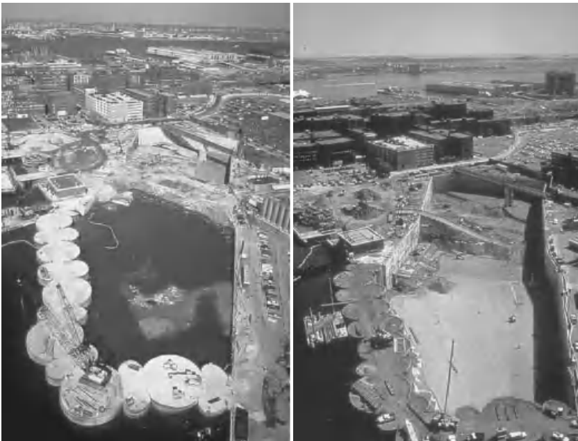
Figure 5.2 Casting Basin Source: Central Artery/Tunnel Project.
