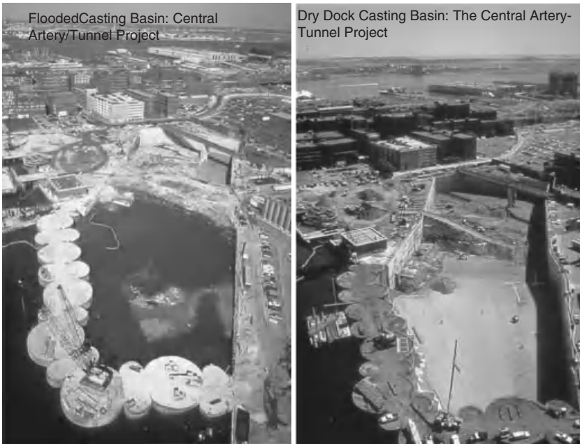
Figure 2.3 Casting Basin Source: Central Artery/Tunnel Project.
