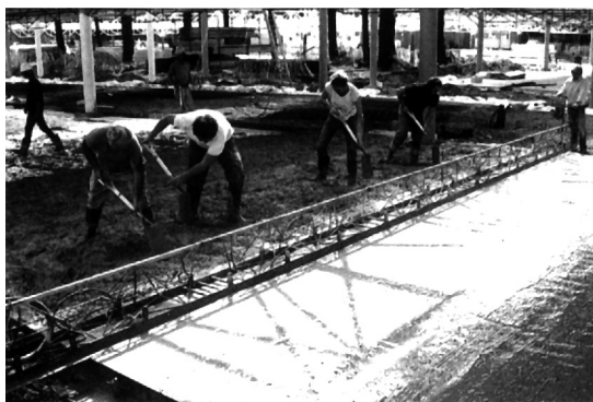
Fig. 2.1. Use of ‘Razorback’ enables greater widths of concrete to be placed
