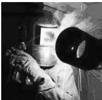
Figure 12.3 Welding of a large diameter pipe
