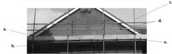
Figure 2.26 Typical scaffolding erection
