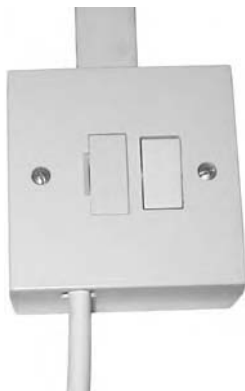
Figure 9.9a Fused spur outlet
