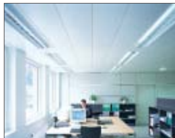
Figure 19 Row of luminaires nearest the window switched off as there is sufficient daylight
