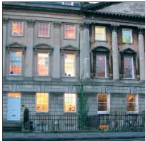
Figure 6 Offices in refurbished building using different lighting styles leads to a poor external appearance
