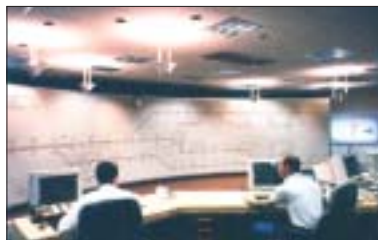
Figure 37 Left: Scheme with combination of direct/indirect and indirect luminaires Below: Scheme with downlighting supplemented by suspended uplighters
