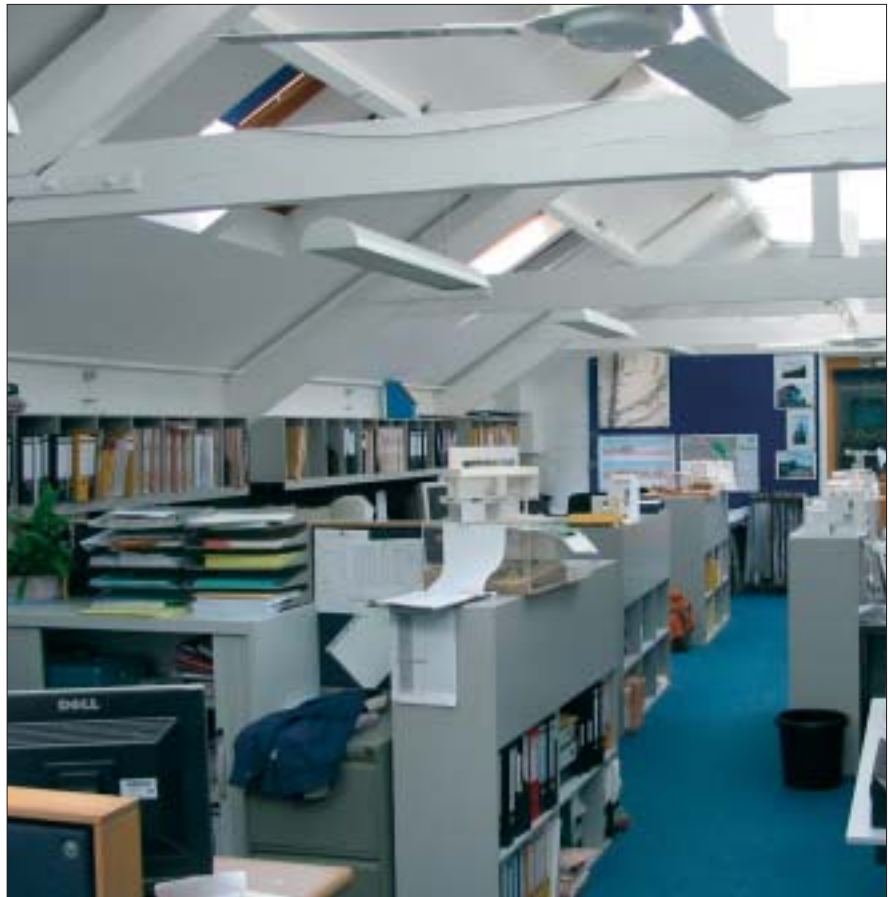
Figure 39 Rooflights with adjustable blinds on sloping windows and louvres on top windows
