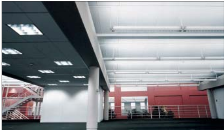
Figure 9 Comparison between direct and combined lighting – note darker ceiling on left with green tinge from reflected light from carpet
