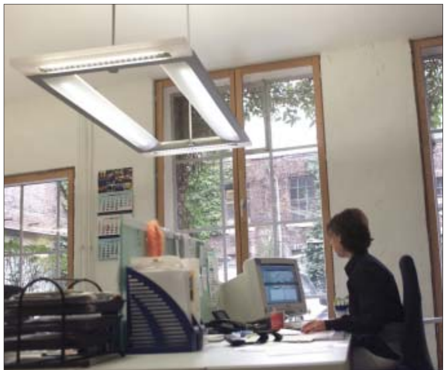
Figure 33 Luminaires hung over desks to provide localised light and avoid obstruction of space and avoid obstruction over circulation space
