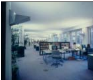
Figure 30 Alternating wall and column mounted indirect lights give a fairly even ceiling luminance
