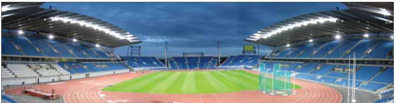
Figure 28 Side lighting to national and international standards, designed to meet requirements for CTV in large sports stadia.
