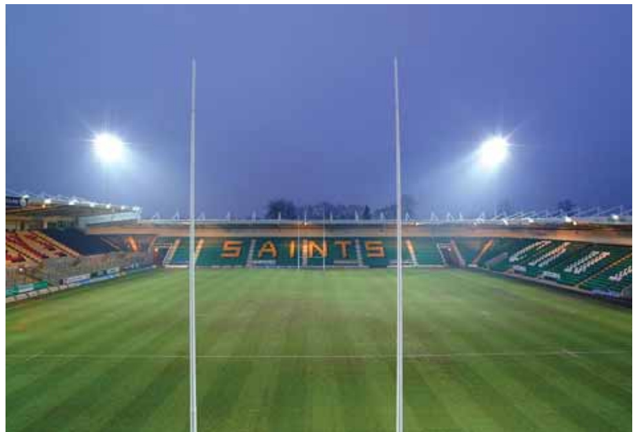
Figure 26 Small sports stadium illuminated using a four-corner mast system.
