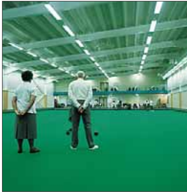
Figure 8 An indoor bowling green showing luminaires parallel to the lines of play.
