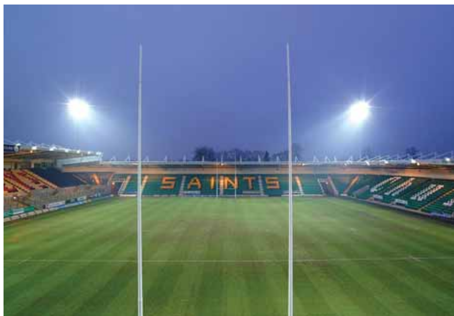
Figure 26 Small sports stadium illuminated using a four-corner mast system.
