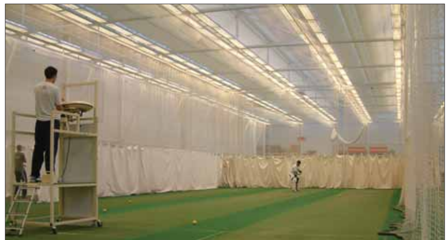
Figure 9 An indoor cricket training facility showing luminaires parallel to the axis of play with the nets being used to reduce glare
