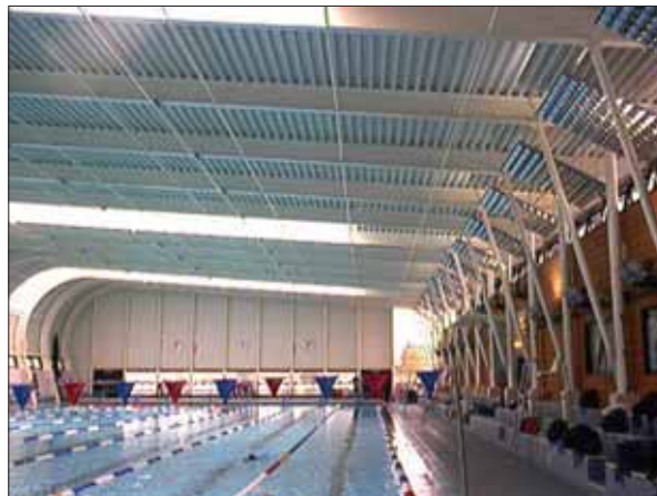
Figure 23 Indoor 50 m swimming pool illuminated by indirect lighting to reduce surface reflections.
