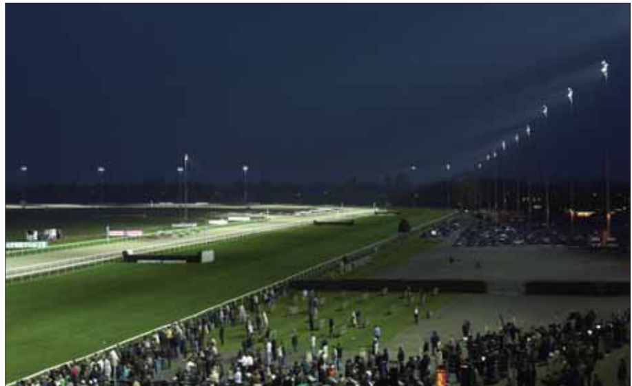
Figure 18 A large horse racing track illuminated using a floodlighting system designed for CTV but with control of obtrusive light.
