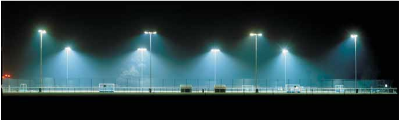
Figure 17 An outdoor hockey pitch illuminated using flat glass floodlights to minimise direct upward light, overspill and glare.
