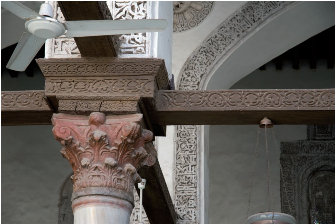
Fig. 9. Mosque of al-Salih Tala'i, wooden tie beams in the prayer hall. (Photo: author)
