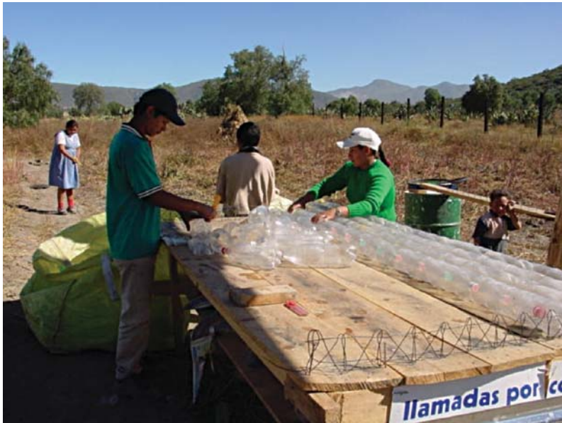
13.8. PET panels construction process. (Source: Author)
