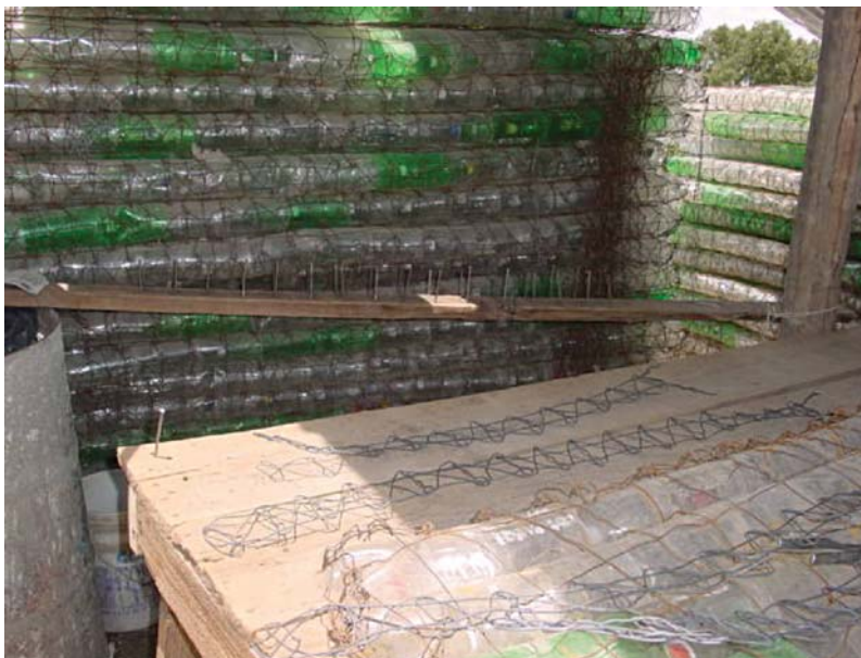
13.2. Construction process of PET modules. Perimeter steel frame and wire enclosure of bottles. (Source: Author)
