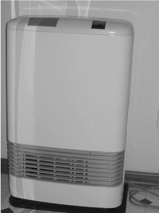
4.6 Balanced-flue gas-fired fan convector.
