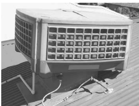
5.2 Ducted evaporative cooler used in hot climates.
