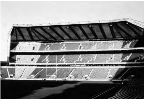
Figure 19.10 The North Stand, Twickenham.
