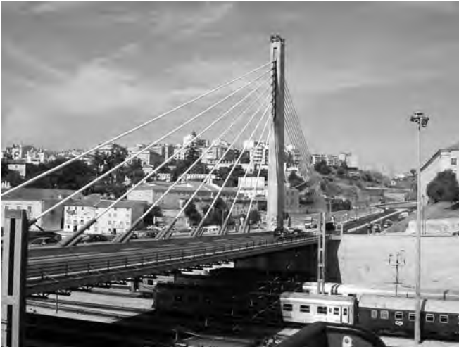
Figure 9.14 A cable-stayed bridge in Lisbon.
