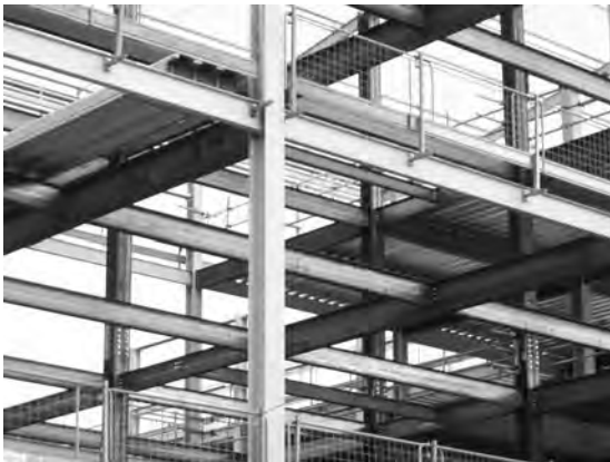
Figure 3.7 A steel-framed building.
