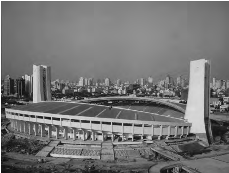
Figure 9.12 Zhejiang Dragon Sports Centre (courtesy of Professor Jida Zhao, China Academy of Building Research, China).
