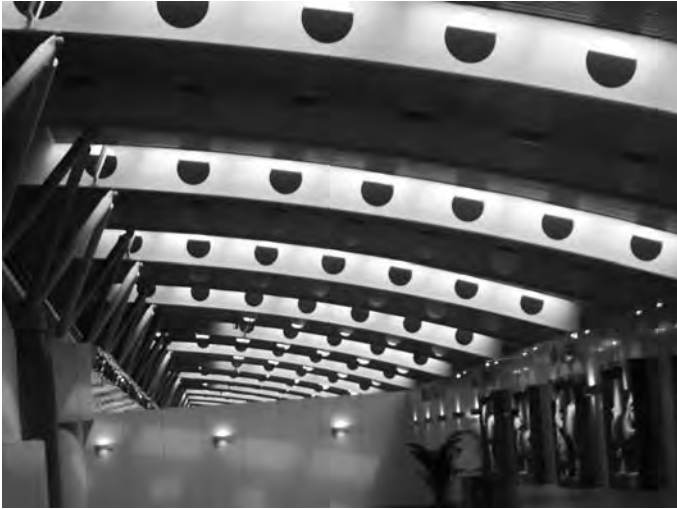
Figure 3.10 Cellular beams.
