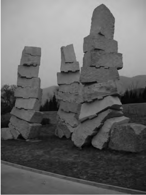
Figure 11.8 Centrally post-tensioned stone columns.
