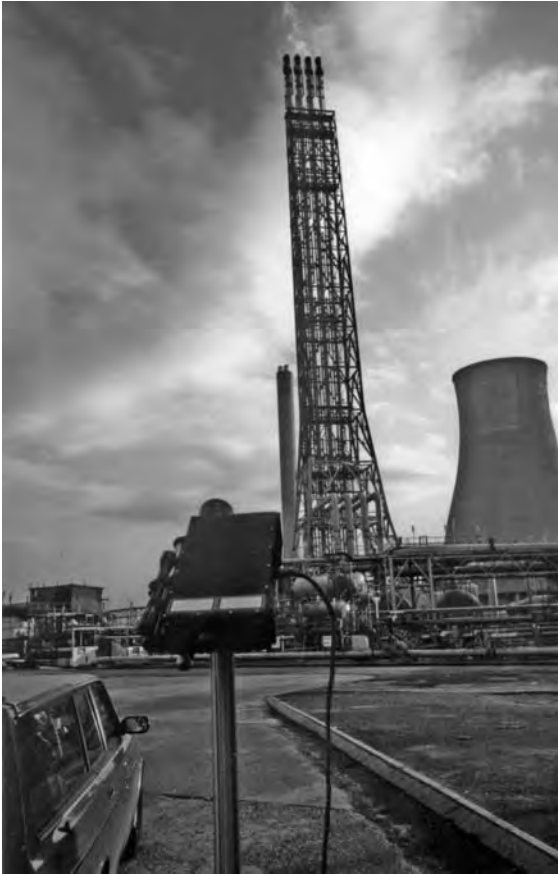
Figure 15.19 A multiflare stack.
