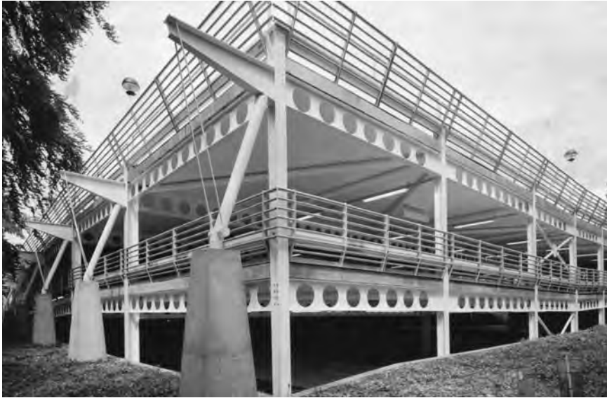
Figure 4.6 Overhangs used to reduce bending moments and deflections (courtesy of Mr J. Calverley).
