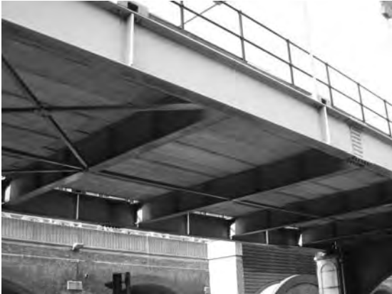
Figure 3.8 A railway bridge.
