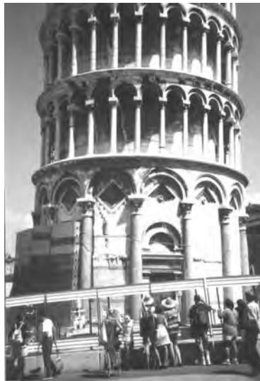
Figure 6.6 Lead blocks used to reduce the uneven stress distribution on foundation.
