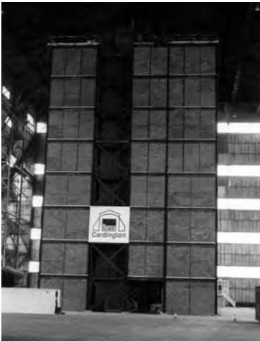
Figure 5.12 Shear walls in a steel-framed building.
