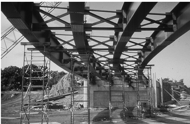
Fig. 6.2 Curved girder bridge erection bracing.
