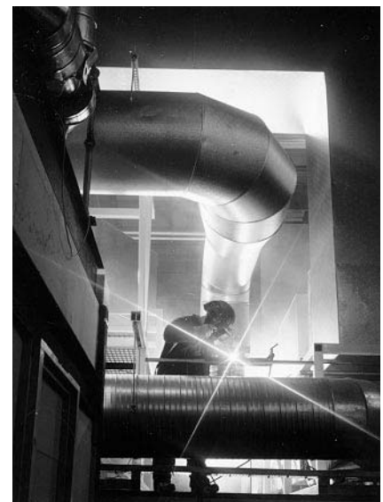
Figure 2.50 The air conditioning systems test facility under construction at BRE
