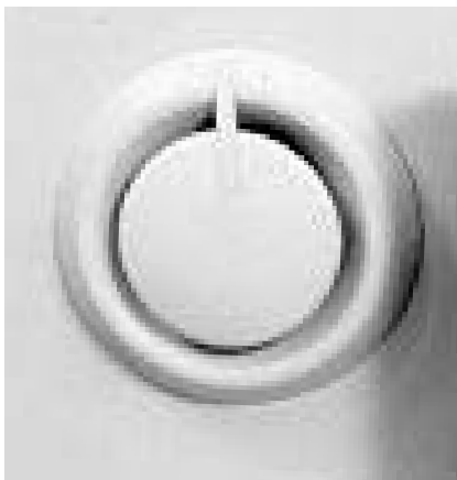
Figure 2.49 An air supply terminal: a form of register, set into a wall, comprising a cone which moves in and out of a nozzle to allow greater or less airflow
