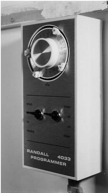
Figure 2.37 Programmers can take many forms. This one dates from the early 1970s. More recent models tend to be digital rather than electromechanical
