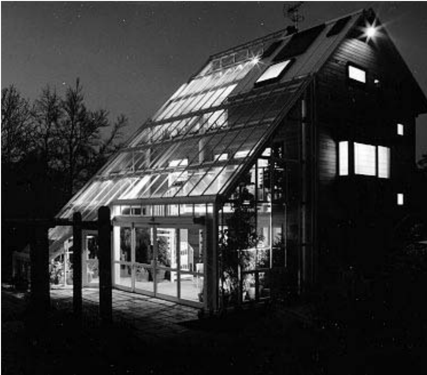
Figure 2.55 A conservatory can provide useful passive solar gains, heating the internal structure of the building for re-emission during the hours of darkness
