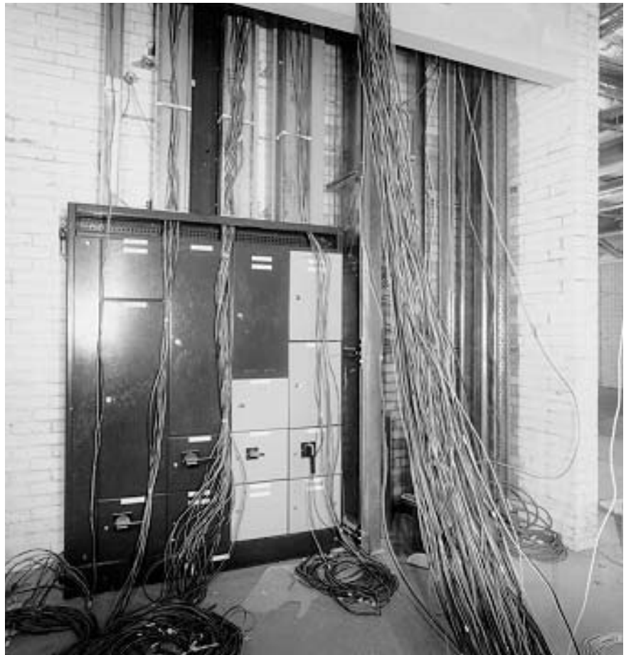
Figure 5.1 Wired services being installed in a large multi-storey building
