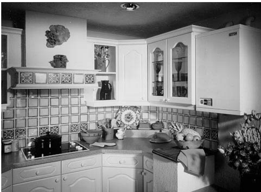
Figure 2.38 A wall hung condensing boiler (far right) integrated into a kitchen layout. In domestic situations the boiler can be sited in the most convenient position (Photograph by permission of Keston Boilers)
