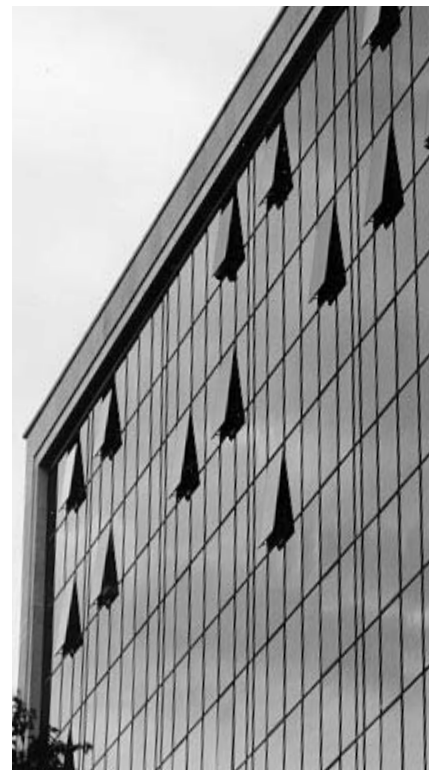
Figure 3.6 Natural ventilation in a multi-storey office building
