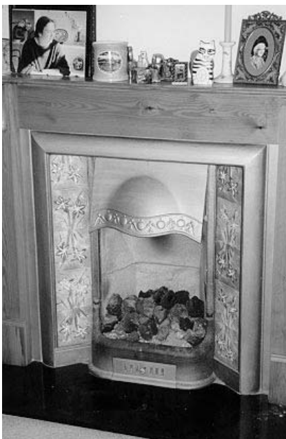
Figure 2.11 This Edwardian cast iron fireplace has a tight fitting fret to allow better control over the rate of combustion
