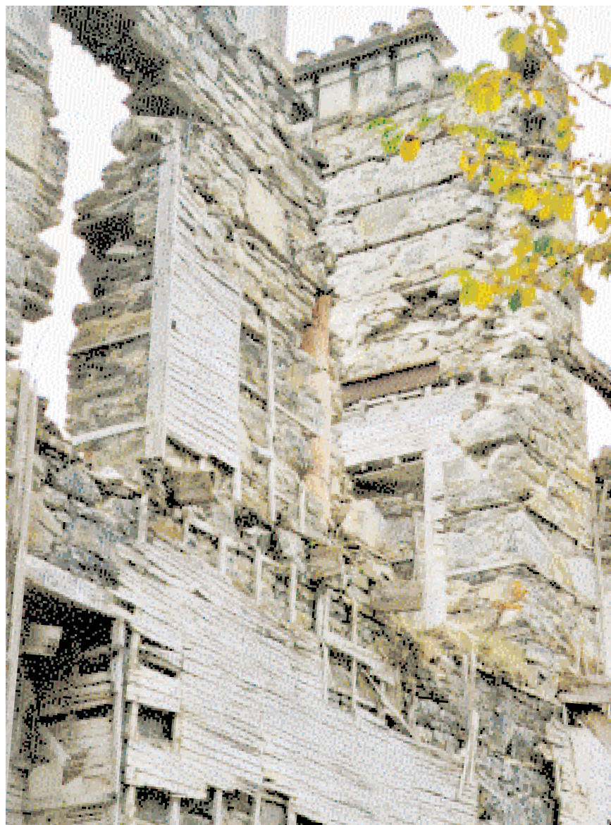
Figure 2.17 The side of the stack (centre of picture) has fallen away in this view of the ruins of Guisachan House, Inverness-shire, and the ceramic chimney liners (reddish colour) have been exposed to view. The house had been built in the third quarter of the nineteenth century
