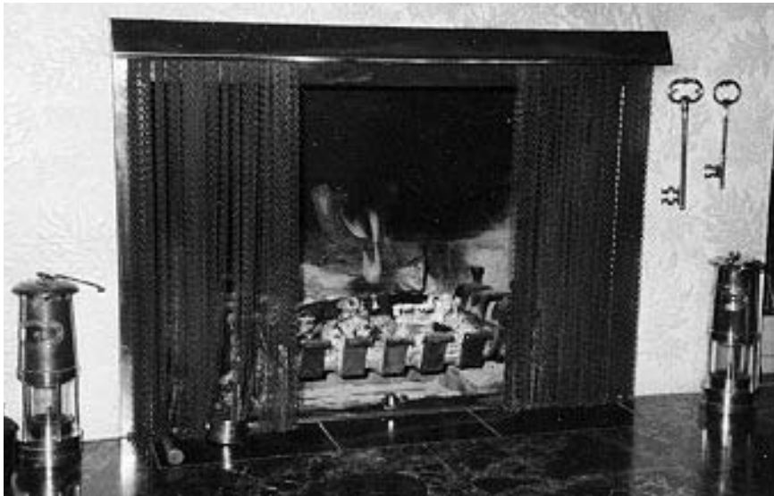
Figure 2.15 The metal mesh curtain of this individually designed screen is both decorative and, when pulled across, prevents flying sparks
