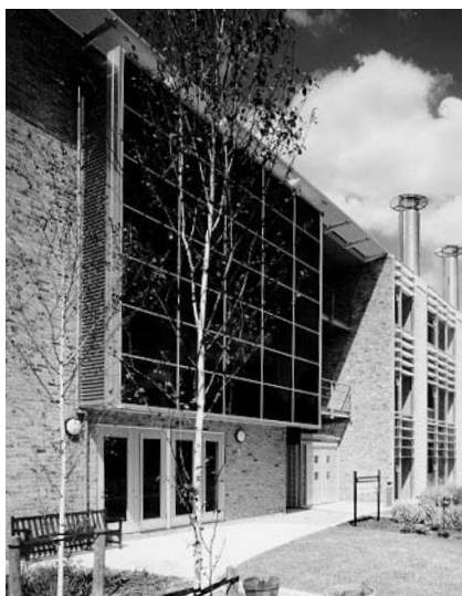
Figure 2.59 Photovoltaic installation on the BRE Environmental Building. A comparatively large surface area is needed to produce a significant amount of power, especially during winter conditions
