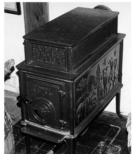
Figure 2.5 A wood burning closed stove without boiler imported into the UK from Norway and installed in the 1970s
