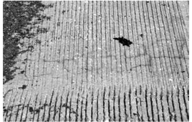
Fig. 3.8(a)—Pattern cracking.
