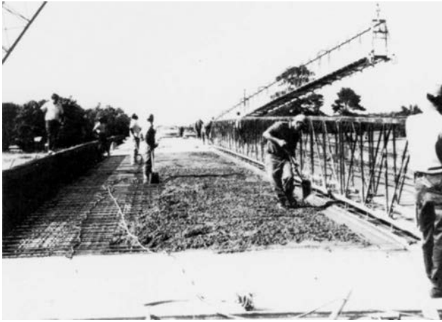
Fig. 6.2.5.1.3—Transverse travel, longitudinal finish screed.
