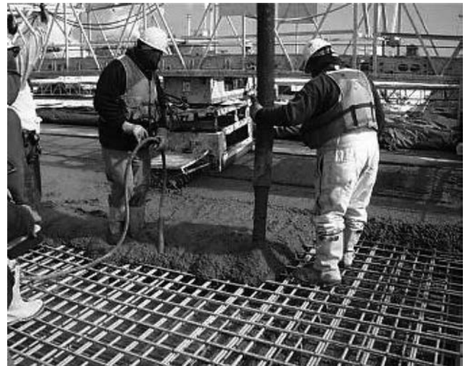
Fig. 6.1.4.1—Placement of concrete using a pumpline.
