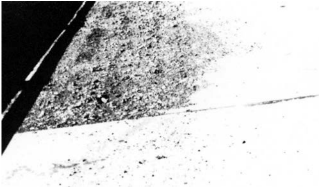
Fig. 4.10—Surface scaling.
