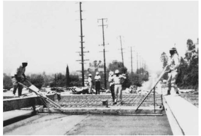
Fig. 6.2.3—Longitudinal floating of bridge deck with bull float.
