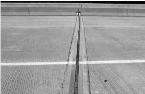
Fig. 3.7.4—Typical strip seal joint system in service.
