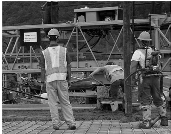
Fig. 6.2.5.1.2(b)—Close-up of transverse finishing element on screed.
