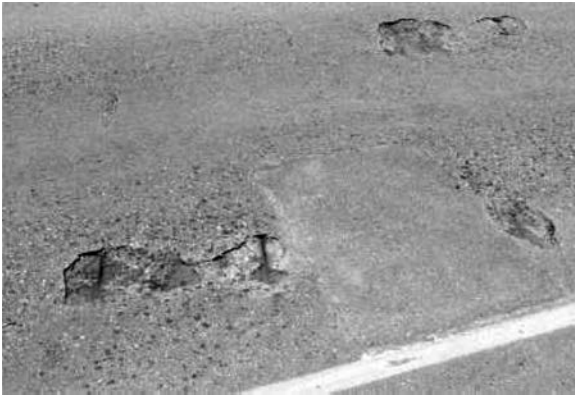
Fig. 5.1.1—Surface spalling.
