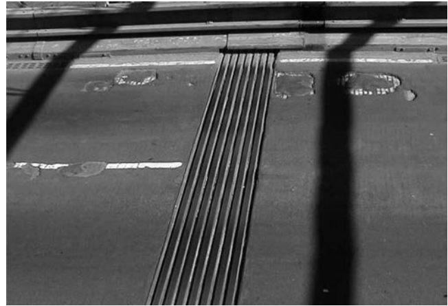
Fig. 3.7.7—Example of modular joint system.
