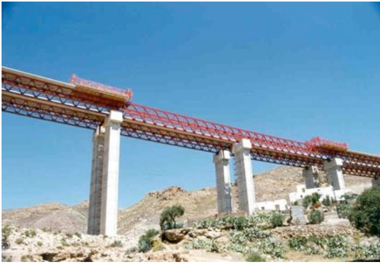
Fig. 7-11. Traveller for a slab on a composite deck. Courtesy of PERI.
