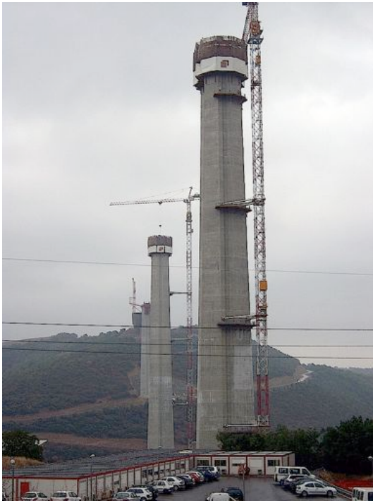
Fig. 6-3. Self-climbing form in Millau Bridge. Courtesy of PERI.
