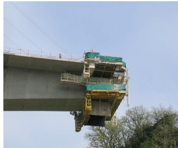
Fig. 7-30. Principle of underslung traveller. Courtesy of Bouygues Travaux Publics.
