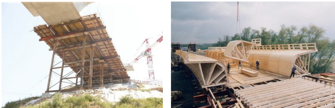
Fig. 6-1. Traditional formwork. Courtesy of Bouygues Travaux Publics.
