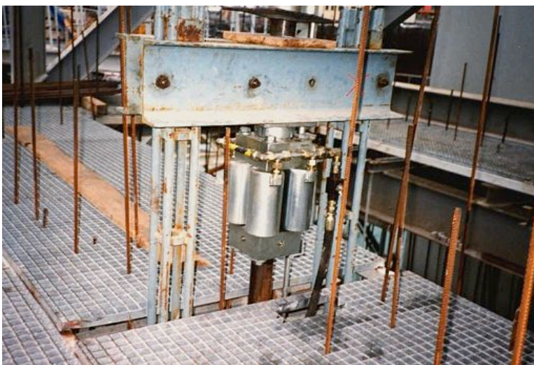
Fig. 6-8. Yoke and hydraulic jacks. Courtesy of Edytesa.
