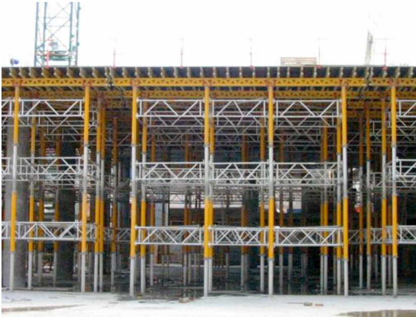
Fig. 7-42. With taller props special bracing must be provided. Courtesy of PERI.
