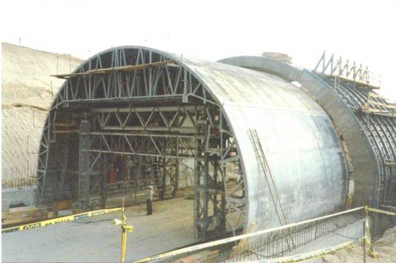
Fig. 7-13. Vault traveller for the cut and cover method. Courtesy of Alcor.
