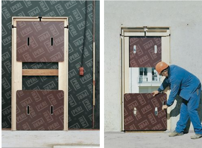
Fig. 3-5. A proprietary box-out system. Courtesy of PERI.
