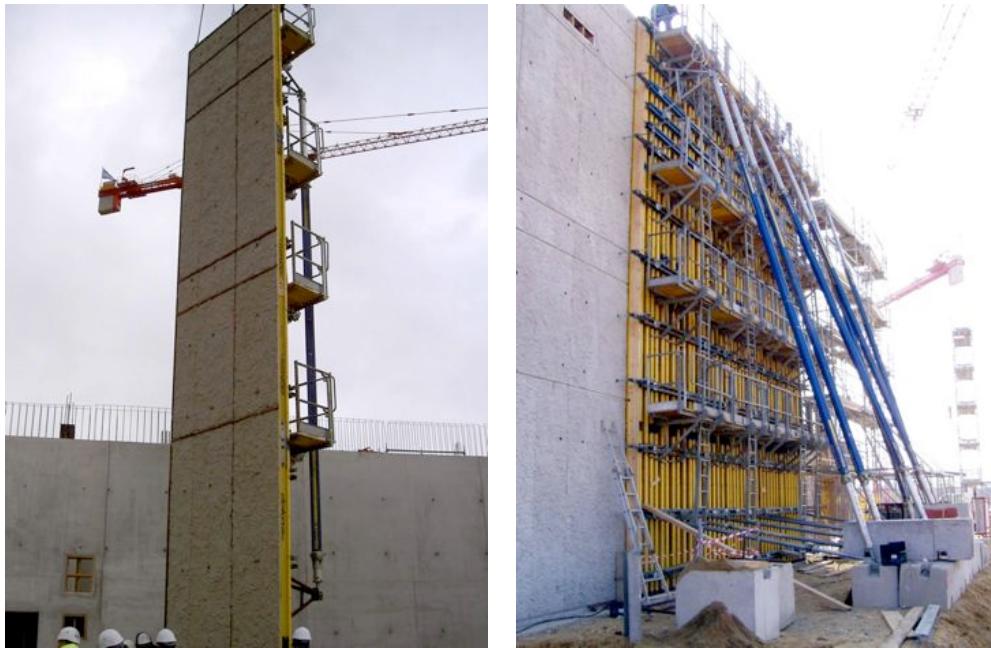
Fig. 6-2. Proprietary formworks. Courtesy of Bouygues Travaux Publics.
