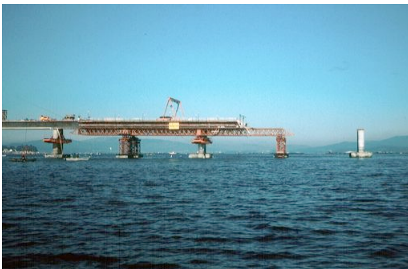
Fig. 7-26. Traveller with intermediate supports. Courtesy of Ferrovial-Agroman.
