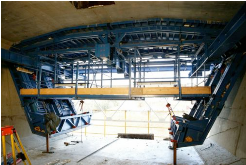
Fig. 7-33. Internal formwork. Courtesy of Setra/CTOA, Gerard Forquet.
