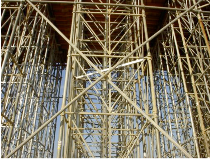
Fig. 7-6. Bracing. Courtesy of Ferrovia-Agroman.
