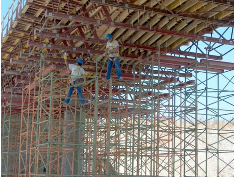
Fig. 3-4. Working before permanent access installation. Courtesy of Ferrovial-Agroman.
