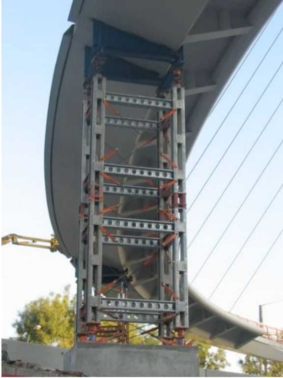
Fig. 7-52. Bearing a composite bridge during assembly. Courtesy of RMD.
