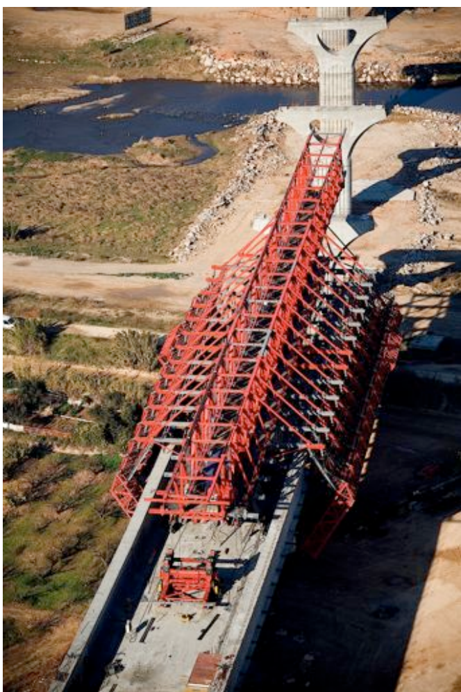
Fig. 7-27. Over-head traveller, opening its formwork. Courtesy of Acciona.
