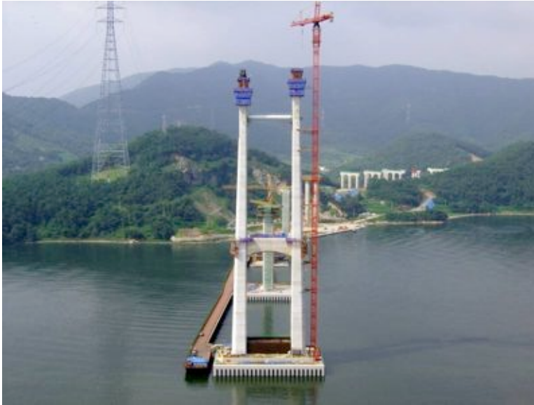
Fig. 6-7. Slip formwork for Machang Bridge. Courtesy of Bouygues Travaux Publics.
