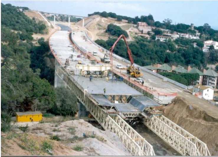
Fig. 7-17. Underslung traveller, cast in place. Courtesy of Ferrovia-Agroman.
