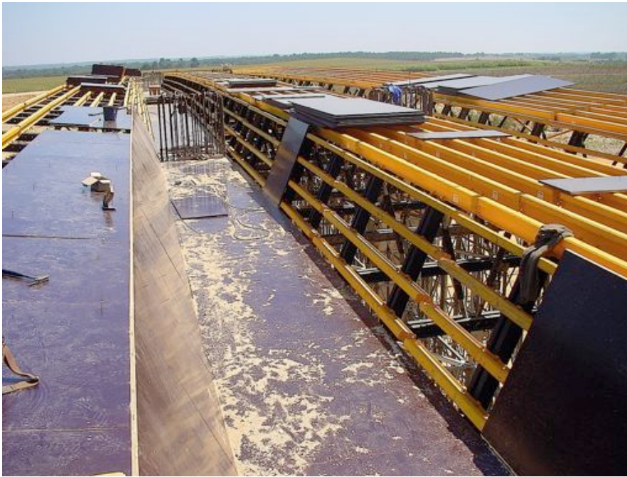
Fig. 7-3. Different parts of this type of falseworks.
