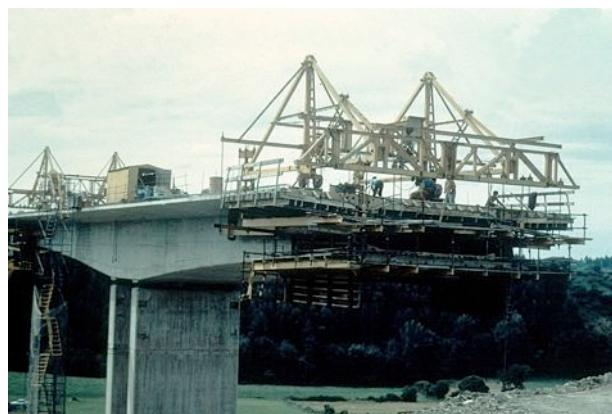
Fig. 7-29. Overhead cantilever formwork with back tie. Courtesy of Ferrovial-Agroman.
