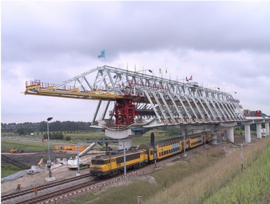
Fig. 7-19. Over-head traveller. Notice the system to bear the formwork keeping free the space over the deck. Courtesy of BAM Civil.
