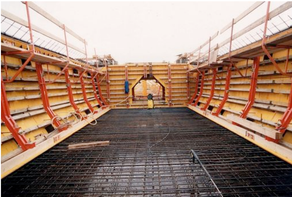
Fig. 7-1. Formwork for incremental launching decks. Courtesy of Setra/CTOA, Gerard Forquet.
