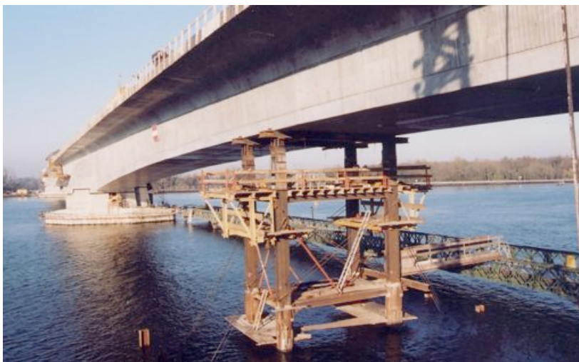
Fig. 7-50. Tower as temporary support. Courtesy of Setra/CTOA, Gerard Forquet.
