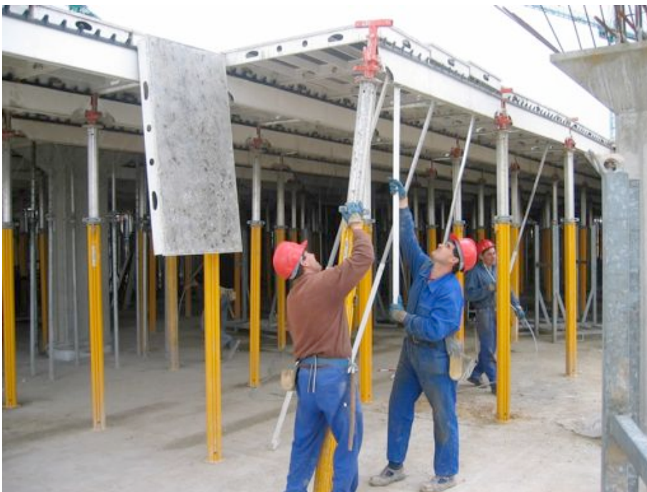
Fig. 7-43. Disassembling. Courtesy of PERI.
