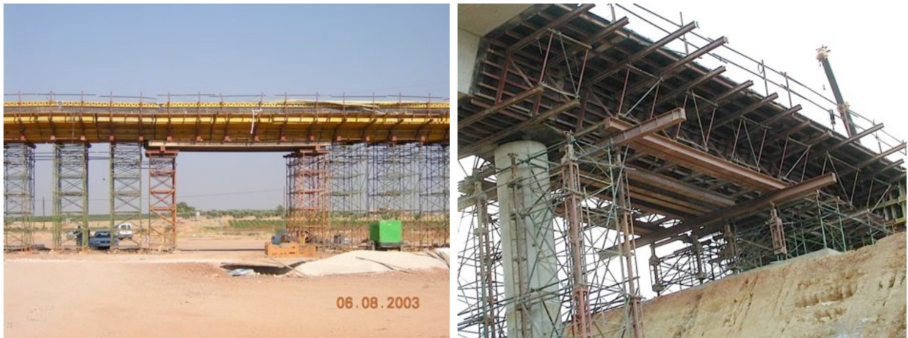
Fig. 7-5. Frames to cross roads and slopes. Courtesy of Ferrovial-Agroman.
