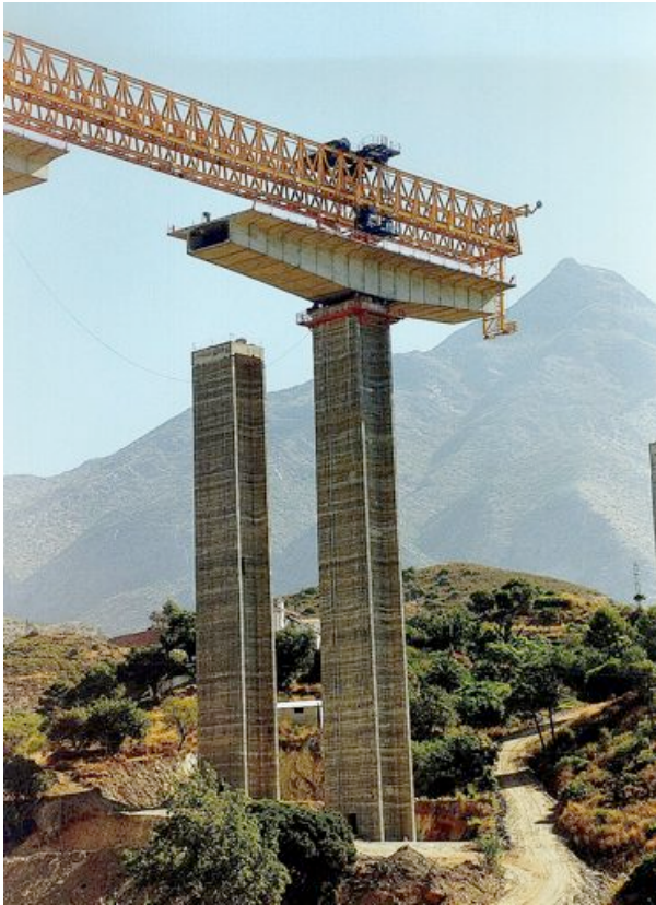
Fig. 7-45. Launcher for cantilever segments. Courtesy of Ferrovial-Agroman.
