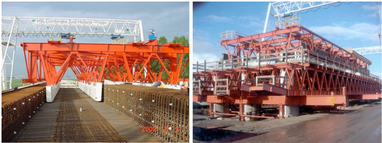
Fig. 7-22. Traveller for a Pi upside-down cross section. Courtesy of BAM Civil.
