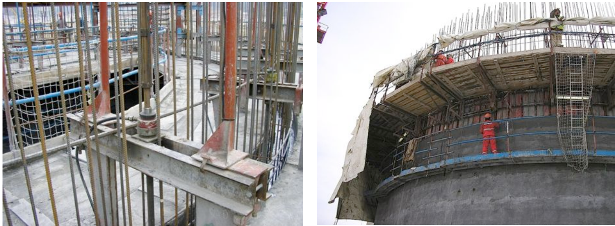
Fig. 6-9. Slip formwork in Tanger harbour. Courtesy of Bouygues Travaux Publics.
