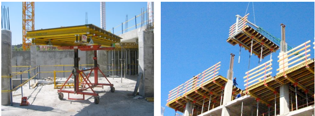
Fig. 7-44. Some proprietary system has safety facilities already implemented. Courtesy of PERI.
