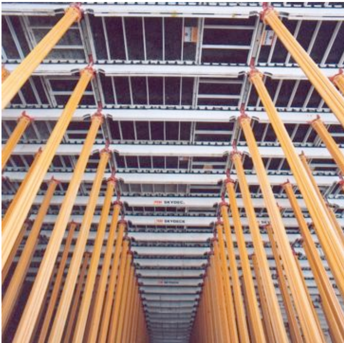
Fig. 7-40. Prop system. Courtesy of PERI.
