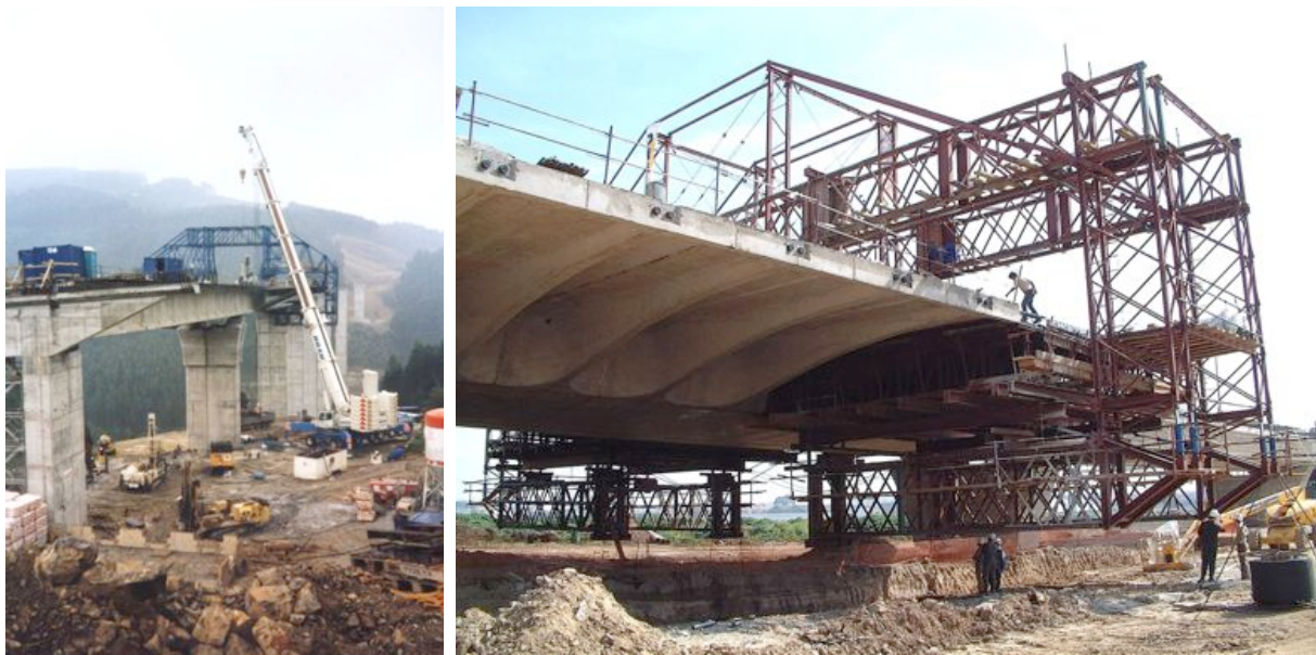
Fig. 7-12. These travellers allow simultaneous concrete slab and assembling of permanent props or ribs. Left: Courtesy of Alcor. Right: Courtesy of Mekanotubo.
