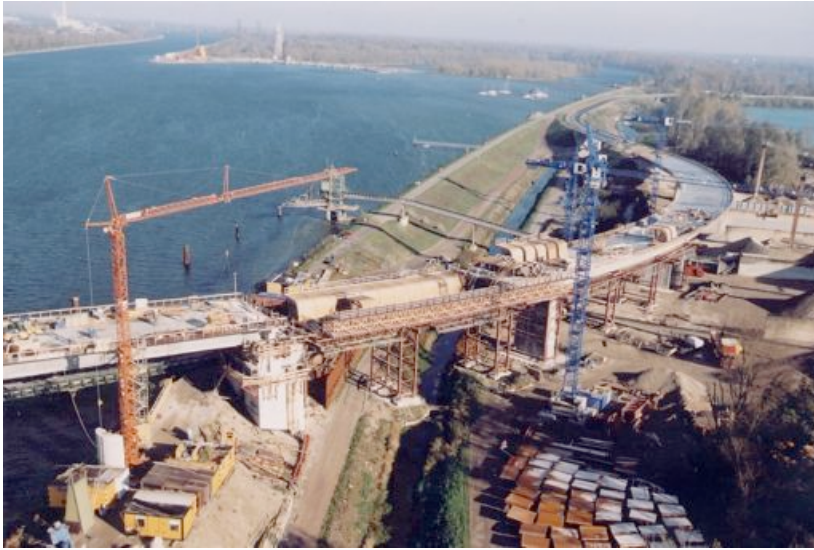
Fig. 7-51. Towers bearing a falsework. Courtesy of Setra/CTOA, Gerard Forquet.
