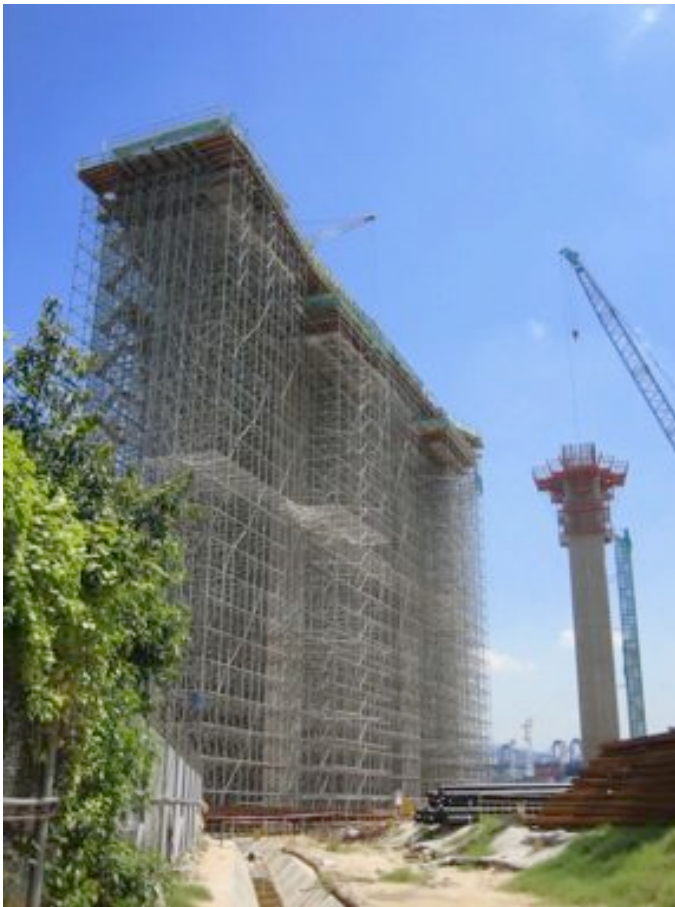
Fig. 7-2. High falsework for bridge shoring. Courtesy of Bouygues Travaux Publics.
