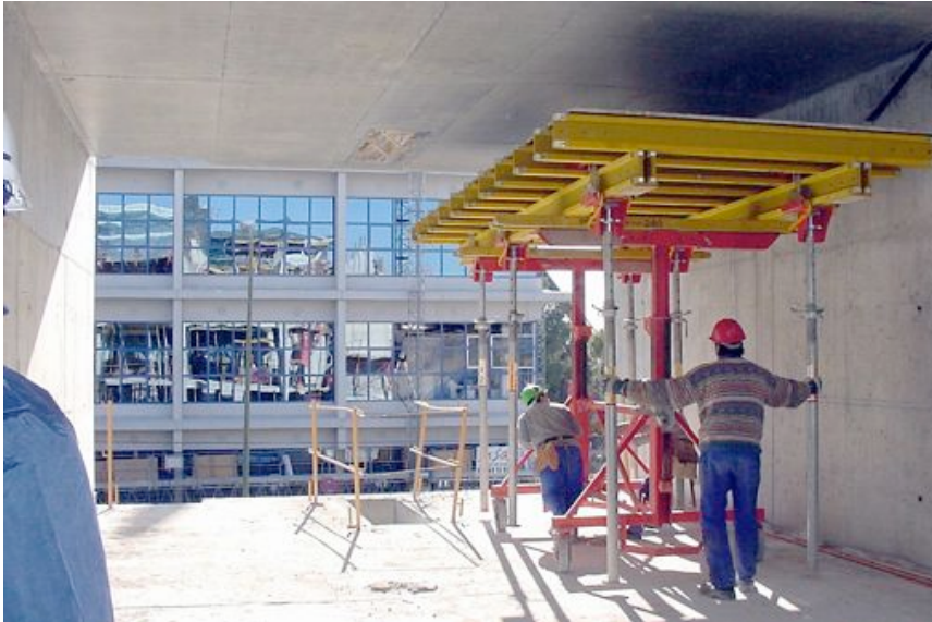
Fig. 7-41. Shoring floor system. Courtesy of PERI.
