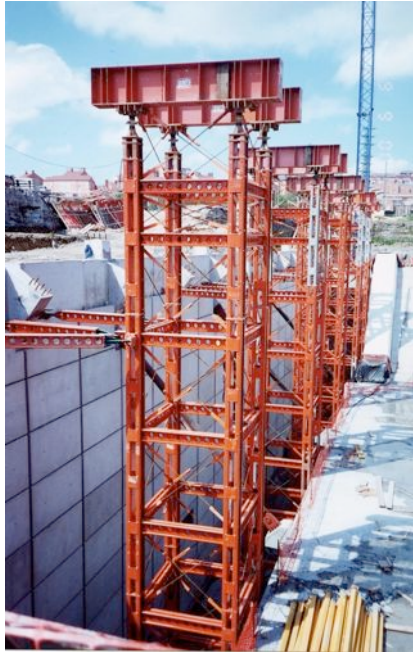
Fig. 7-57. Tower with stiffening elements attached to a wall. Courtesy of RMD.
