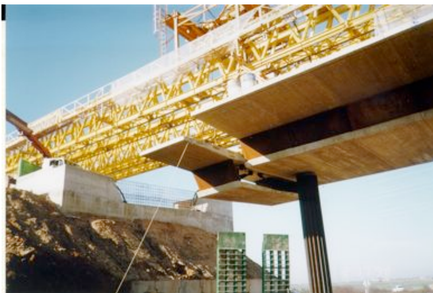
Fig. 7-20. Pre-cast segments hanging from the traveller. Courtesy of Ferrovial-Agroman.
