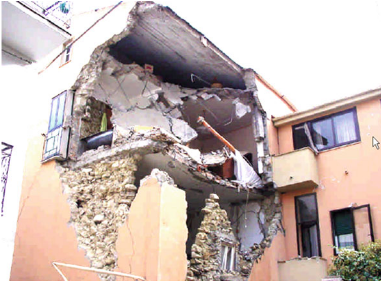
Fig. 11.38 Corner failure
