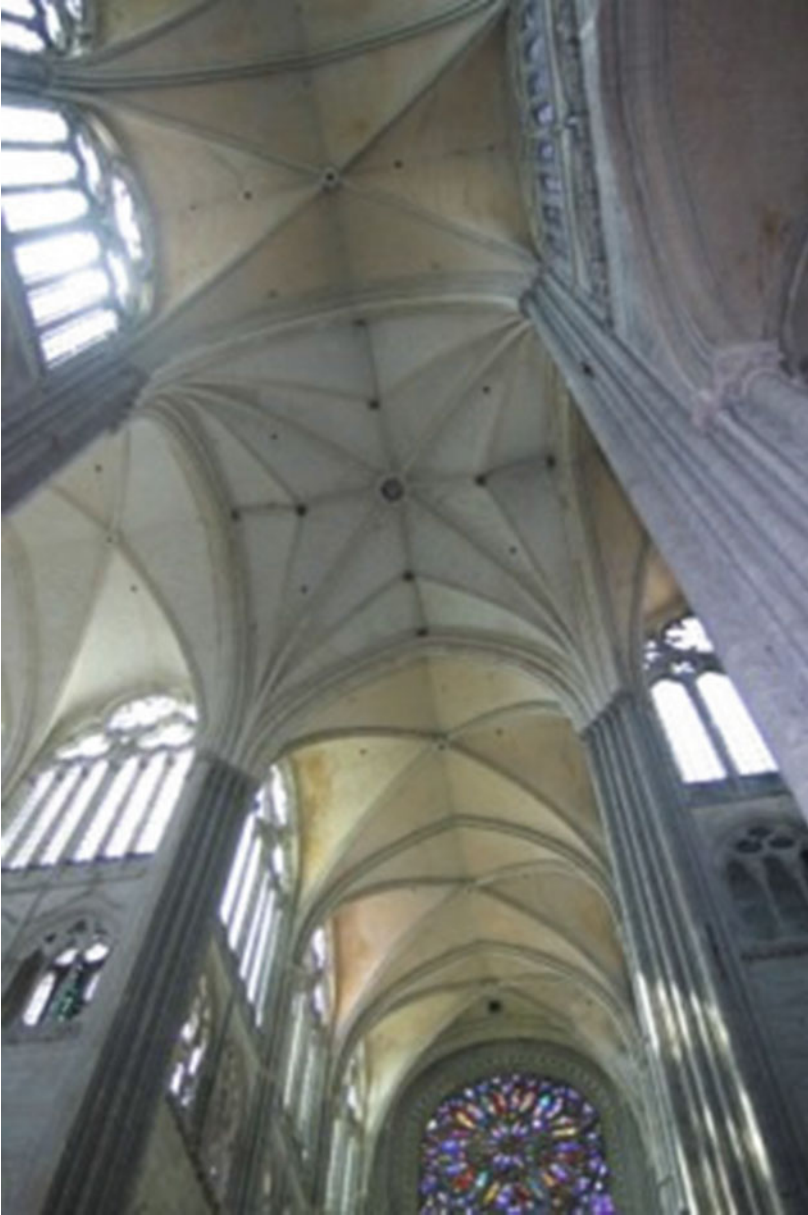
Fig. 6.1 Cross vaults of the cathedral of Amiens
