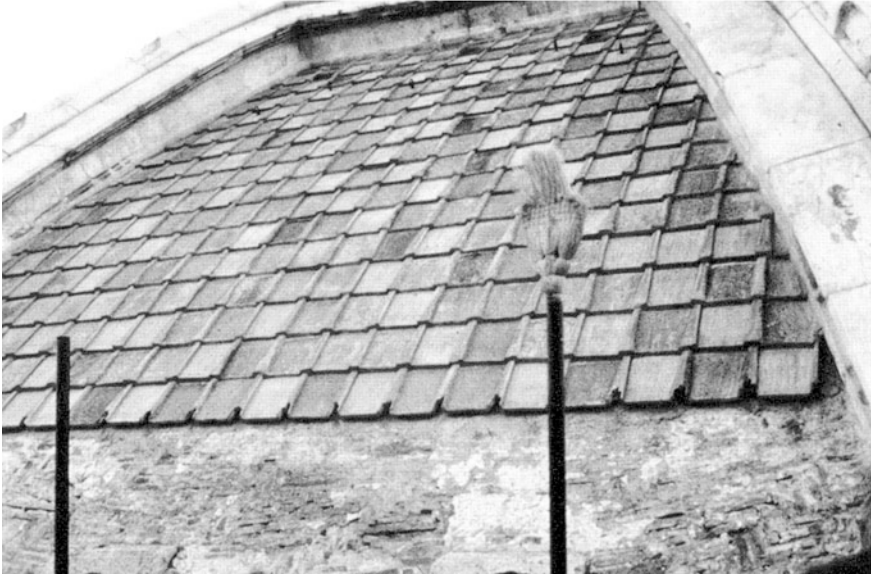
Fig. 4.59 Discovery of the conical brick beds beneath the horizontal rows of tiles (Di Pasquale 2002)
