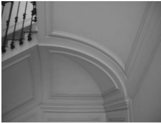
Fig. 8.2 Stair corner at the flight-to-landing intersection
