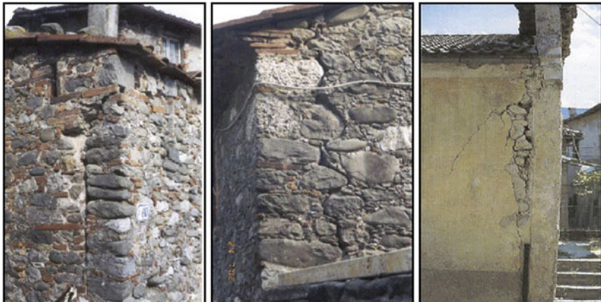
Fig. 11.35 Corners damagements
