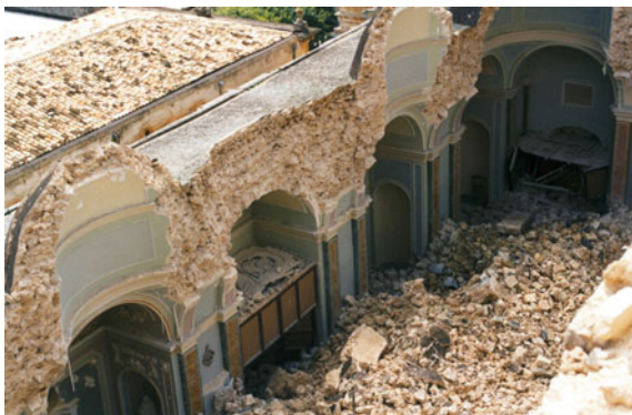
Fig. 2.84 The massively thick concrete of the arches and of the small domes over the right aisle
