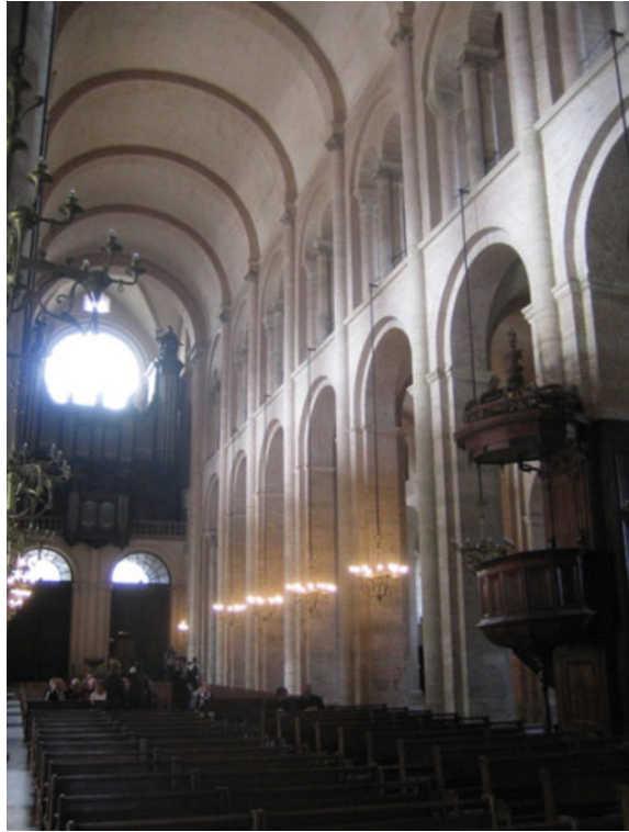
Fig. 5.1 Barrel vault of the Basilica of St. Sernin in Toulouse
