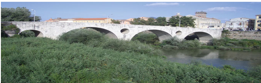
Fig. 3.21 An elliptical profile bridge on the River Calore in Benevento
