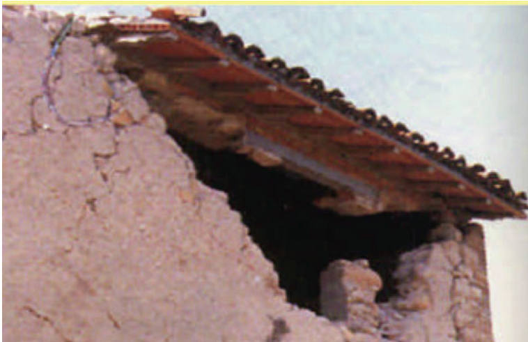
Fig. 11.39 Breaking of the tip of a facade wall
