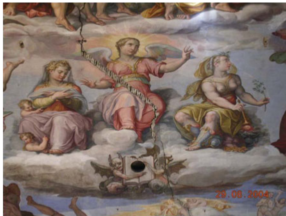
Fig. 4.64 Cracks running across the fresco of Zuccari (Ottoni 2012)
