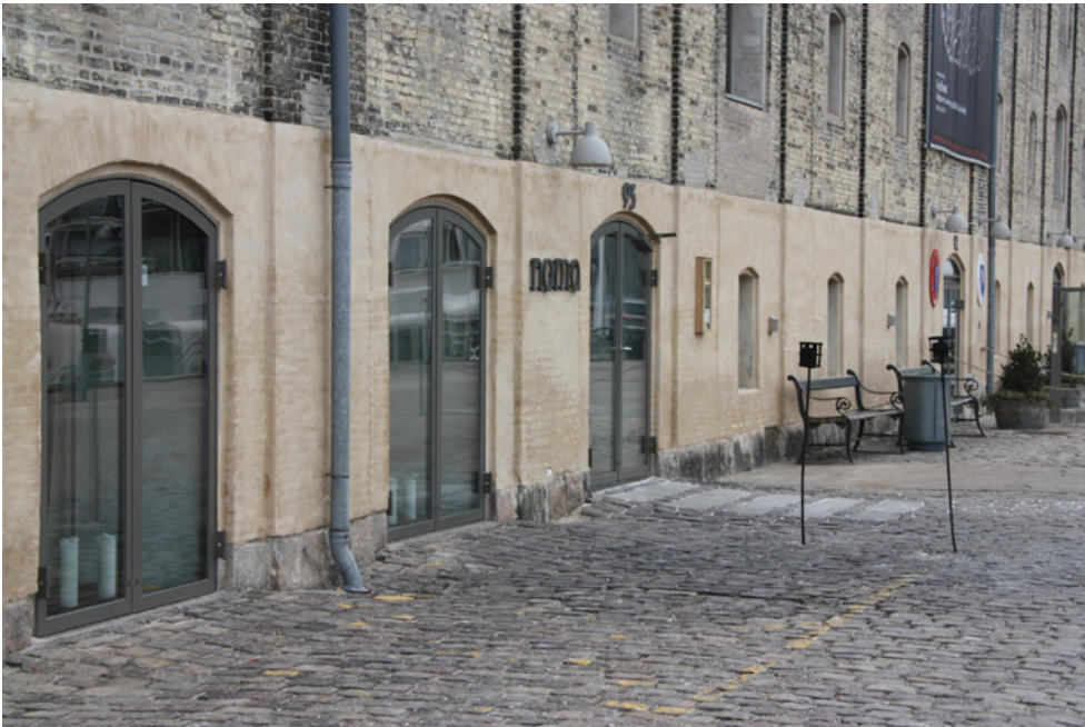
Figure 8.15 The North Atlantic House (detail), Copenhagen, Denmark. Photograph provided courtesy of Dr. Juriaan van Meel.
