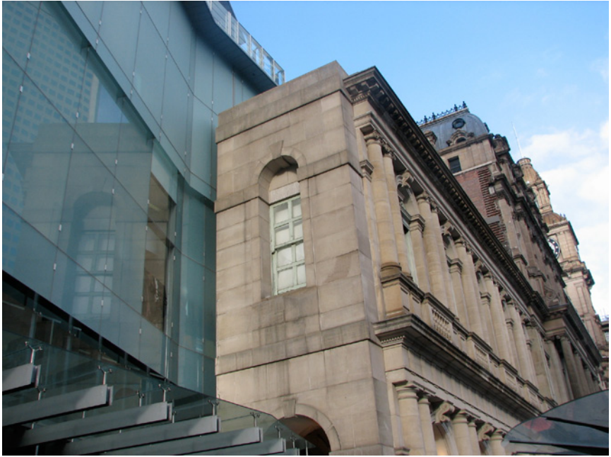
Figure 9.4 Melbourne GPO exterior (showing junction of new extension).
