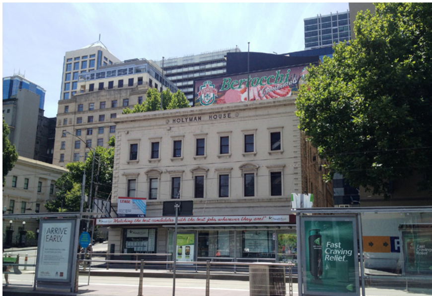
Figure 3.4 Holyman House, Melbourne.
