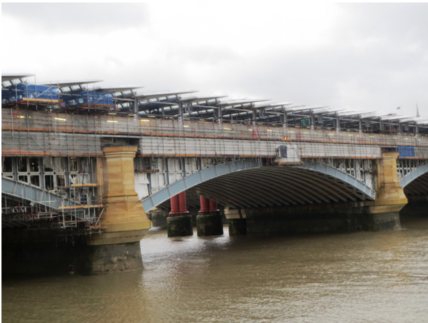
Figure 5.7 Blackfriars Bridge and Station, London, UK.
