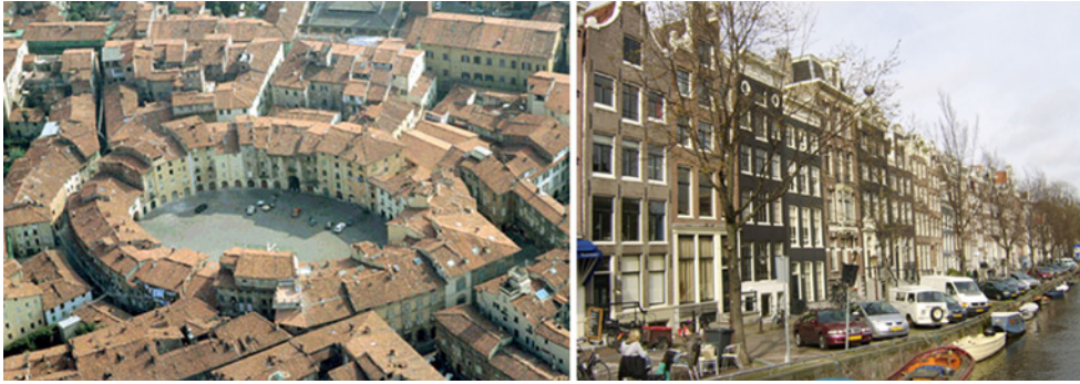
Figure 5.1 The former amphitheatre in Lucca and the canal houses in Amsterdam.
