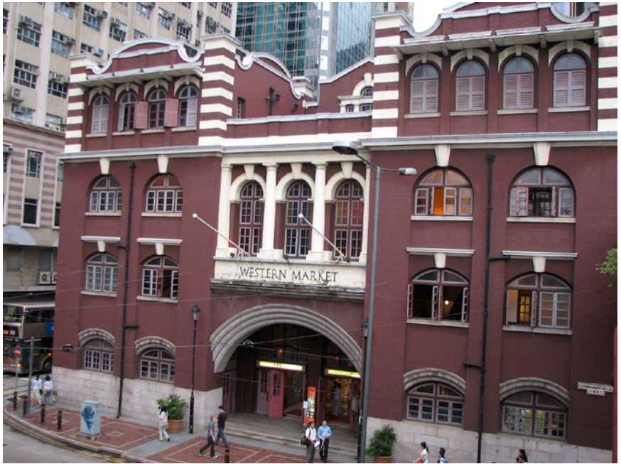
Figure 1.1 Western Market (1906–2003), Sheung Wan, Hong Kong.
