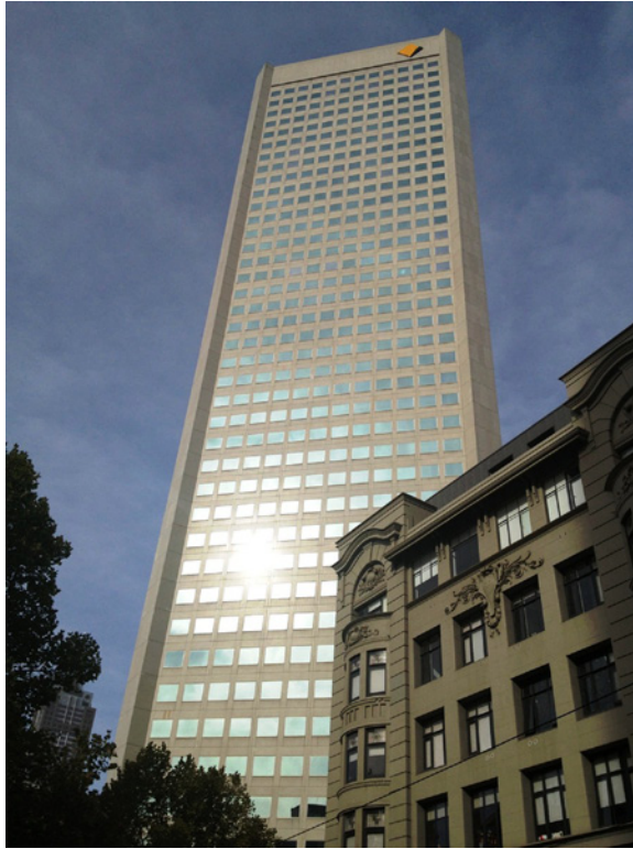
Figure 4.9 Front elevation, 385 Bourke Street.
