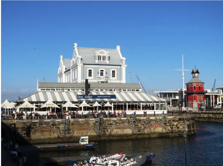
Figure 5.15 The African Trading Post Building, Waterfront, Cape Town, South Africa.
