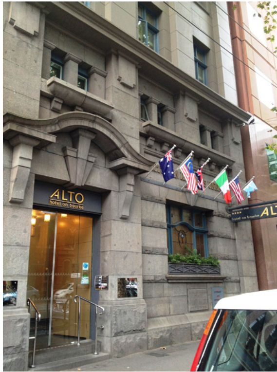
Figure 4.2 Front elevation, 636 Bourke Street.
