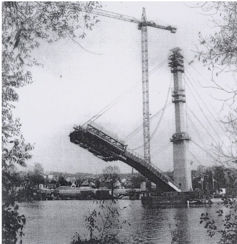
Fig. 8.3-3: Main bridge Veitshöchheim
