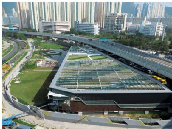
Figure E9.9.2 North Plant and Chiller Installation. © Arup
