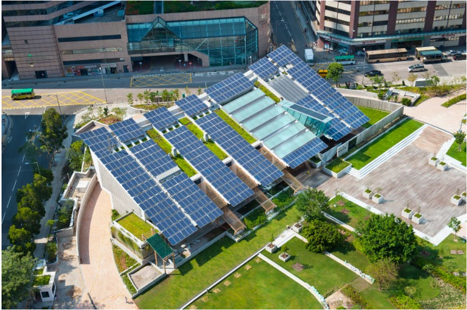
Figure E9.2.1 CIC ZCB in Hong Kong. © Arup
