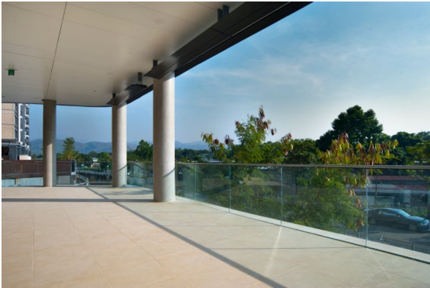
Figure E12.3.2 AIU Application at The Green Atrium, Hong Kong. © Arup
