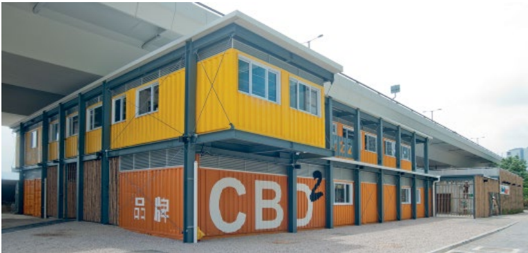
Figure E7.5.1 Energising Kowloon East Office, Hong Kong. © Arup
