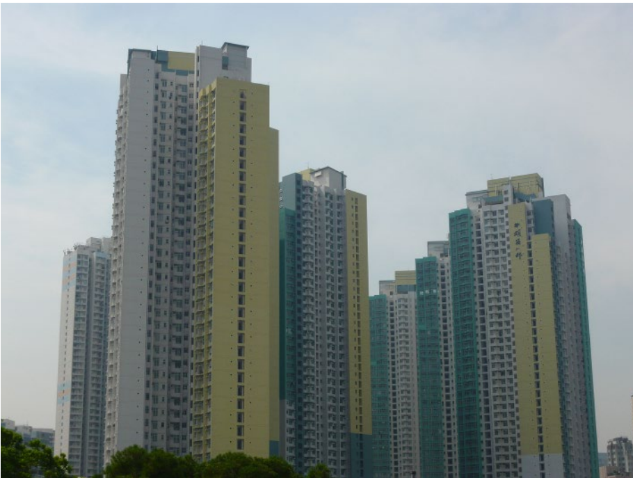
Figure E11.1.1 Upper Ngau Tau Kok Estate Redevelopment, Hong Kong. © Arup
