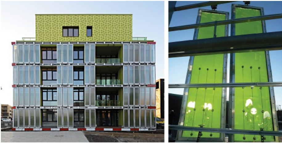
Figure E8.5.1 BIQ House in Germany. © Colt/Arup/SCC
