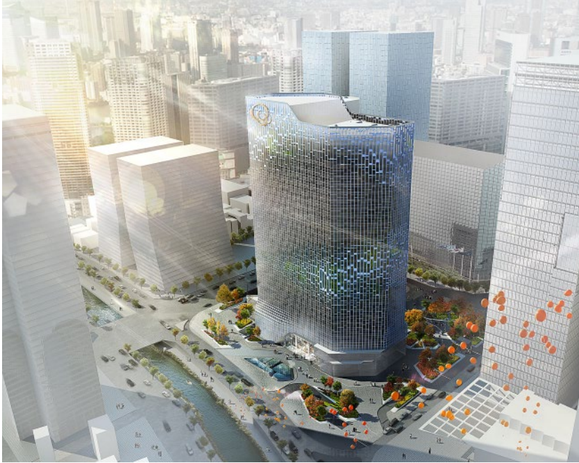
Figure E9.4.1 Hanwha Headquarters in Seoul, South Korea. © UNStudio
