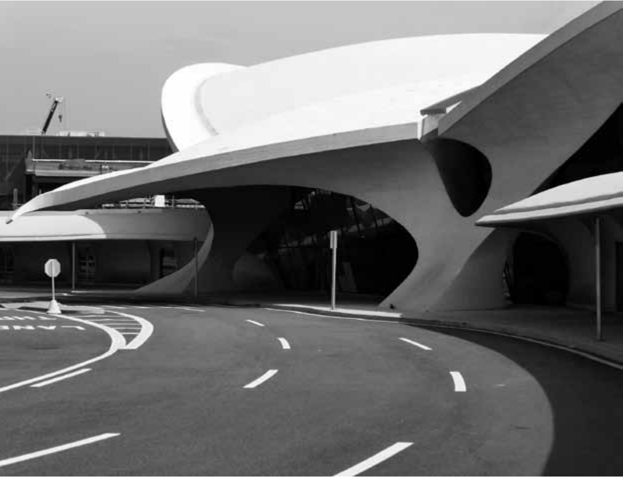
71. Arriving at TWA Terminal 5, JFK Airport, NYC, Eero Saarinen, opened in 1962. © Bill Caplan
