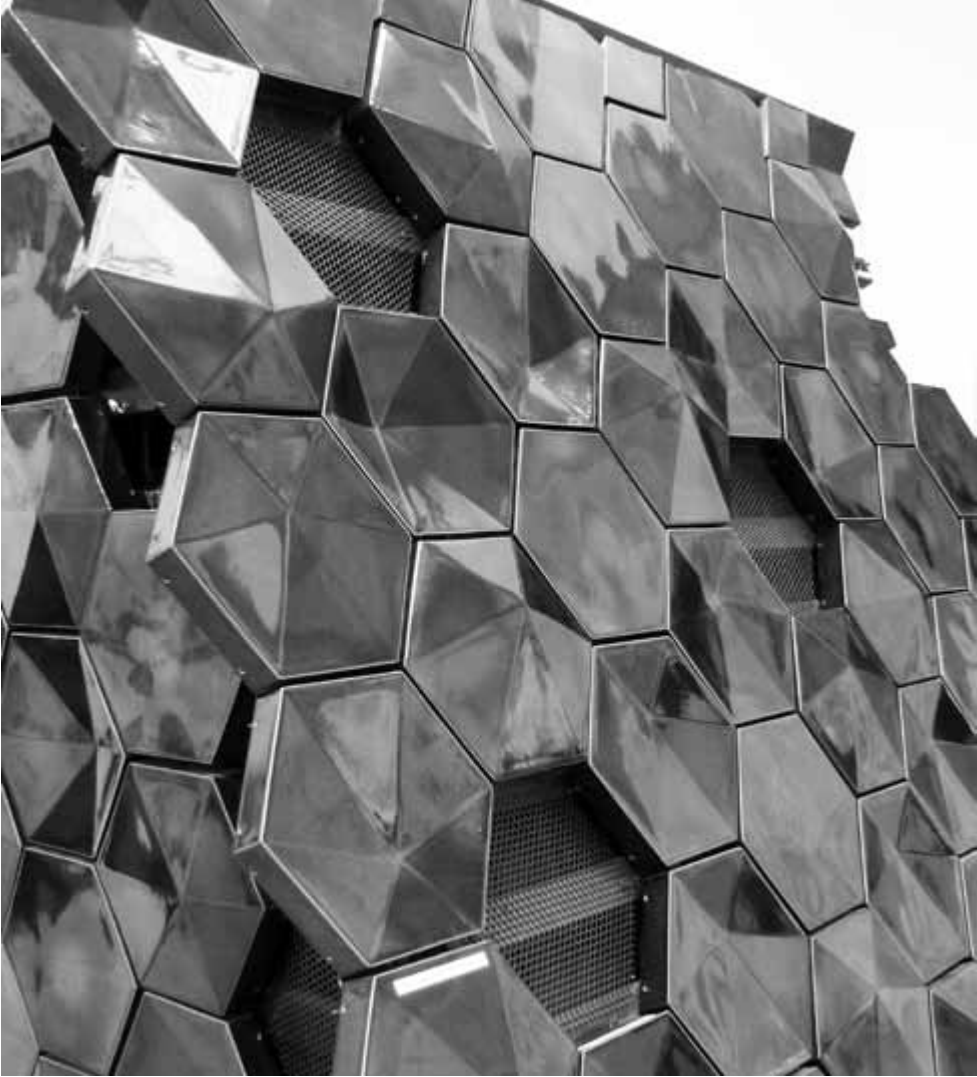
19. Rain barrier tiles and ventilating sectors; a physical, operative and sensible surface composite. Agrob Buchtal GmbH, designed by Herzog and de Meuron. 2014 Architecture Biennale, Venice. © Bill Caplan
