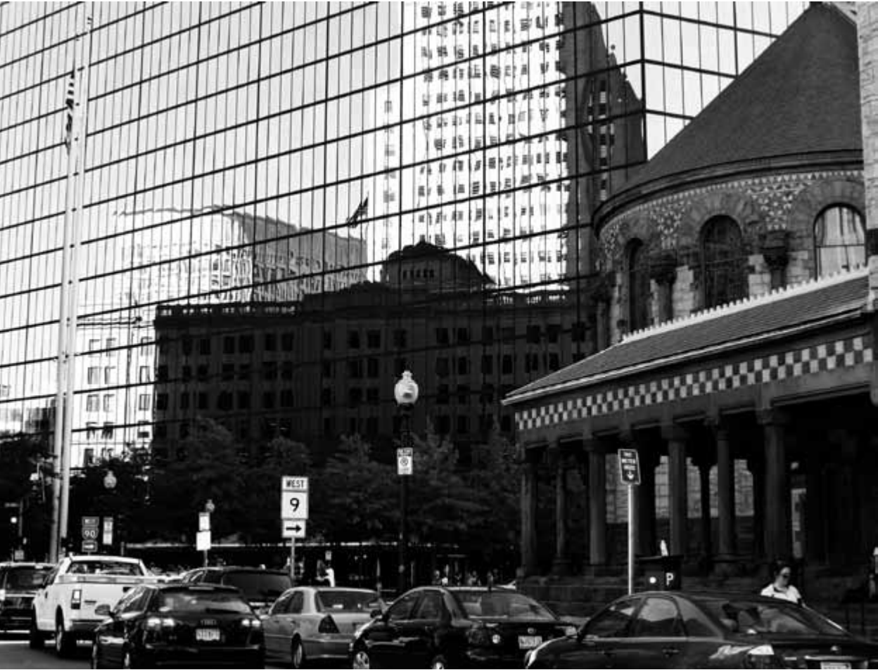
13. The Hancock Tower from Clarendon Street (above); the Stuart Street facade (right). © Bill Caplan
