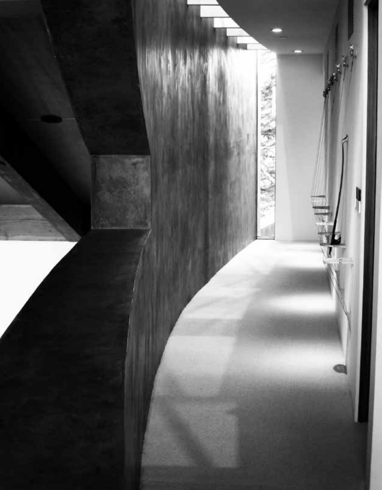
113. Curved hallway wall surfaced with trowelled black cement; the southwest window. © Bill Caplan
