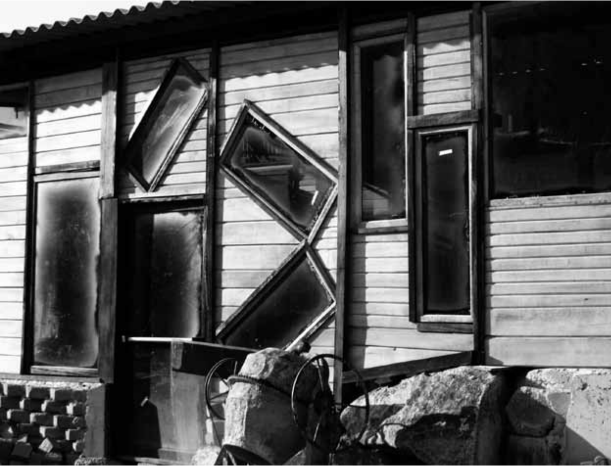
9. An envelope's barriers and ports. House in Florianopolis, Brazil. © Bill Caplan
