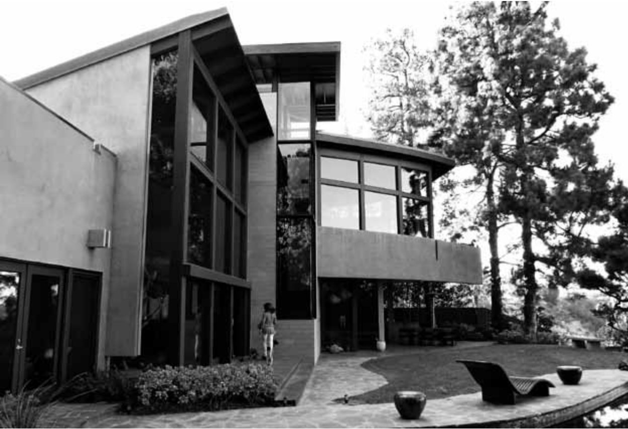
105. Eastern facade of the Stradella Road residence by David Hertz. Thermal chimney in centre. © Bill Caplan 120
