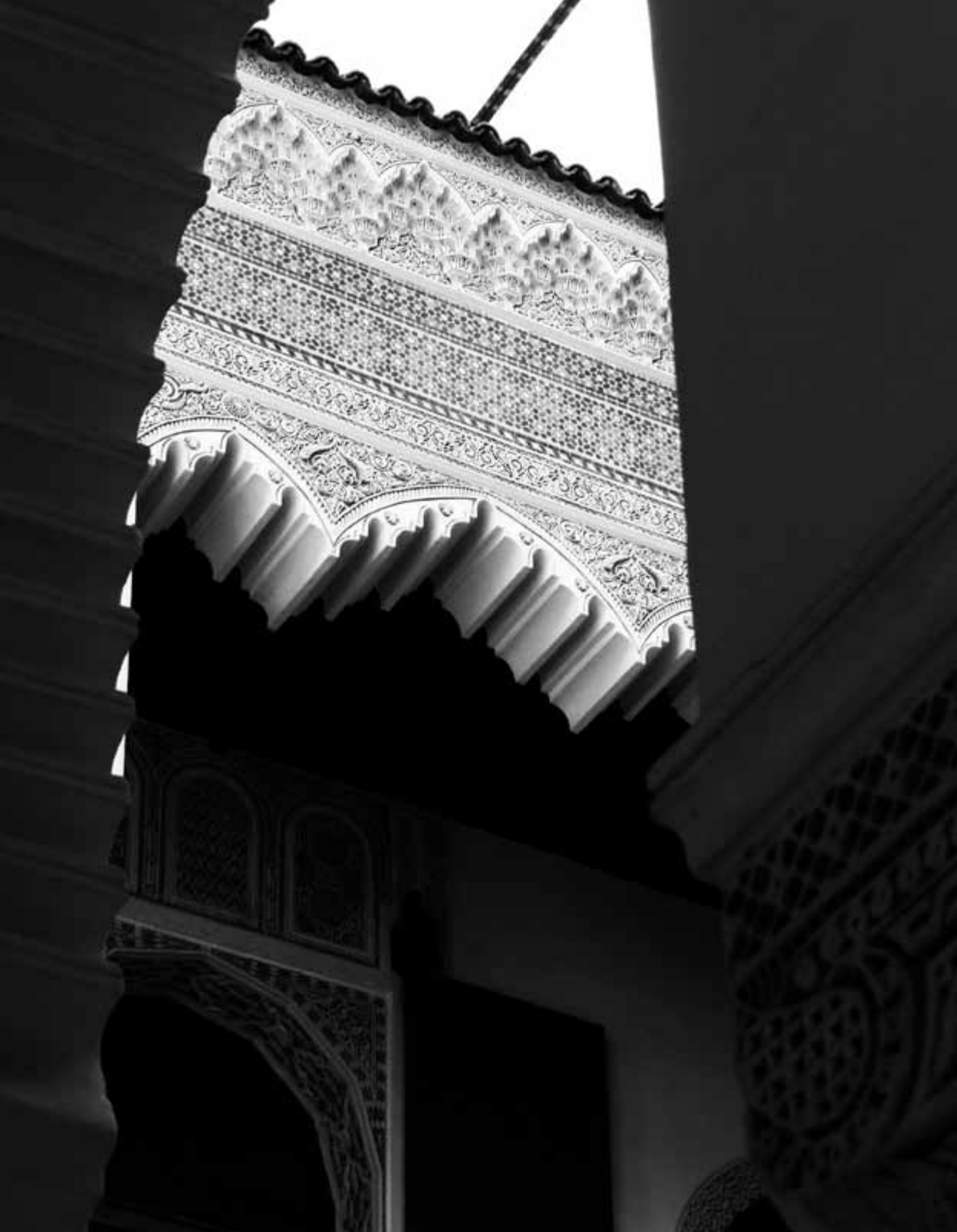
90. Carved stucco ornamentation with adjacent tile, riad in Fez, Morocco. © Bill Caplan
