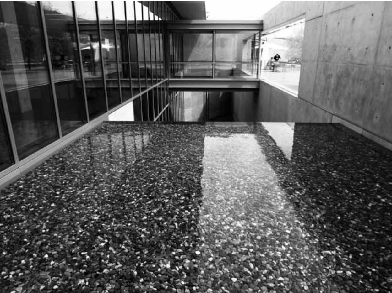
117. The Clark Center ground-level hydrology system water feature; excavated light well in rear. © Bill Caplan
