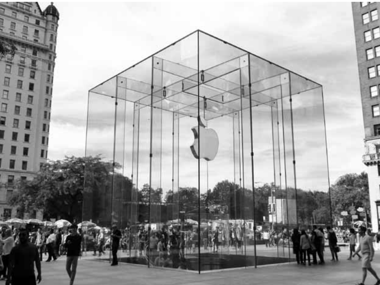
22. Glass walls, roof, structure: Apple Store by Bohlin Jackson, Fifth Avenue, New York City. © Bill Caplan
