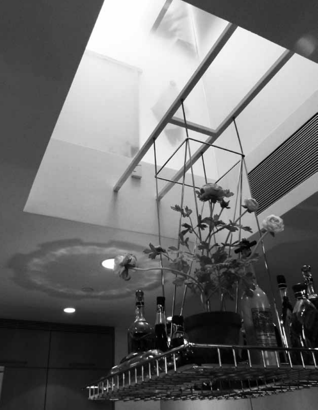
109. Kitchen: light shaft, exhaust and heat chimney, Stradella Road residence. © Bill Caplan
