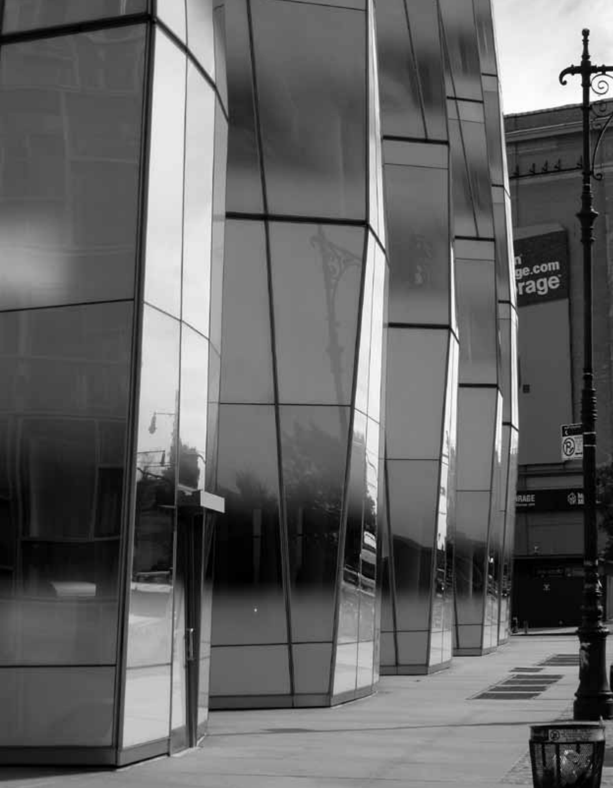
17. The IAC Building street interface on the West Side Highway. © Bill Caplan
