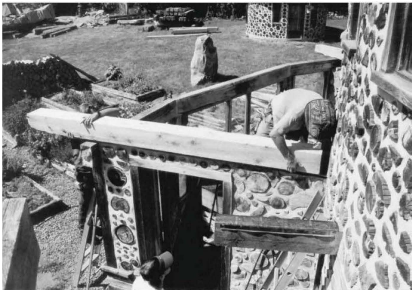
Fig. 5.8: We install the east side girt.
