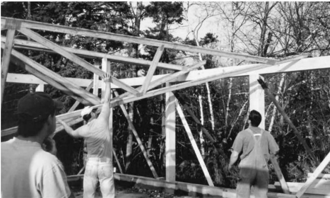
Fig. 4.46: The trusses are temporarily stored upside down, straddling the sidewalls.
