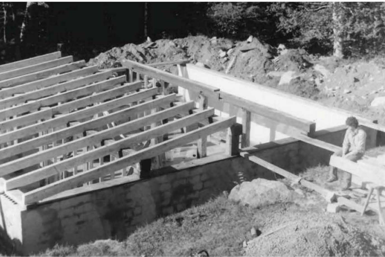
Fig. 4.40: Here, all of the east side four-by-eight rafters at Log End Cave are in place, with their western (right) ends supported over 30-foot-long ten-by-ten central girder or ridge beam. This ridge beam is well-supported along its length by a total of four posts, one at each end, and two others along the way to shorten the spans.
