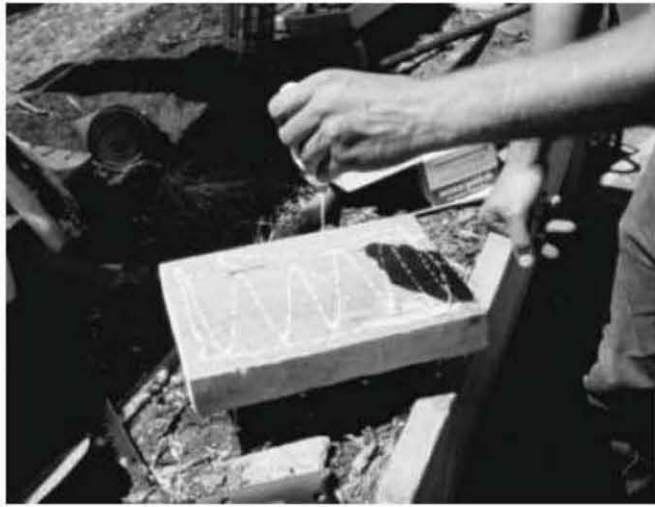
Fig. 5.9: Glue is applied to the gusset.
