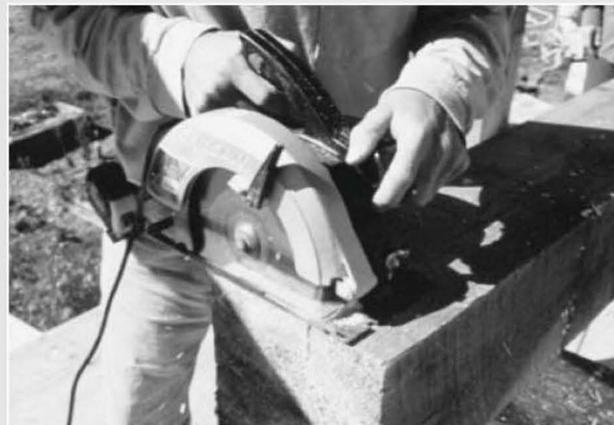
Fig. 5.28: Circular saw and handsaw.
