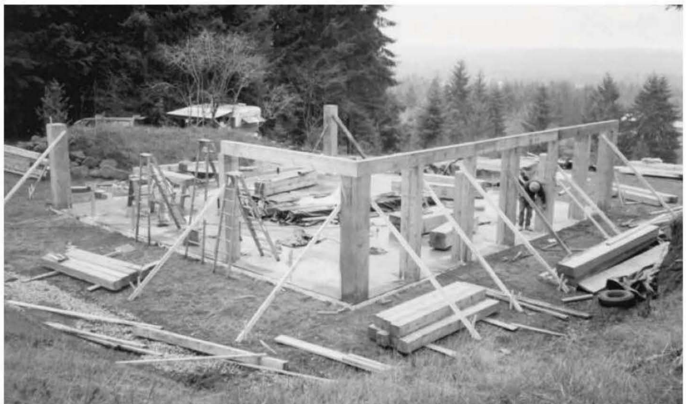
Fig. 4.54: Joe's sidewall posts are made of two eight-by-eights, strapped together with Simpson ties. The entire post is anchored to the concrete foundation with a Simpson HPAHD "hold-down." A code-required damp-proof course is installed between the post and the concrete. Joe Zinni photo.
