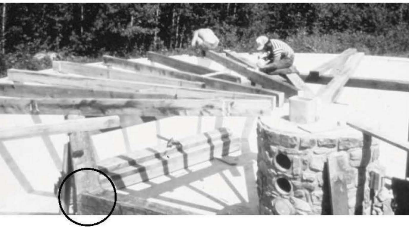
Fig. 4.23, above: Truss plates tie the girders together at the octagonal internal frame at Earthwood. This frame cuts the radial floor joist spans in half.
