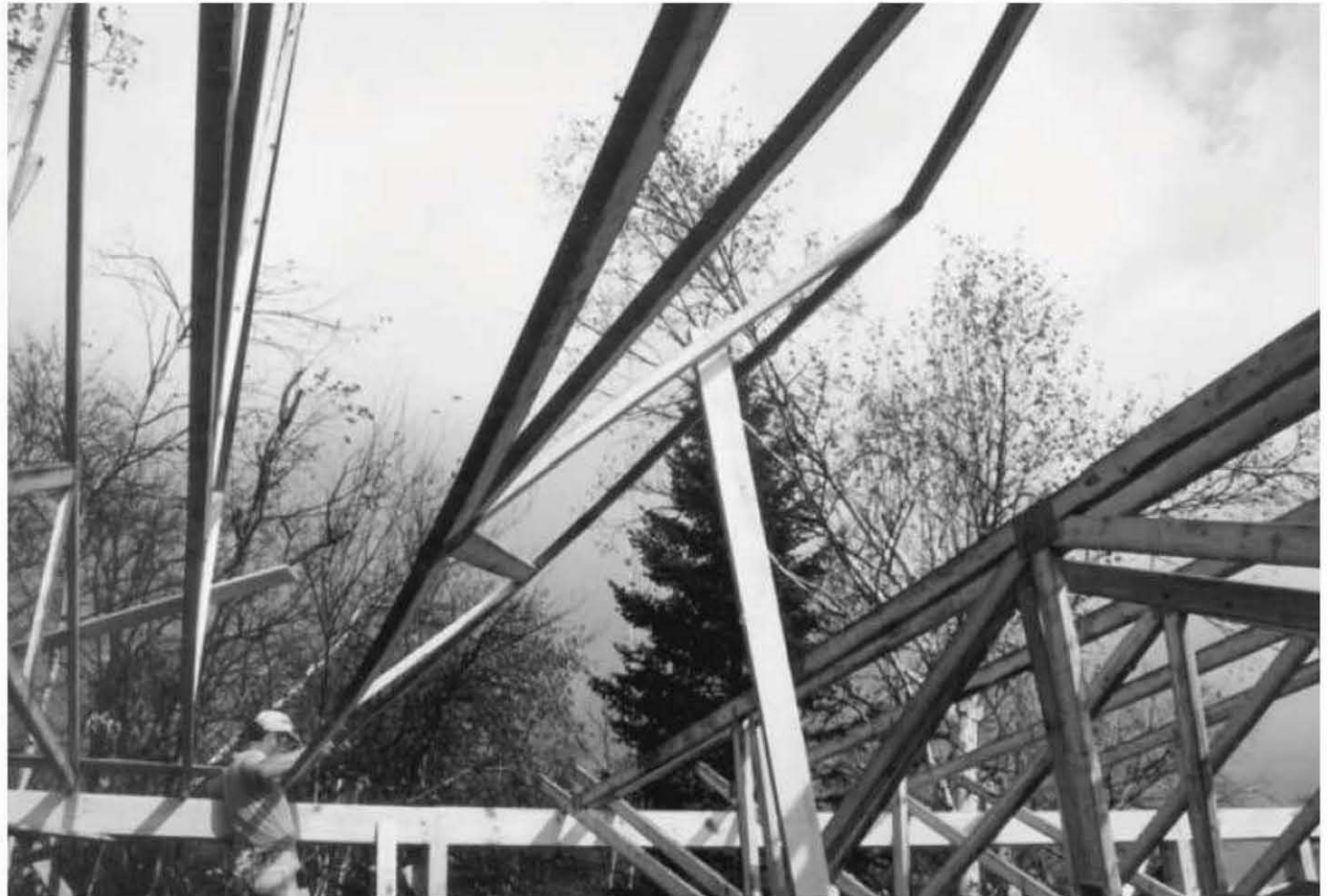
Fig. 4.49: The third truss is raised.
