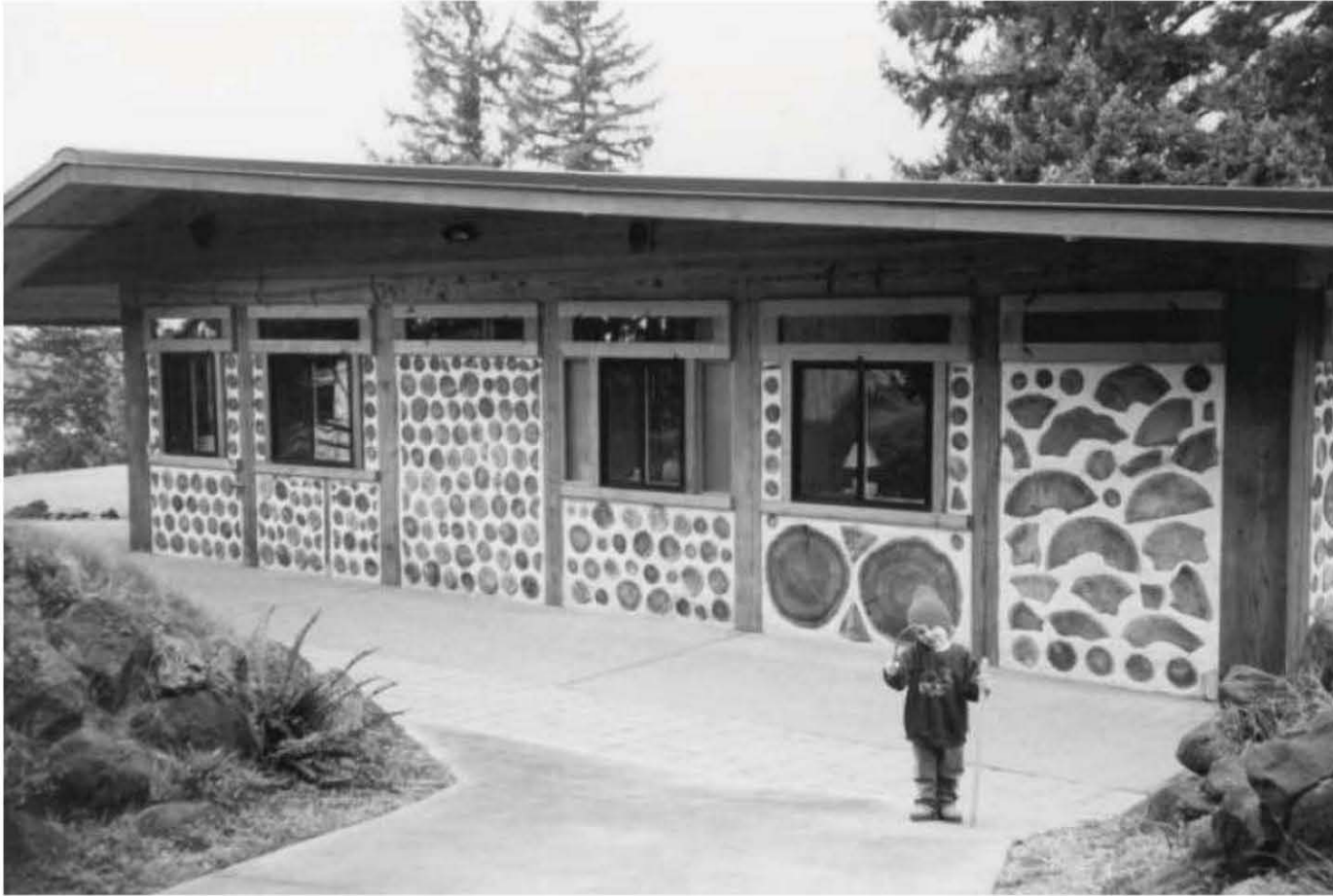
Fig. 4.62: The Zinni's completed home, with cordwood infilling. The trusses have two different pitches on their top chords. Young Sage Zinni looks like a leprechaun next to this massive structure. Joe Zinni photo.
