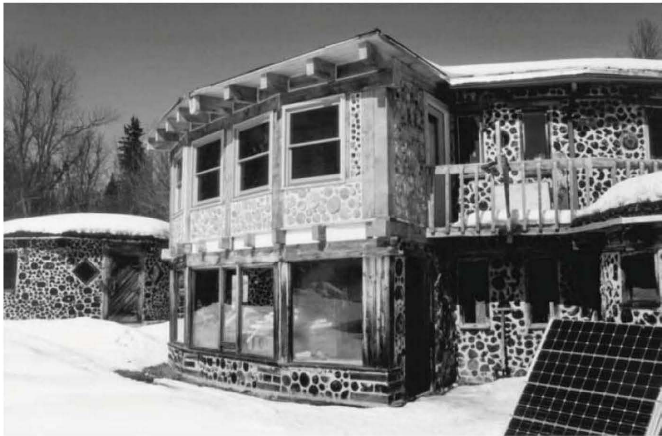
Fig. 5.41a & b (detail, below): The completed sunroom at Earthwood. Only the cordwood snow-blocking in the lower solar room remains to be done. We also waited until the spring of 2003 to put the earth on the roof.
