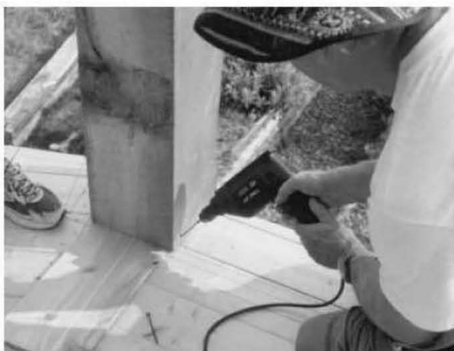
Fig. 5.30: The author toe-screws the base of the post to the floor.
