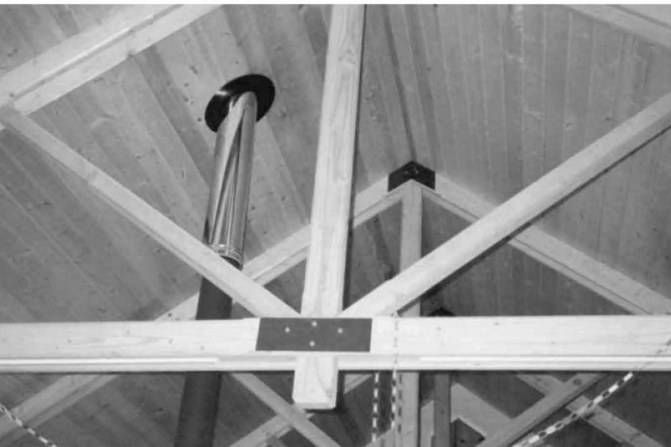
Fig. 4.52: Strong trusses, built on site, support a plank roof.
