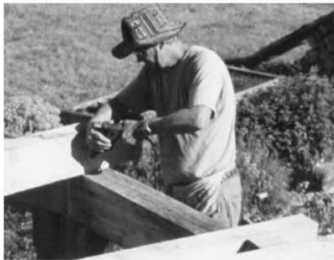
Fig. 5.12: The author toe-screws the four-by-eight joist to the six-by-ten girder.
