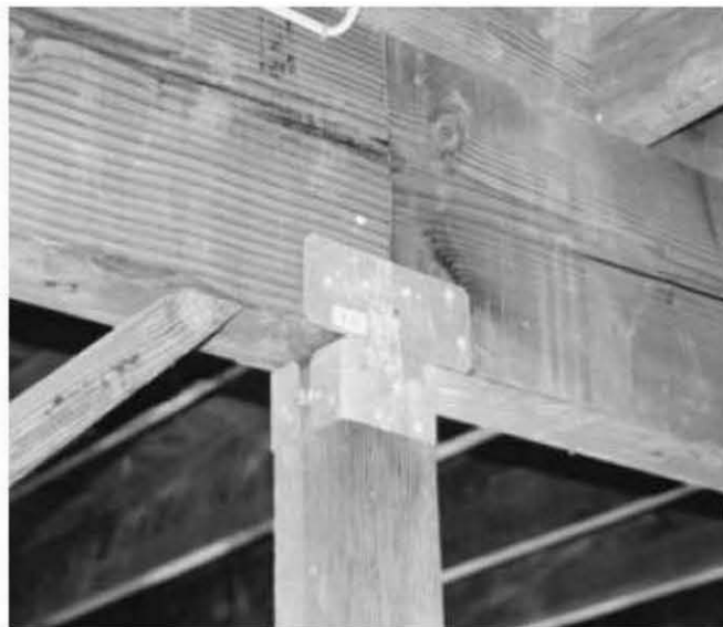
Fig. 4.23, above: Truss plates tie the girders together at the octagonal internal frame at Earthwood. This frame cuts the radial floor joist spans in half.
