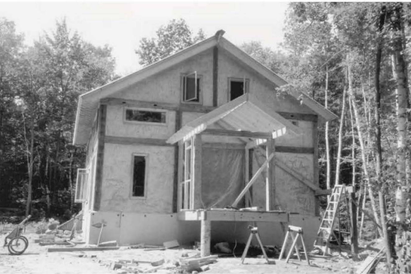
Fig. 1.2: Ki Light built a straw bale house near West Chazy, New York using a simple timber frame whose members are joined by the non-traditional means described in this book.
