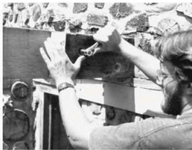
Fig. 5.11: Doug tightens a hex nut up to a washer on the threaded end of one of the bolts. As Doug looks at the stub, he is installing a bolt at the upper left and lower right of the stub, keeping about three inches from all edges. The carriage end of the bolt is on the other side of the unit, and is drawn into the new four-by-eight by tightening the nut. We countersunk the nuts and washers, so that we could use 8-inch bolts without the threaded end protruding from the joist.
