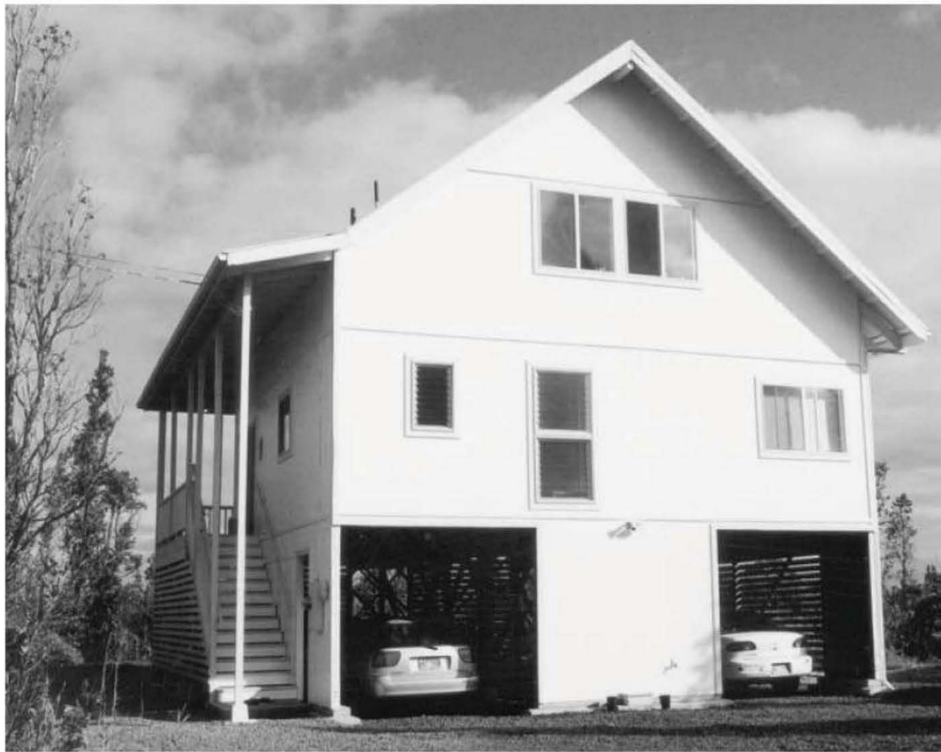
Fig. 4.18: Steve and Eileen Sugar's home in Hawaii makes use of a post-and-beam frame and mechanical fasteners.
