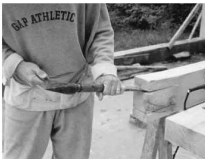
Fig. 4.30: The two longer cuts meet, but not quite all the way, because of the circular shape of the saw blade. However, the wood is easily snapped off with a chisel.
