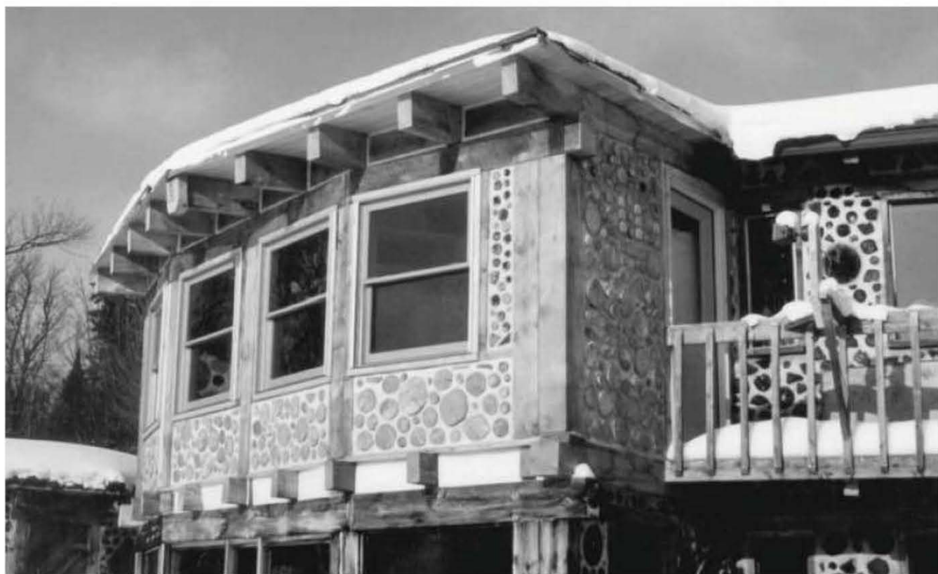
Fig. 5.41a & b (detail, below): The completed sunroom at Earthwood. Only the cordwood snow-blocking in the lower solar room remains to be done. We also waited until the spring of 2003 to put the earth on the roof.
