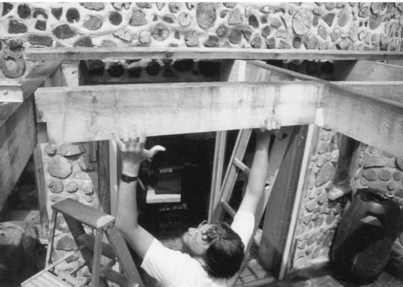
Fig. 5.18, below: Doug places the header onto its supports.
