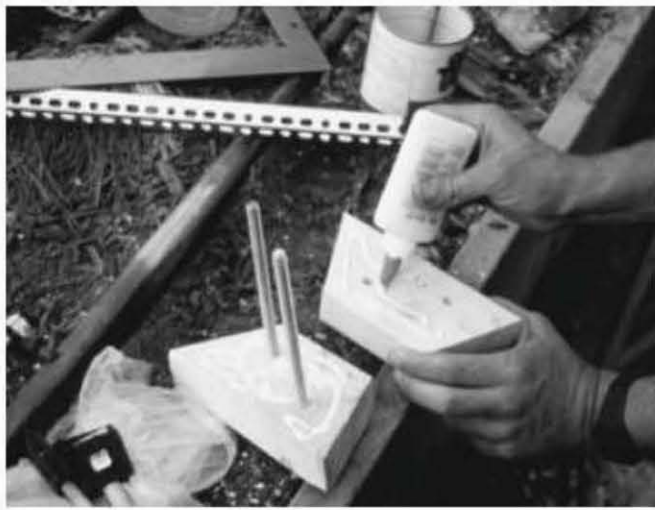
Fig. 5.16, near right: The supports are glued and the carriage bolts installed.
