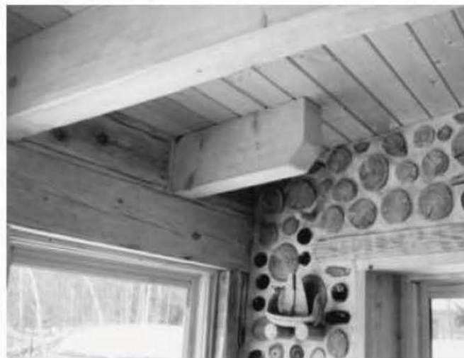
Fig. 5.44, near right: Ceiling and rafter detail.
