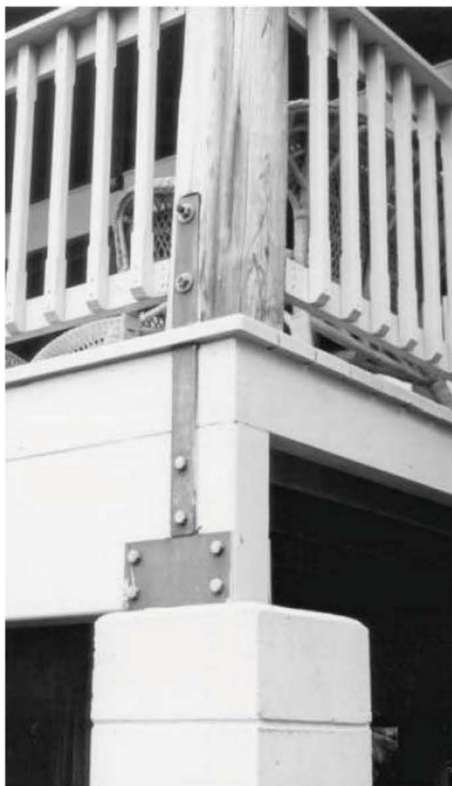
Fig. 4.18: Steve and Eileen Sugar's home in Hawaii makes use of a post-and-beam frame and mechanical fasteners.
