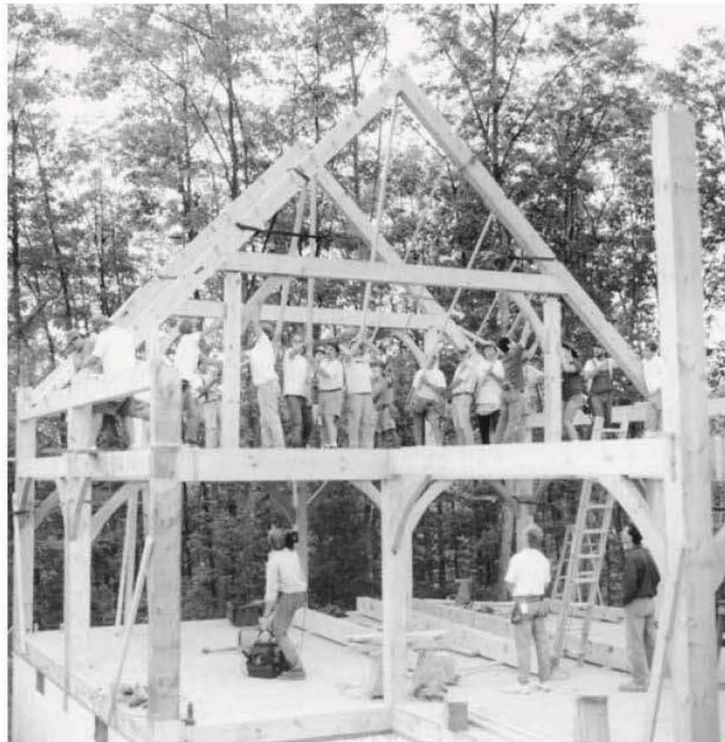
Fig. 2.17: Students at Fox Maple School of Traditional Building in Brownfield, Maine, erect a timber frame at a workshop. Photo provided by Fox Maple Director Steve Chappell.
