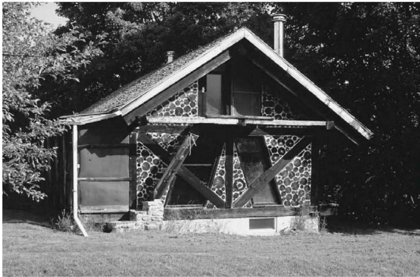
Fig. 1.1: In 1975, the author, with his wife, Jaki, built Log End Cottage, West Chazy, New York, using simple timber framing strategies “for the rest of us.” Panels between posts are infilled with cordwood masonry.
