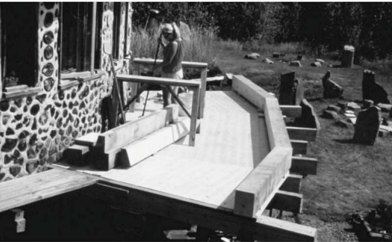
Fig. 5.23: The girders are mocked up on the deck.
