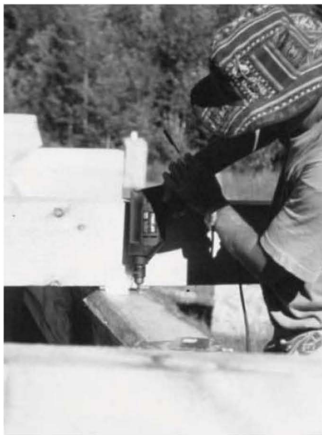
Fig. 5.13: A right angle fastener can take the place of toenails or toe-screws.
