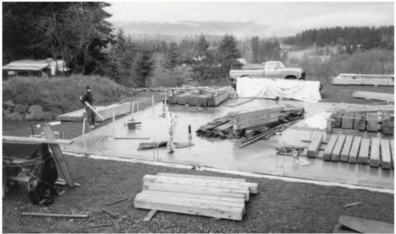
Fig. 4.54: Joe's sidewall posts are made of two eight-by-eights, strapped together with Simpson ties. The entire post is anchored to the concrete foundation with a Simpson HPAHD "hold-down." A code-required damp-proof course is installed between the post and the concrete. Joe Zinni photo.
