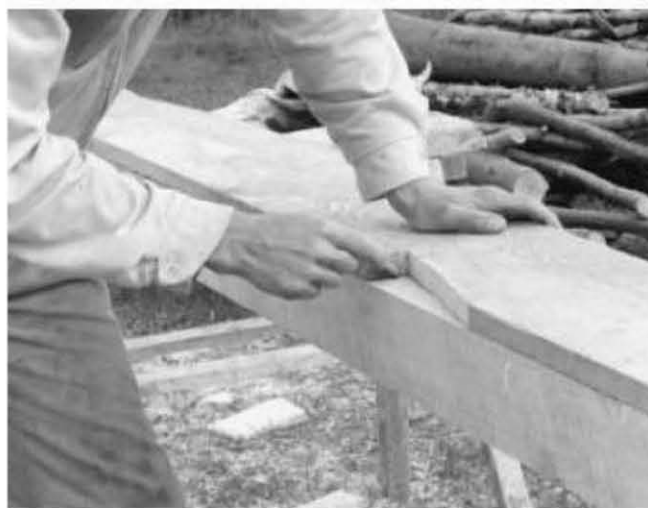
Fig. 4.42: I mark the birdsmouth on a four-by-eight rafter by using a template made from a one-by-eight board.
