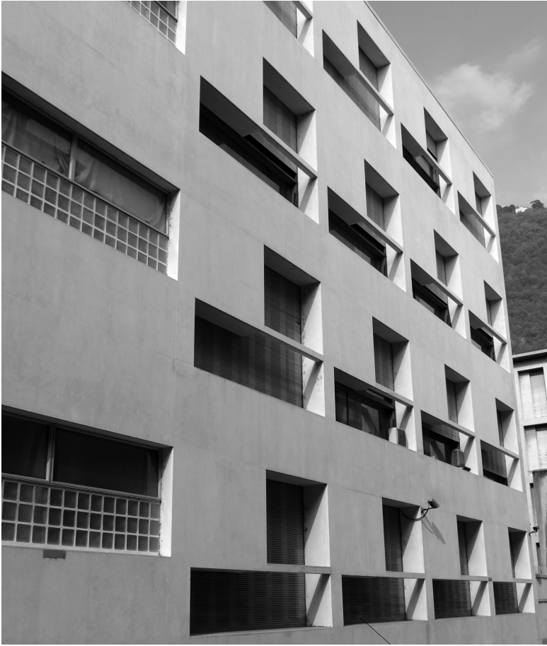
19.02 Beauty for buildings should be more than skin deep. Casa del Fascio, Giuseppe Terragni, 1931–1933
