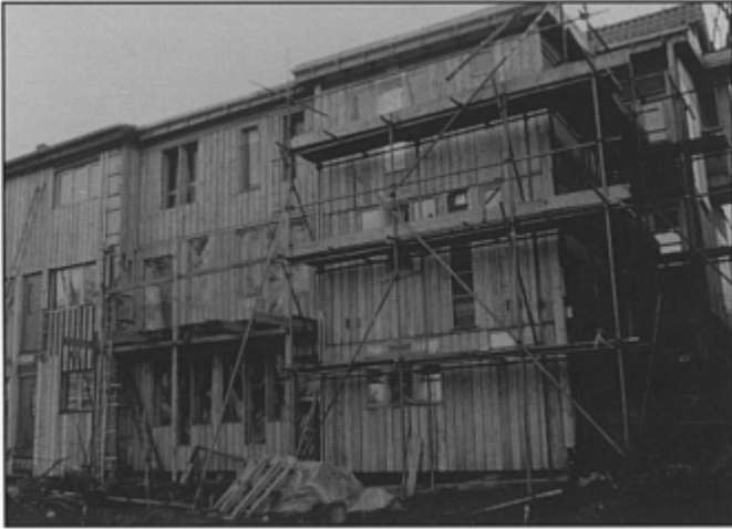
Plate 7. Housing at Chapel Allerton (Rear elevation)
