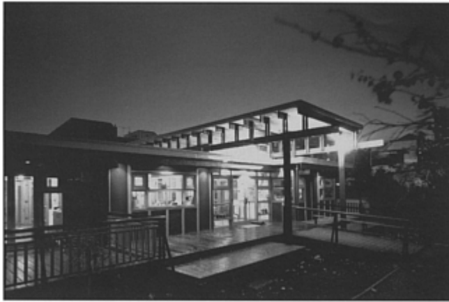
Plate 3. Calthorpe Community Centre Timber Frame Building, Kings Cross London
