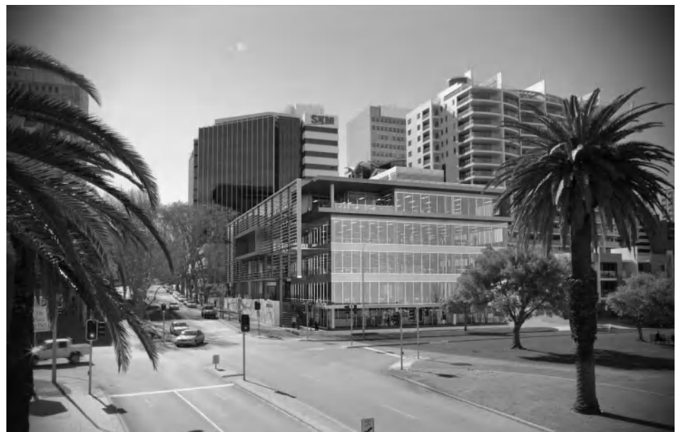
Figure 12-2 Two Victoria Avenue in Perth, Australia, achieved the highest Green Star certification of six stars. This 77,500-square-foot office building was designed by Woodhead for Stockland. Sustainable features include operating louvers to reduce heat loads, an active chilled beam system, roof-integrated wind turbines, on-site graywater treatment, and high-performance glazing. Image courtesy of Stockland.
