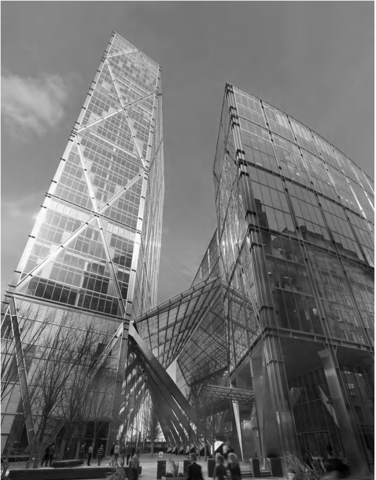
Figure 12-1 These London office towers, designed by Skidmore, Owings & Merrill for British Land, achieved the highest BREEAM rating of Excellent. Combined, the 13-story 201 Bishopsgate and the 35-story Broadgate Tower provide 800,000 square feet of office space and ground-floor bars, cafes, and shopping. At its completion in 2008, 201 Bishopsgate and The Broadgate Tower was the largest speculative office development undertaken in the City of London.
