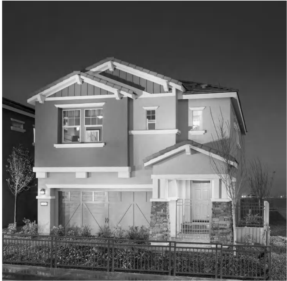
Figure 4-5 The Venezia model is one of four models offered in the Villa Trieste community. All homes have roof-integrated solar systems. Centralized battery storage is provided at the substation level to store excess energy for use when needed. Photo © 2009, Pulte Homes and the Communities of Del Webb.
