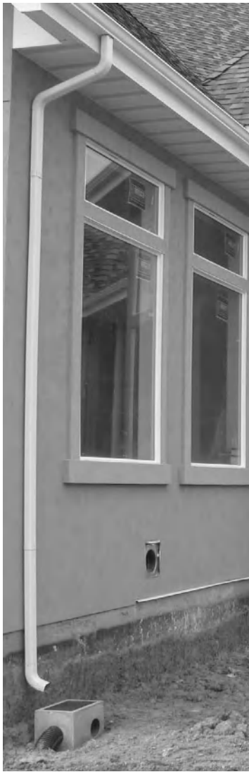
▲ Figure 6-7 To enhance durability and reduce maintenance, the NGBS rewards roof water discharge systems that carry water a minimum of five feet from foundation walls. Photo courtesy of Magleby Companies.
