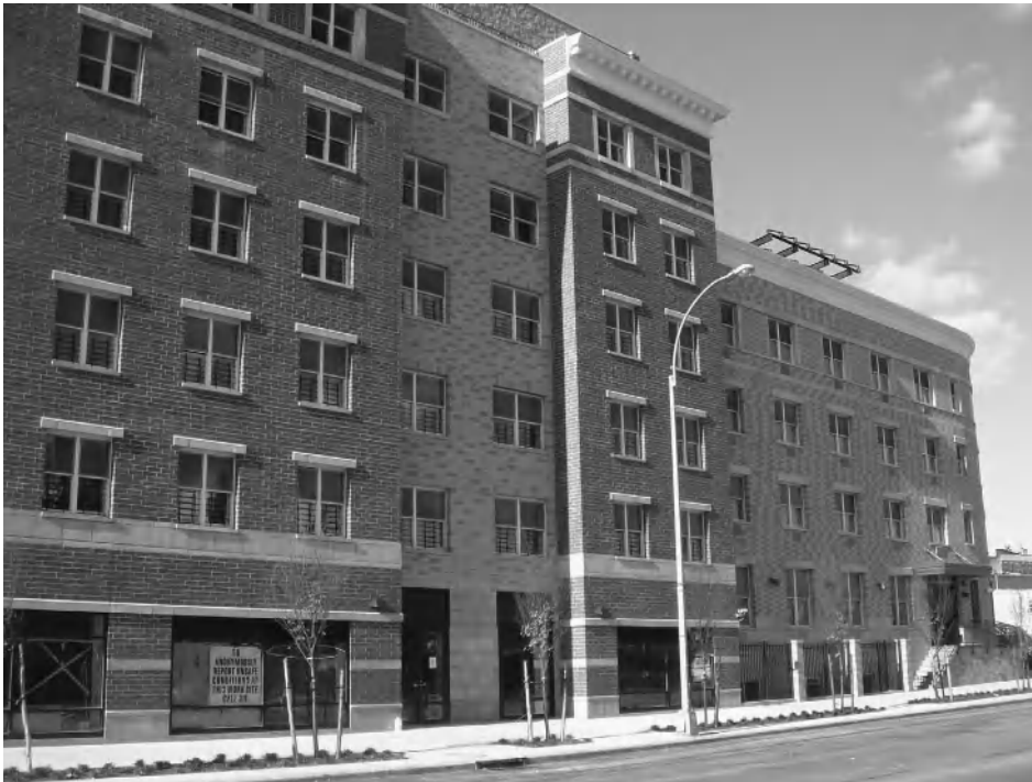
Figure 3-12 Intervale Green was built on a long-vacant site once visited by President Jimmy Carter to bring attention to urban decay. A few years later, the shoot-out scene in the movie Fort Apache, the Bronx was filmed there. Located only half a block from a subway station, the building is convenient to public transportation. Photo courtesy of WHEDCo.
