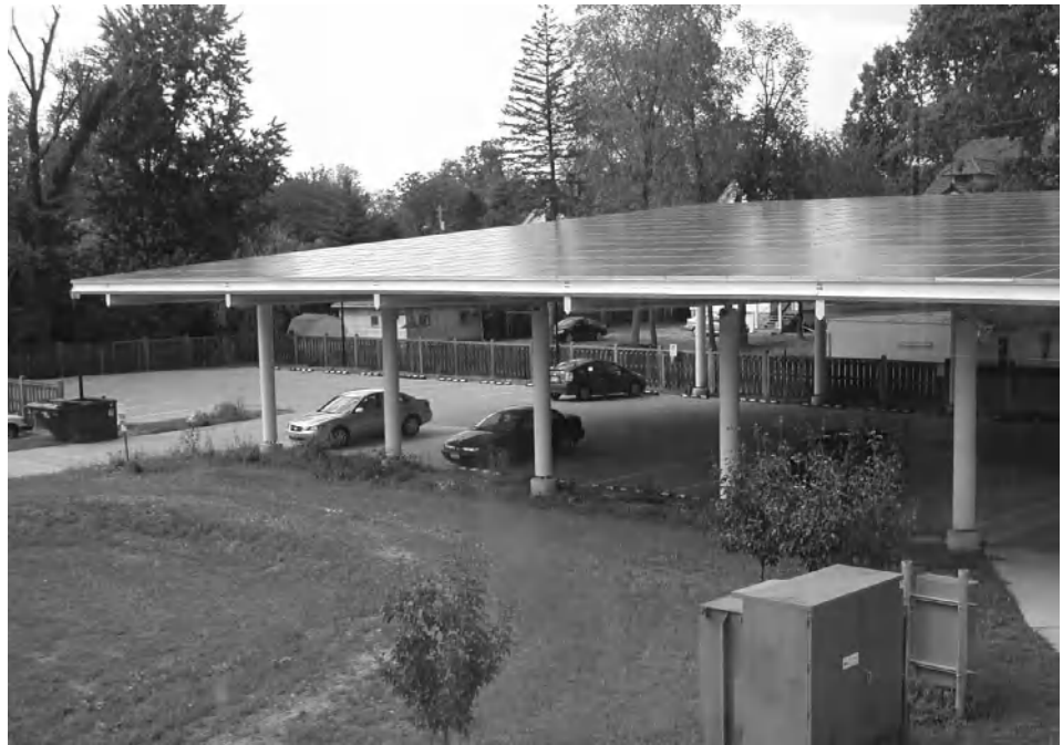
Figure 2-2 This parking canopy covered with solar photovoltaic panels produces electricity for the adjacent Adam Joseph Lewis Center for Environmental Studies at Oberlin College, Oberlin, Ohio. Photo courtesy of Bonnie Yelverton.
