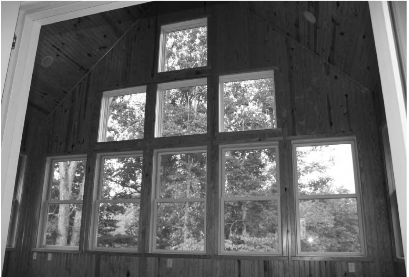
Figure 3-5 South-facing windows are shaded by deciduous trees in the summer, allowing for solar heat gain in the winter. Photo by Isaac Zuercher.
