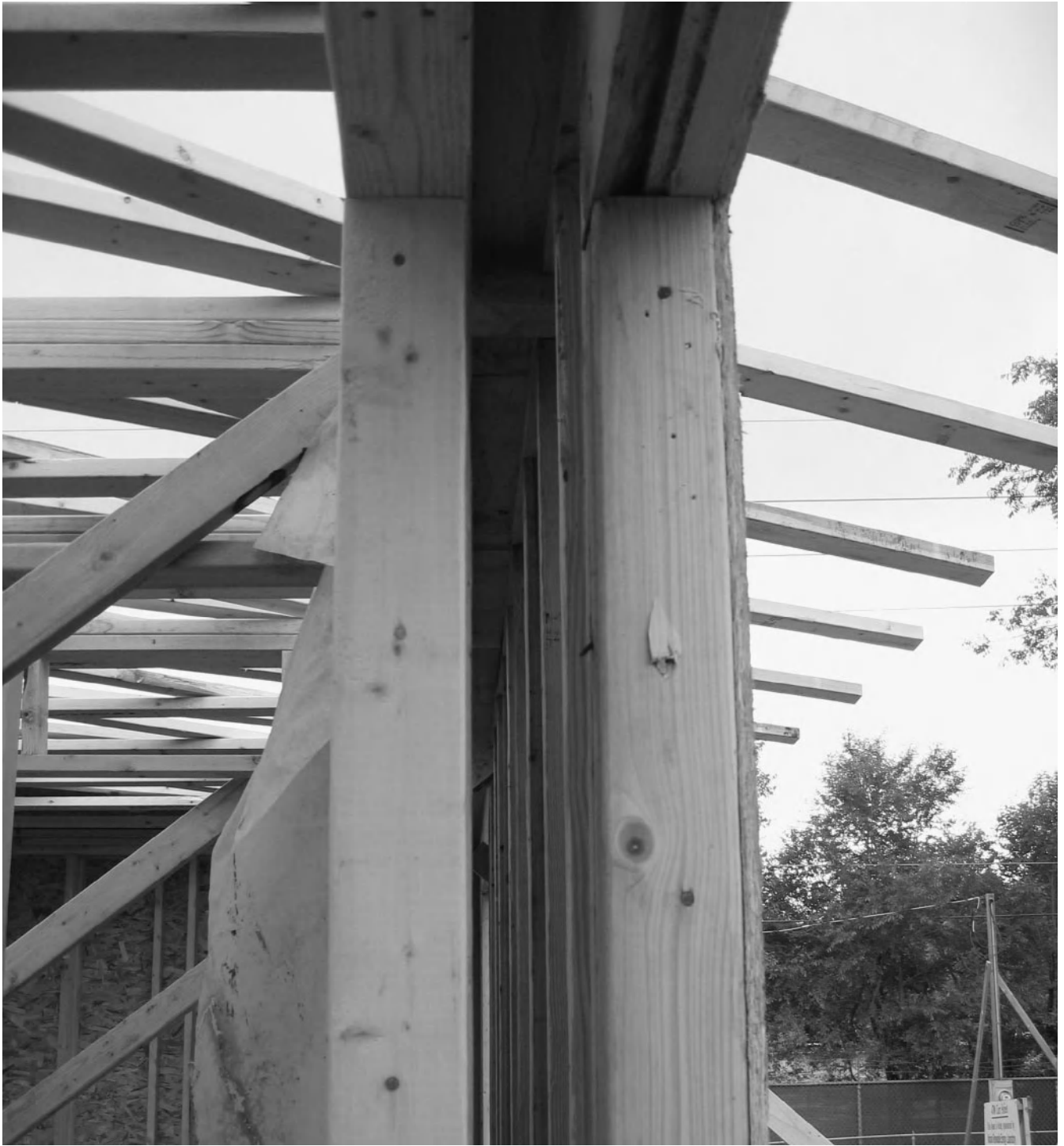
Figure 6-2 The double-stud wall construction creates a thermal break for a high-performance exterior wall. This home was constructed as a net-zero energy home by Habitat for Humanity of Metro Denver, with the assistance of the National Renewable Energy Laboratory (NREL). Photo by Paul Norton. Courtesy of DOE/NREL.
