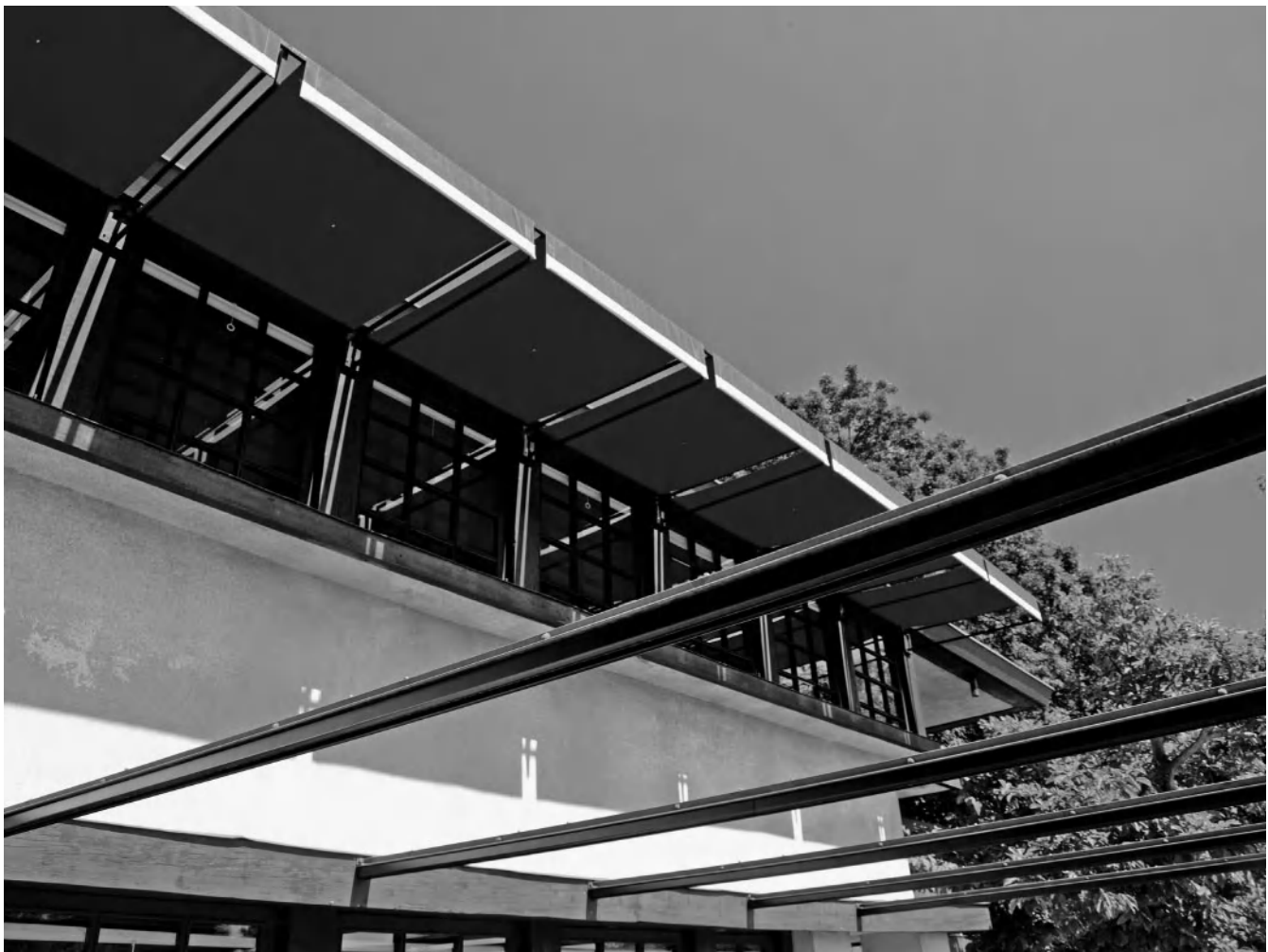
Figure 1-1 Awnings like these on Frank Lloyd Wright’s Westcott House in Springfield, Ohio, have been reducing solar gain since well before “green” was a type of building. Photo © 2007, Joseph M. Knapp.
