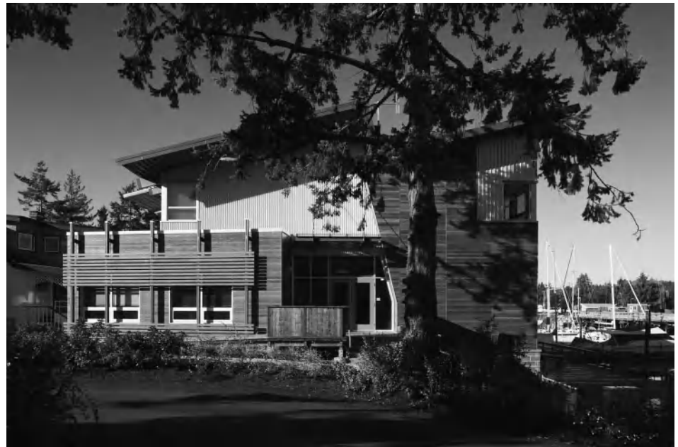
Figure 12-4 The Gulf Islands Operation Center includes an ocean-based geothermal system and exterior sunshades. Photo by Derek Lepper. Courtesy of McFarland Marceau Architects Ltd.
