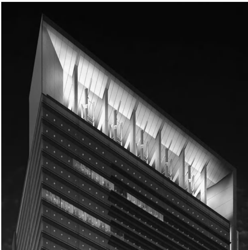
Figure 8-11 Wind turbines at the top of the Discovery Tower are a visible reminder of the building's sustainable building program. Image property of Gensler.
