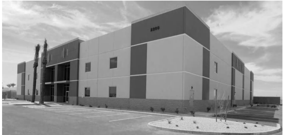
Figure 9-5 This office and warehouse building is located adjacent to the Chandler Municipal Airport. The building received high marks for site design and enhancements which minimized its environmental impact. Photo courtesy of Jack MacDonough.
