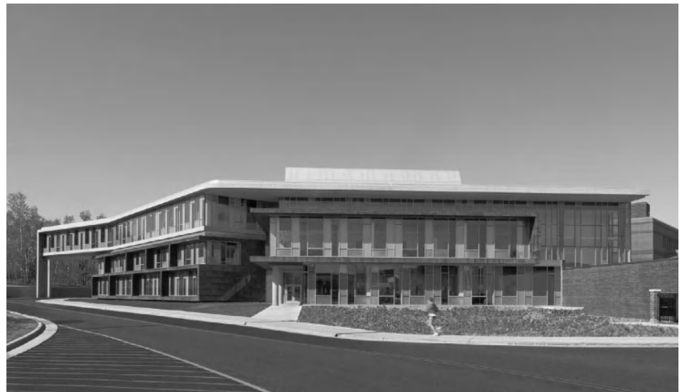
Figure 10-7 Energy models were created at three different points in the design process. The project achieved eight LEED points by being 51 percent more energy efficient than ASHRAE 90.1-1999. Photo by James Steinkamp. © 2009, Steinkamp Photography.
