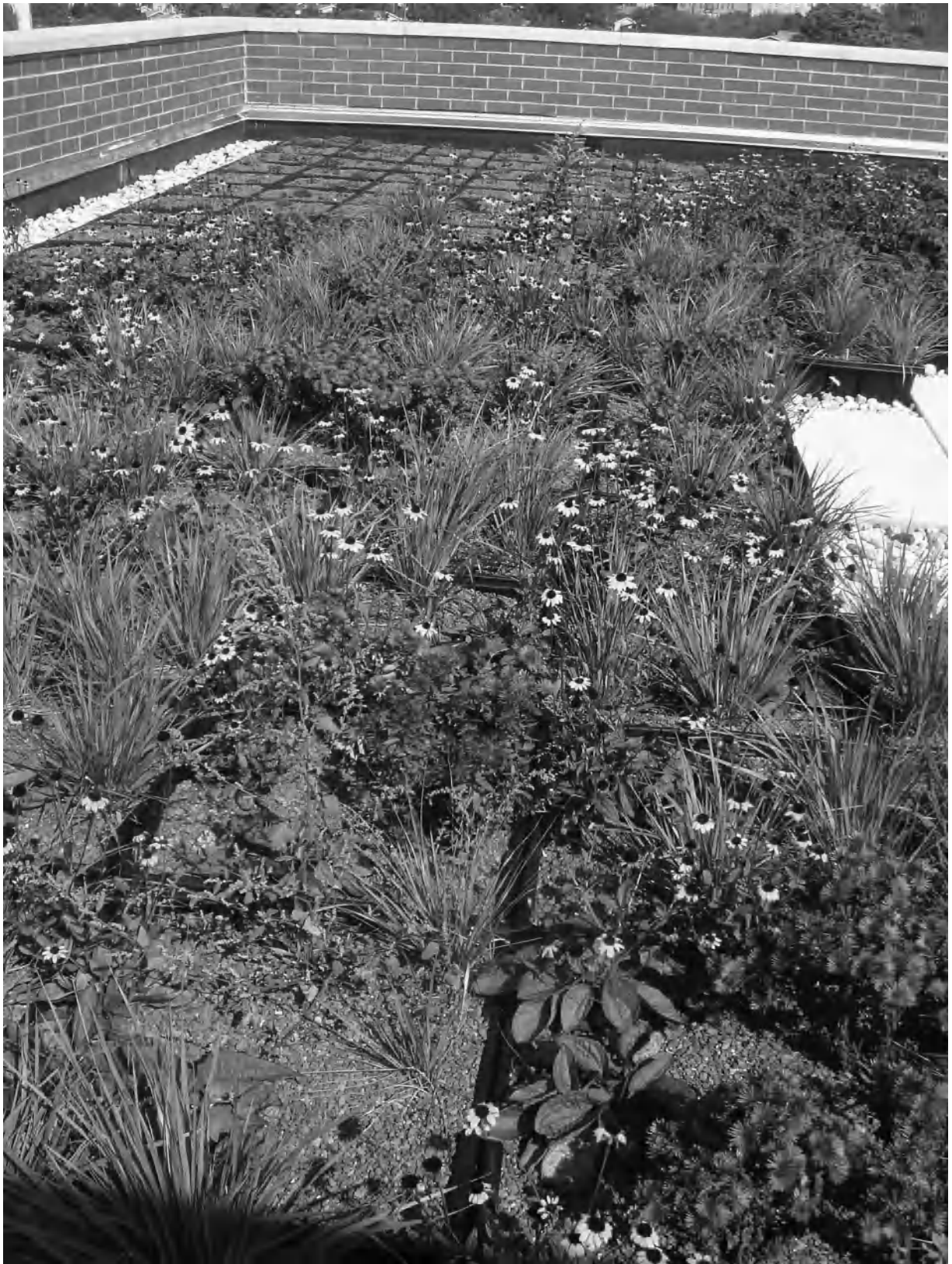
Figure 3-13 The project has 20,000 square feet of green roof, some of it accessible to residents. Residents also have access to two private courtyards and a public sculpture garden featuring the work of local Bronx artists. Photo courtesy of WHEDCo.
