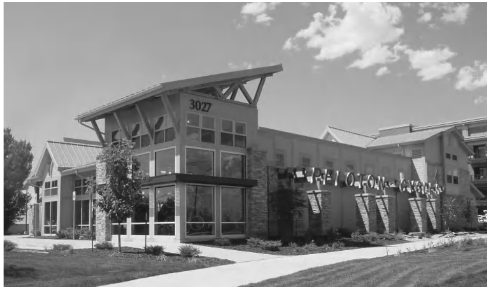
Figure 8-4 Part of the roof is made with structural insulated panels (SIPs), contributing to the high R-value of the building envelope. © 2009, Architecture West, LLC.
