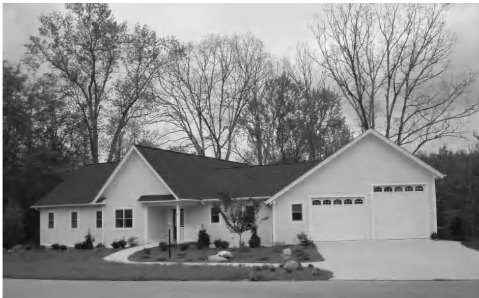
Figure 3-4 Situated in a retirement community, this home is accessible to wheelchair users. Photo by Isaac Zuercher.
