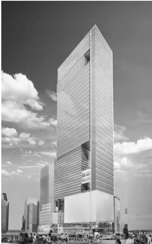
Figure 12-3 Hysan's Hennessy Centre Redevelopment project, designed by Kohn Pederson Fox Associates, is expected to earn Platinum-level certification for both HK-BEAM and LEED upon its completion in 2011. The 36-story, 710,000-square-foot mixed-use office and retail building will incorporate natural daylight and ventilation, low-e double glazing, sunshades designed for different solar orientations, and recycled and recyclable materials. Image courtesy of Kohn Pederson Fox Associates.
