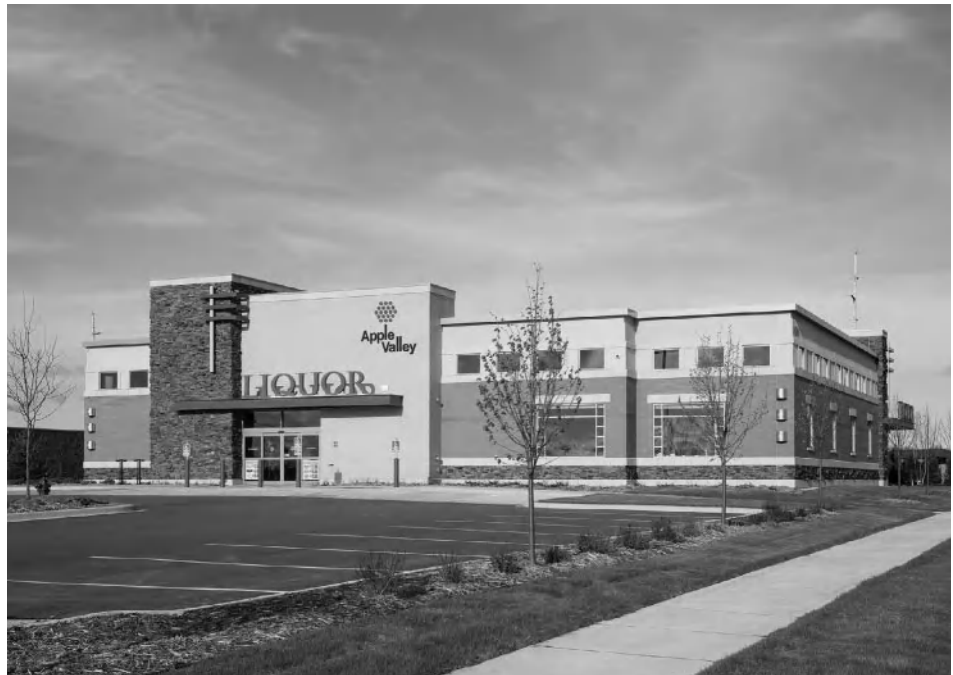
Figure 9-7 The natural stone on the façade, Minnesota Greenolite, is from a quarry less than 250 miles from the building site. Photo by Brian Droege. Courtesy of CNH Architects.
