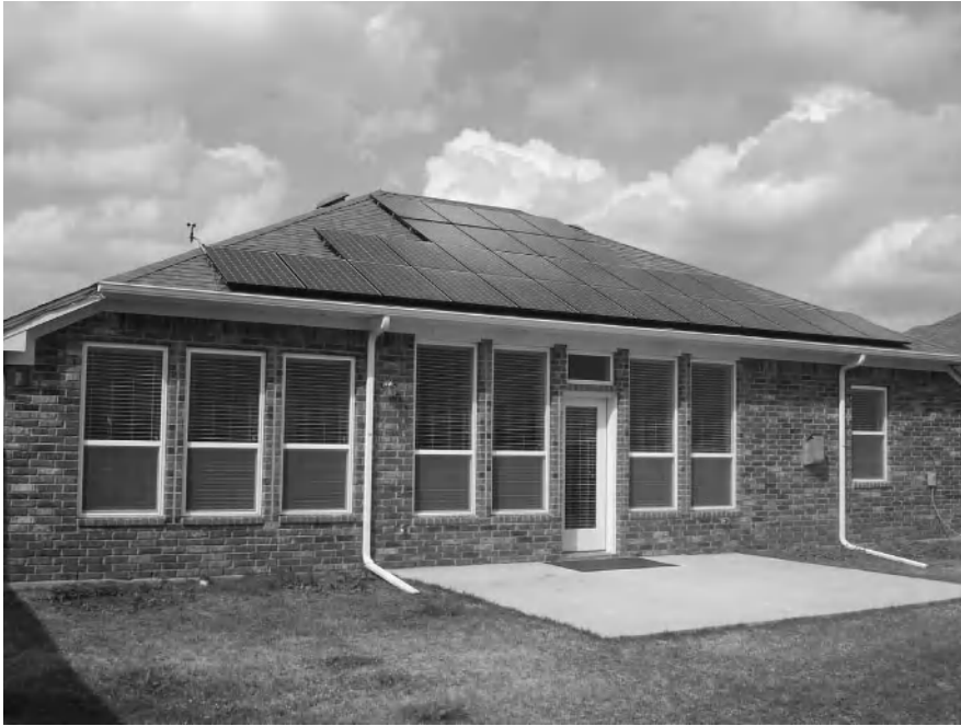
Figure 4-1 South-facing solar photovoltaic panels generate energy while the roof overhang provides some relief from the summer sun. Photo courtesy of Ideal Homes, www.Ideal-Homes.com.
