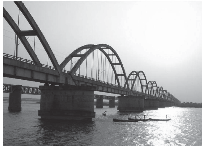
FIG. 18.3 Godavari arch bridge
