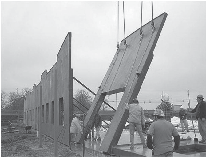
FIG. 2.14 Tilt-up wall construction Courtesy: Insul-Deck LLC, www.insuldeck.com
