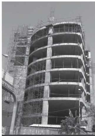
FIG. 2.24 Typical rigid, jointed RC framed buildings under construction in Chennai, India
