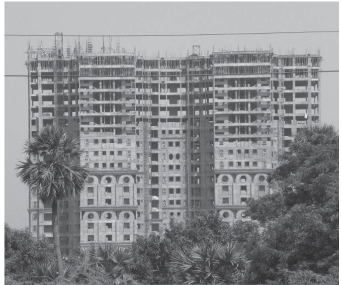
FIG. 20.1 Construction of a multi-storey building in Chennai
