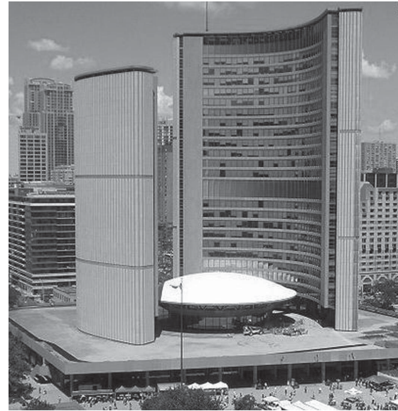
FIG. 2.25 Typical shear wall-frame system (a) Plan (b) The City Hall of Toronto, Ontario, Canada
