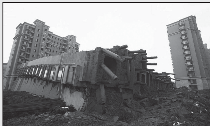
Toppling of building in China
