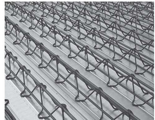
FIG. 11.31 Lattice shear reinforcement suggested by Park, et al. (2007) (Reprinted with permission from ACI)
