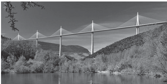
FIG. 13.7 Piers of Millau Viaduct, France
