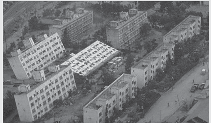
Tilting of apartments
