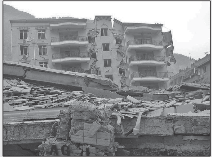
Complete collapse of RC buildings during the 2008 Sichuan earthquake
