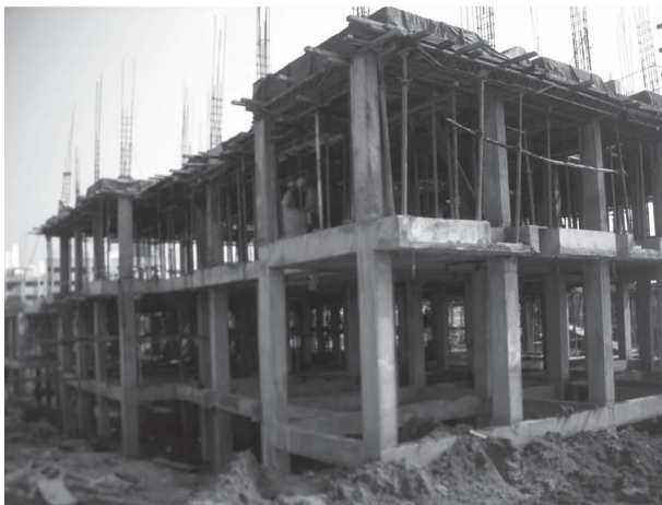
FIG. 2.24 Typical rigid, jointed RC framed buildings under construction in Chennai, India
