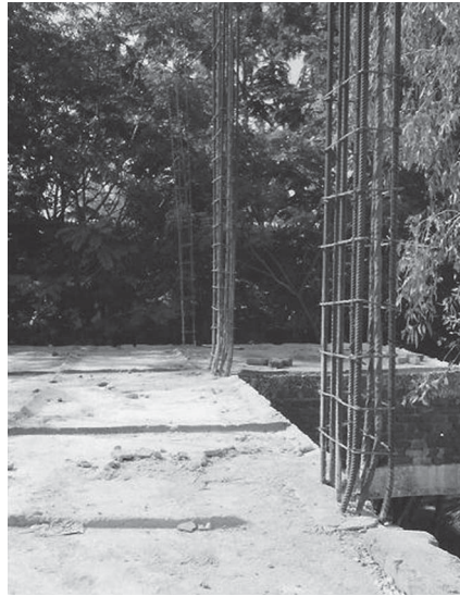
FIG. 13.19 Continuous columns (a) Small offset in continuous columns (b) Kinking of bars
