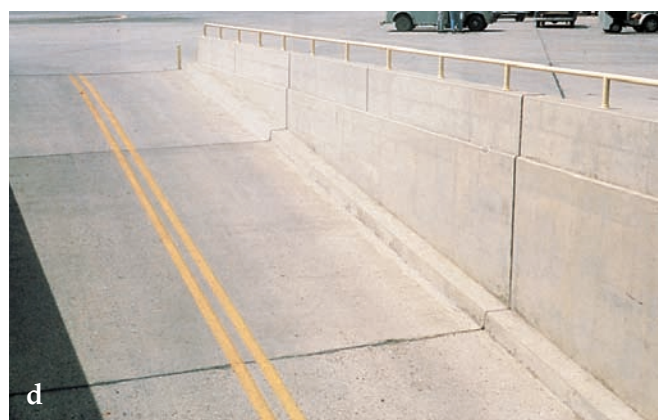
Figure 10-10. (a) Illustration showing no crack development in concrete that is free to shrink (slab on rollers); however, in reality a slab on ground is restrained by the subbase (or other elements) creating tensile stresses and cracks. (b) Typical shrinkage cracks in a slab on ground. (c) A properly functioning contraction joint controls the location of shrinkage cracking. (d) Contraction joints in the slabs and walls shown will minimize the formation of cracks.
