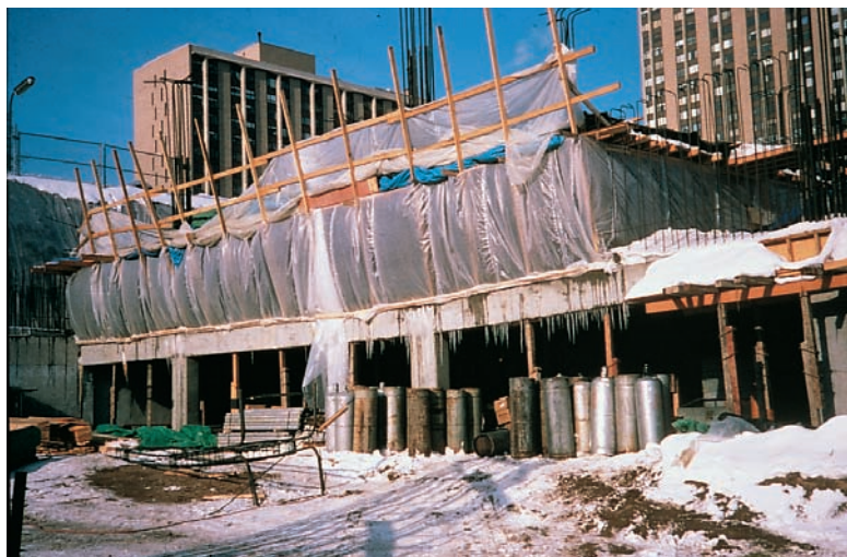
Figure 17-1. When suitable preparations to build enclosures and insulate equipment have been made, cold weather is no obstacle to concrete construction.
