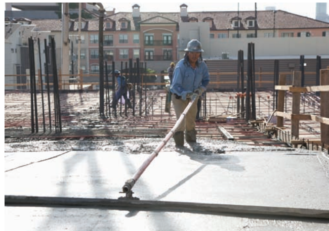
Figure 14-23. Highway straightedges are used on highway pavement and floor construction where very flat surfaces are desired (Courtesy of Baker Concrete).
