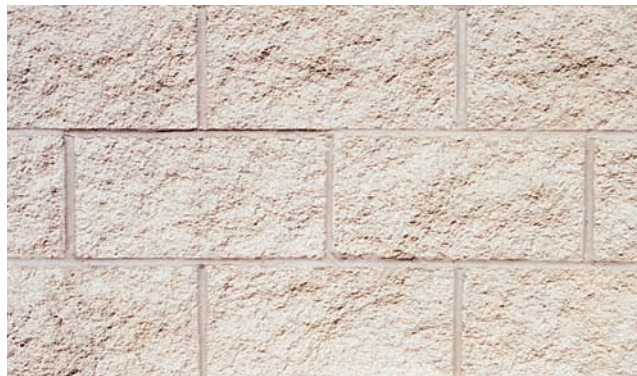
Figure 3-22. Masonry cement and mortar cement are used to make mortar to bond masonry units together.
