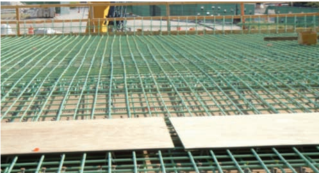
Figure 8-6. Epoxy-coated reinforcing bars.
