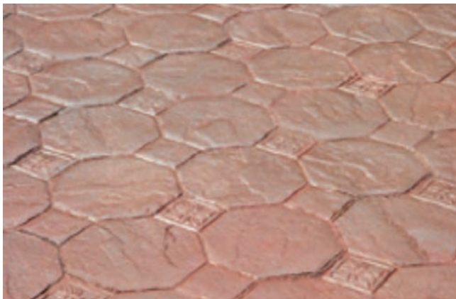
Figure 9-32. Pattern-stamped finish and colored surfaces are popular for decorative concretes.
