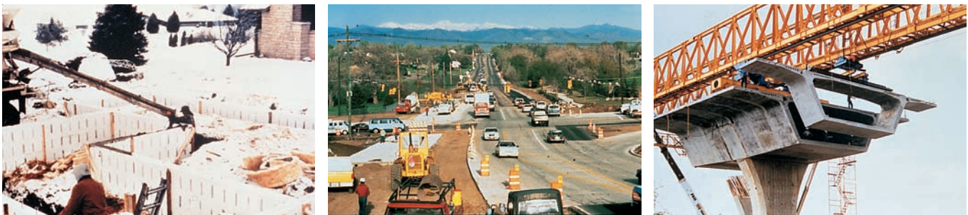
Figure 3-19. High early strength cements are used where early concrete strength is needed, such as in (left to right) cold weather concreting, fast track paving to minimize traffic congestion, and rapid form removal for precast concrete.
