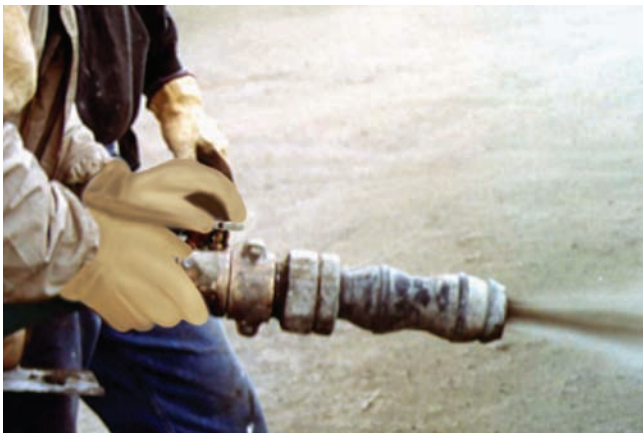
Figure 13-17. Shotcrete is pneumatically applied concrete.
