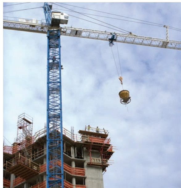
Figure 13-12. The tower crane and bucket can easily handle concrete for tall-building construction (Courtesy of Baker Concrete).
