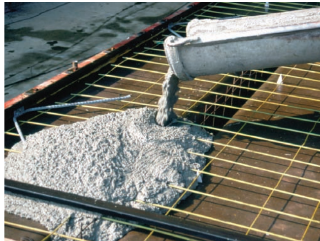
Figure 8-8. Welded wire reinforcement (Courtesy of BASF).
