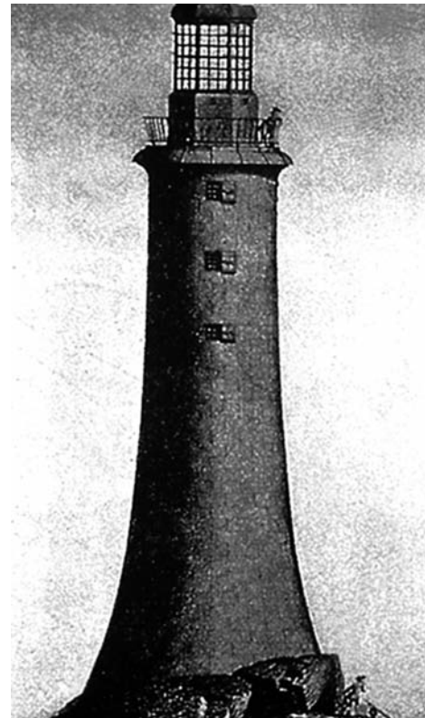
Figure 1-9. Eddystone lighthouse constructed of natural cement by John Smeaton.
