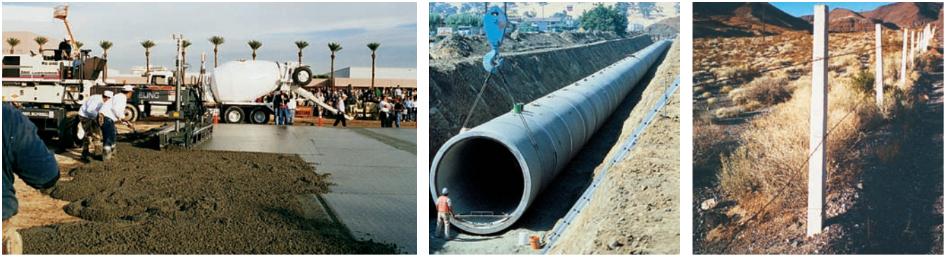
Figure 3-16. Moderate sulfate resistant cements and high sulfate resistant cements improve the sulfate resistance of concrete elements, such as (left to right) slabs on ground, pipe, and concrete posts exposed to high-sulfate soils.
