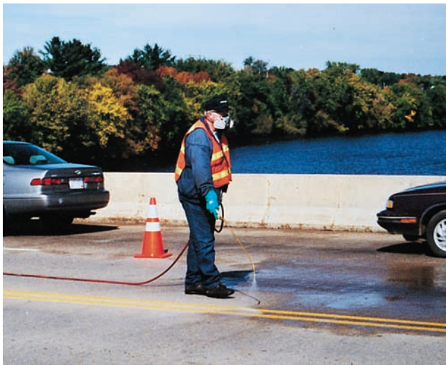
Figure 15-13. Penetrating sealers help protect reinforcing steel in bridge decks from corrosion due to chloride infiltration without reducing surface friction.
