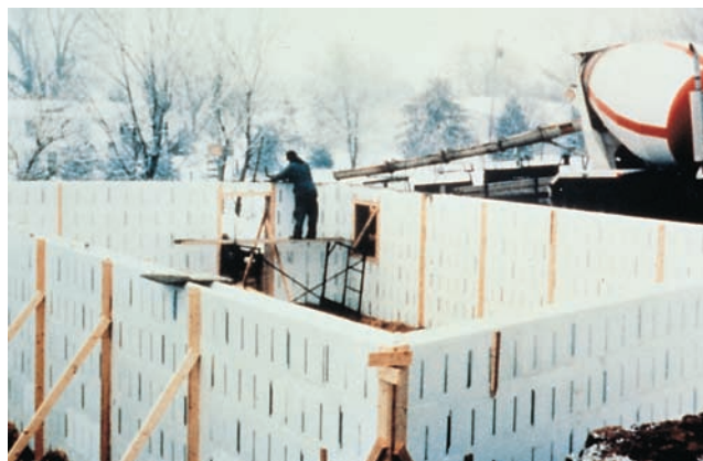
Figure 17-20. Insulating concrete forms (ICF) permit concreting in cold weather.
