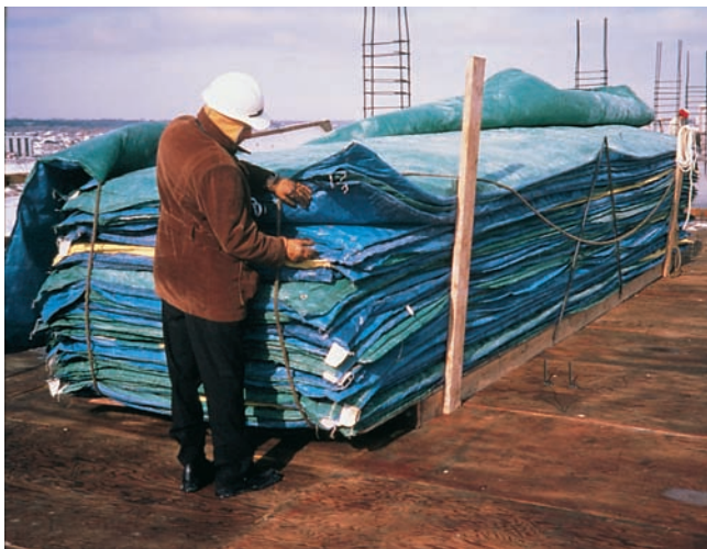
Figure 17-19. Stack of insulating blankets. These blankets trap heat and moisture in the concrete, providing beneficial curing.
