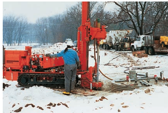
Figure 3-24. (top) A slurry of finely ground cement and water can be injected into the ground, as shown here, to stabilize in-place materials, to provide strength for foundations, or to chemically retain contaminants in soil. Illustration (right) of grout penetration in soil.
