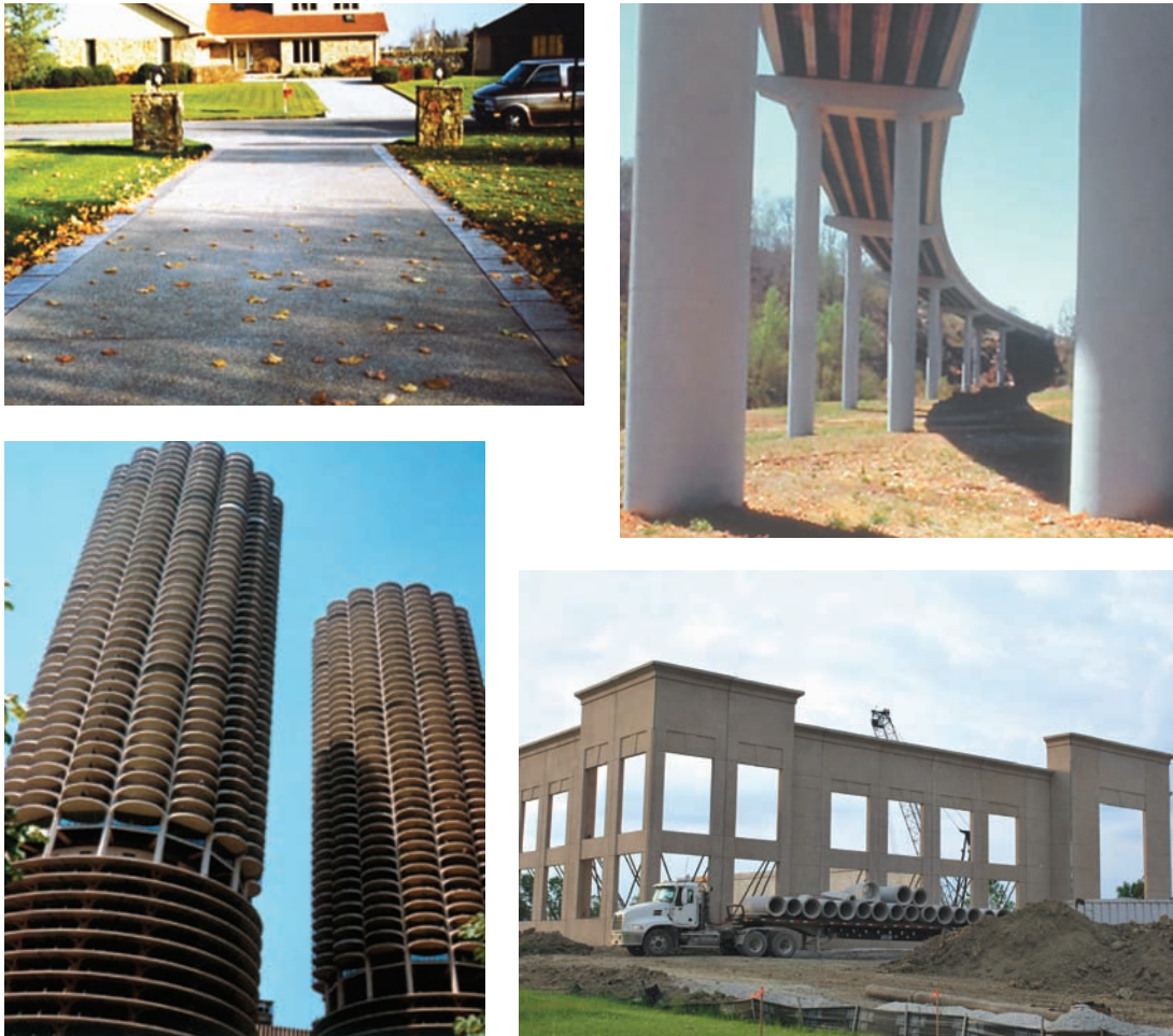
Figure 1-7. Concrete's primary markets include: pavements, bridges, and high-rise and low-rise buildings.
