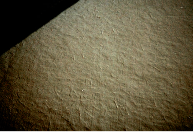
Figure 8-15. Bridge deck with steel fibers.
