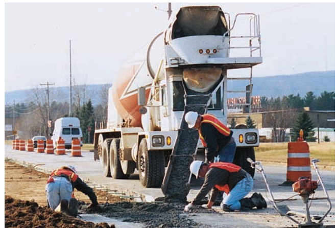
Figure 13-11. In comparison to conventional rear-discharge trucks, front-discharge truck mixers provide the driver with more mobility and control for direct discharge into place.
