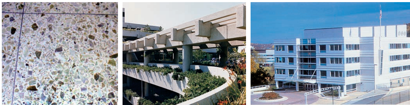
Figure 3-20. White portland cement is used in white or light-colored architectural concrete, ranging from (left to right) terrazzo for floors shown here with white cement and green granite aggregate, to decorative and structural precast and cast-in-place elements, to building exteriors. The far right photograph shows a white precast concrete building housing the ASTM Headquarters in West Conshohocken, Pennsylvania (Courtesy of ASTM).
