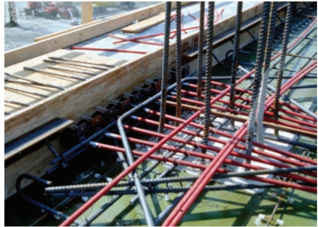
Figure 8-11. Post-tensioning tendon layout.
