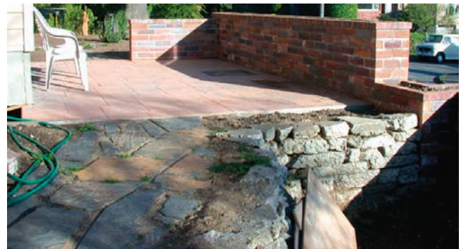
Figure 2-10. This 25,450 L (7000 gallon) concrete cistern has a colored and stamped top to double as a patio (Courtesy of www.sensiblehouse.org ).
