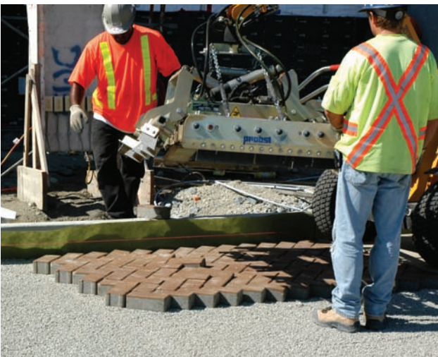
Figure 2-8. Interlocking concrete pavers allow water to infiltrate between the units (Courtesy of ICPI).
