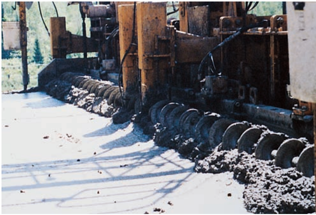
Figure 13-16. The screw spreader quickly spreads concrete over a wide area to a uniform depth. Screw spreaders are used primarily in pavement construction.
