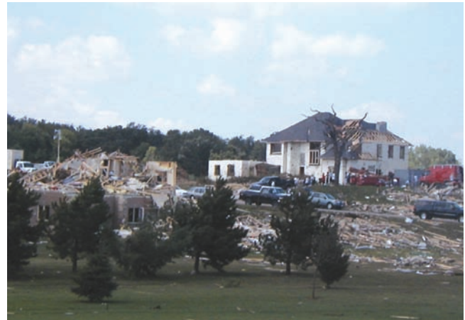
Figure 2-2. The concrete home shown still standing survived a tornado in Wisconsin. This is a prime example of the resistance of concrete structures to tornado forces.
