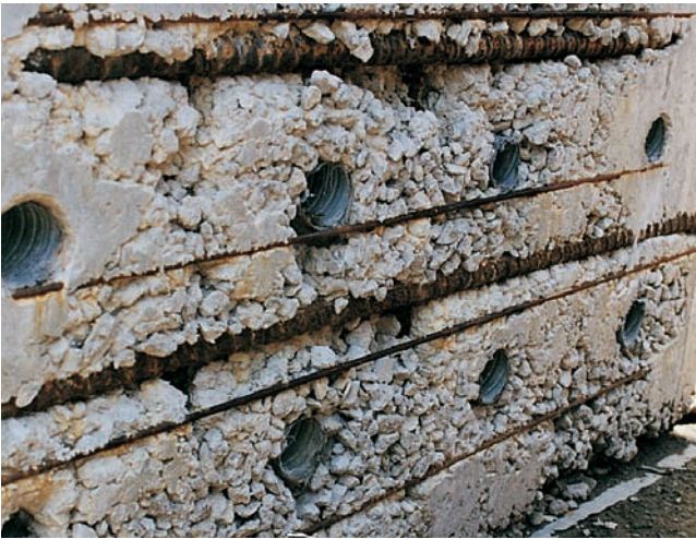
Figure 9-18. Poor consolidation can result in early corrosion of reinforcing steel and low compressive strength.
