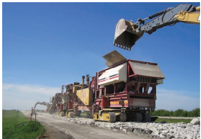
Figure 2-13. Paving trains can recycle existing concrete pavement. The crushed concrete can be used as aggregate in new concrete or as base material (Courtesy of NCPTC).
