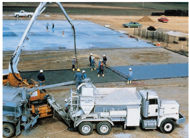
Figure 13-7. Mobile batcher measures materials by volume and continuously mixes concrete as the dry ingredients, water, and admixtures are fed into a mixing trough at the rear of the vehicle.
