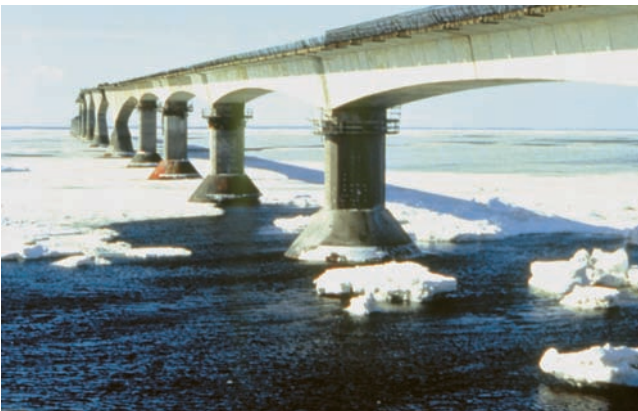
Figure 11-1. The Confederation Bridge, (shown here under construction), is a concrete bridge in a severe environment with a 100 year design life.
