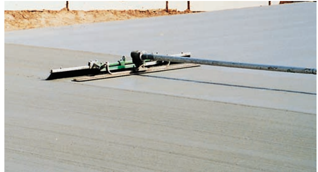
Figure 14-26. Brooming provides a slip-resistant surface mainly used on exterior concrete.
