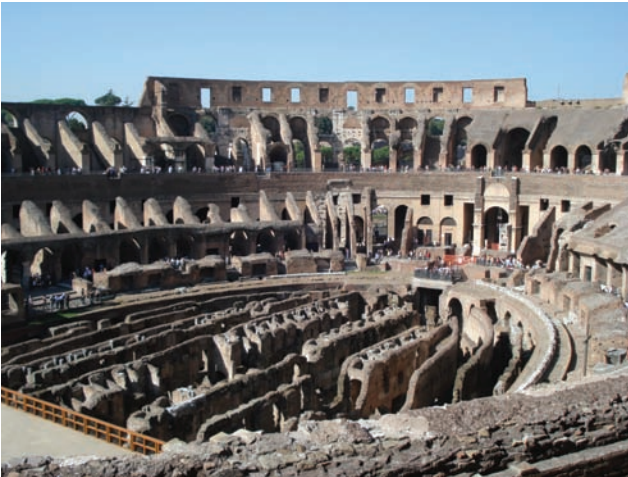
Figure 1-8. Coliseum in Rome, completed in 80 AD, was constructed of concrete. Much of it still stands today (Courtesy of J. Catella).
