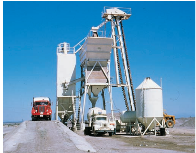
Figure 13-6. Truck-mixed concrete is mixed completely in a truck mixer.
