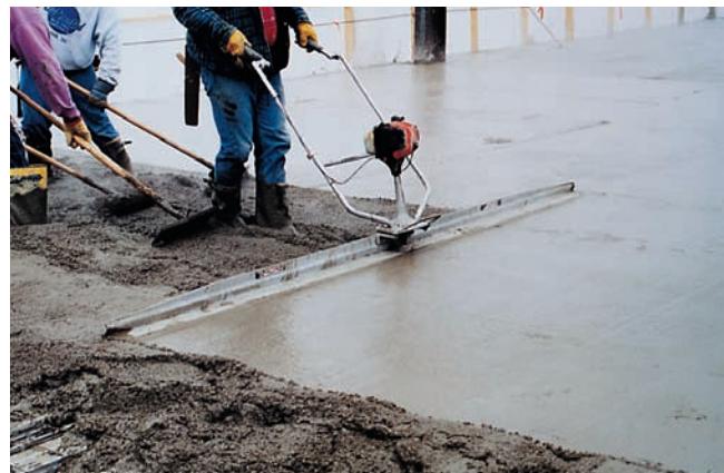
Figure 14-20. Where floor tolerances are not critical, an experienced operator using this vibratory screed does not need screed poles supported by chairs to guide the screed. Instead, the operator visually matches elevations to forms or previous passes. The process is called wet screeding.
