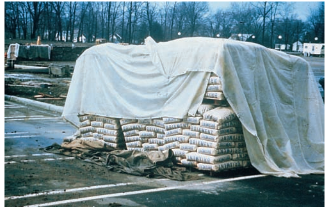
Figure 3-53. When stored on the job, cement should be protected from moisture.
