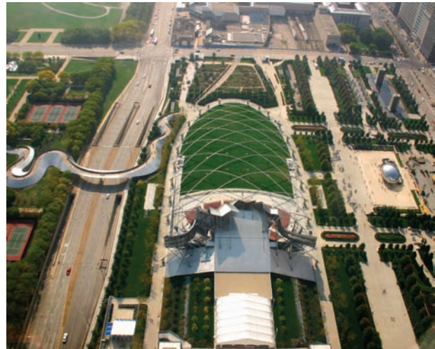
Figure 2-9. Chicago's Millennium Park is one of the largest green roofs and is built on top of a commuter rail station and two parking garages (Courtesy of J. Crocker).
