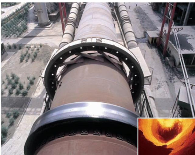
Figure 3-7. Rotary kiln (furnace) for manufacturing portland cement clinker. Inset view inside the kiln.
