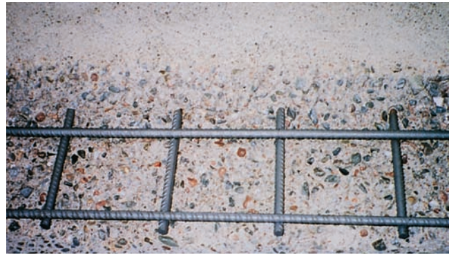
Figure 14-37. Concrete prepared for patch installation.
