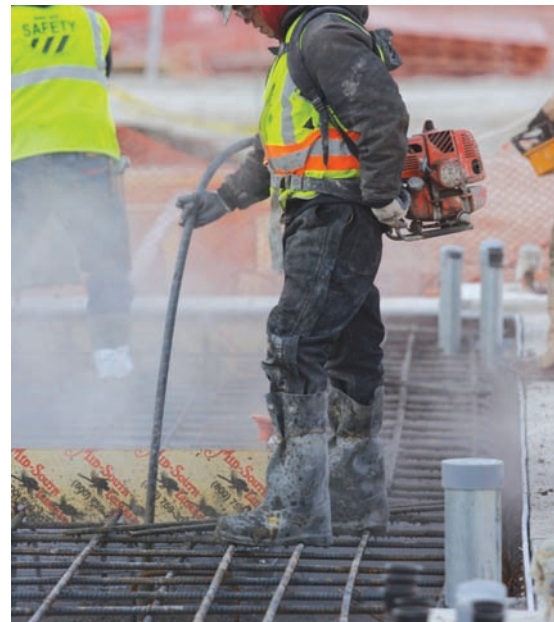
Figure 14-18. Internal vibrators are commonly used to consolidate concrete in walls, columns, beams, and slabs (Courtesy of Baker Concrete).
