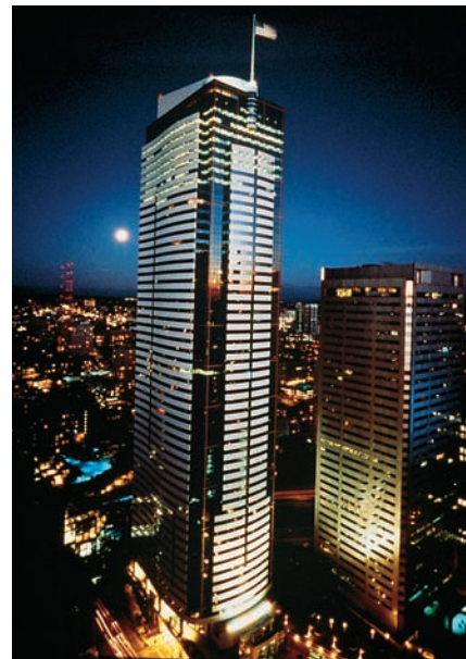
Figure 19-5. The Two Union Square building in Seattle used concrete with a designed compressive strength of 131 MPa (19,000 psi) in its steel tube and concrete composite columns. High-strength concrete was used to meet a design criterion of 41 GPa (6 million psi) modulus of elasticity.
