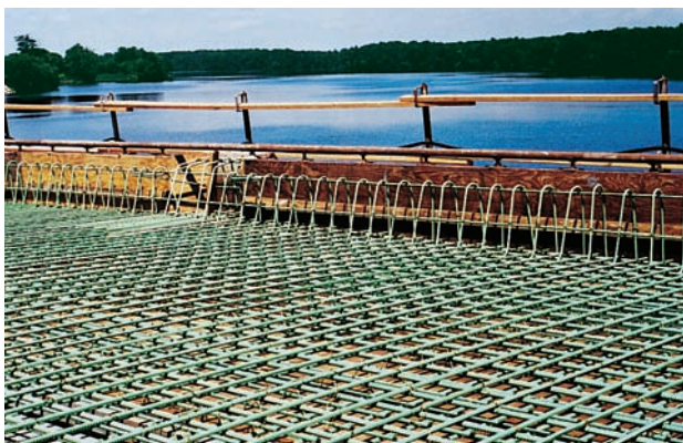
Figure 11-32. Epoxy-coated reinforcing steel used in bridge deck.
