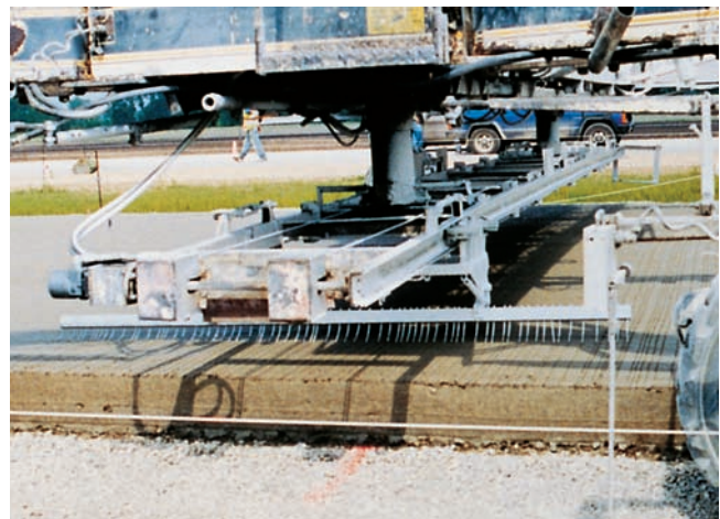
Figure 14-26. Brooming provides a slip-resistant surface mainly used on exterior concrete.
