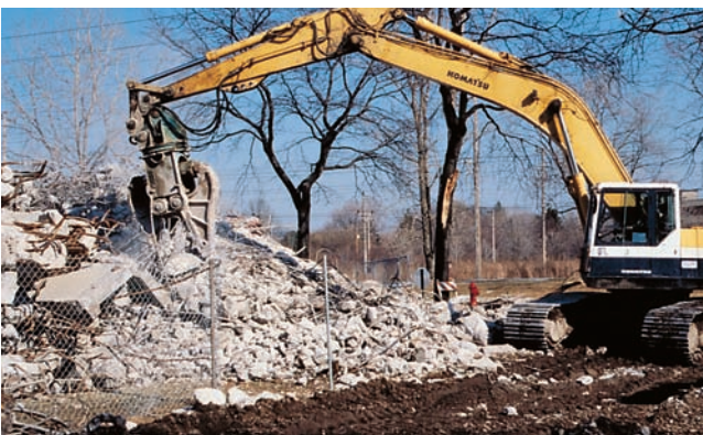
Figure 6-4. Heavily reinforced concrete is crushed with a beam-crusher.
