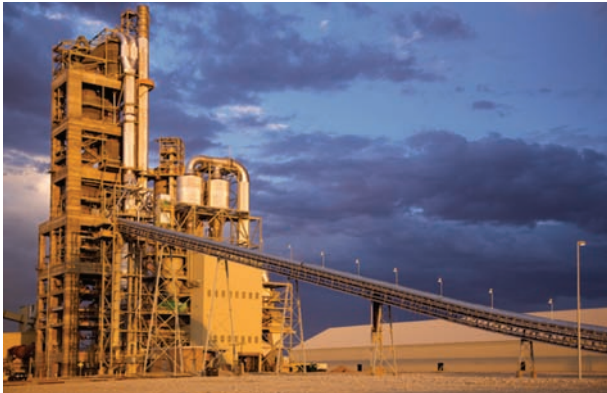
Figure 1-3. Portland cement manufacturing plant (Courtesy of GCC).
