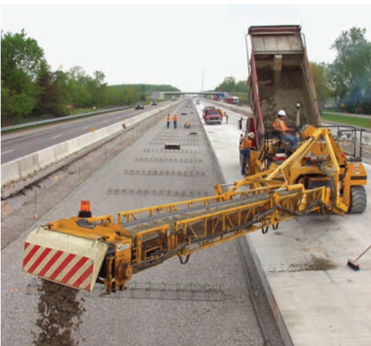
Figure 13-5. (top) Truck agitators are also used with central-mix batch plants. Agitation mixing capabilities allow truck agitators to supply concrete to projects with slow rates of concrete placement and at distances greater than nonagitating trucks. (bottom) Nonagitating trucks are used with central-mix batch plants where short hauls and quick concrete discharge (by conveyor, in this example) allows the rapid placement of large volumes of concrete (Courtesy of Gomaco).
