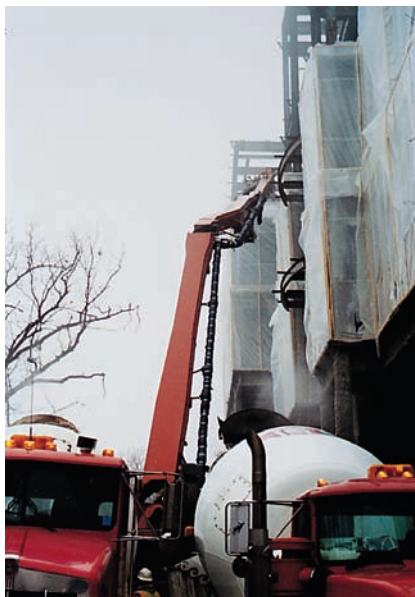
Figure 17-1. When suitable preparations to build enclosures and insulate equipment have been made, cold weather is no obstacle to concrete construction.
