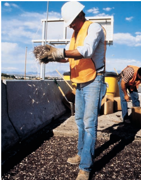
Figure 8-16. Tightly bunched steel fibers are placed in a form before cement slurry is poured into this application of slurry-infiltrated steel-fiber concrete (SIFCON).
