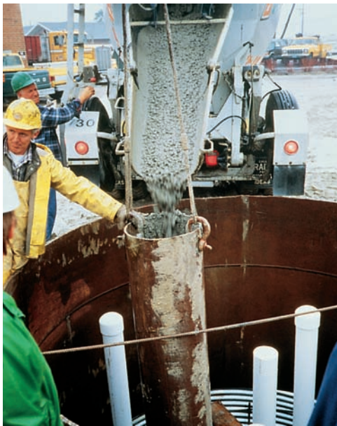
Figure 20-8. (left) A drilled pier (caisson), 3 m (10 ft) in diameter and 12.2 m (40 ft) in depth in which “low-heat” high-strength concrete is placed and (right) temperatures of this concrete measured at the center and edge and at three different levels in the caisson (Burg and Fiorato 1999).
