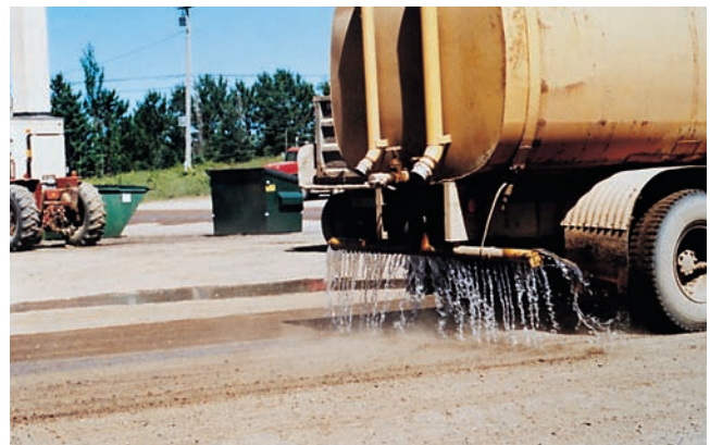
Figure 14-2. Water trucks with spray-bars are used to moisten subgrades and base course layers to achieve adequate compaction and to reduce the amount of water drawn out of concrete as it's placed.
