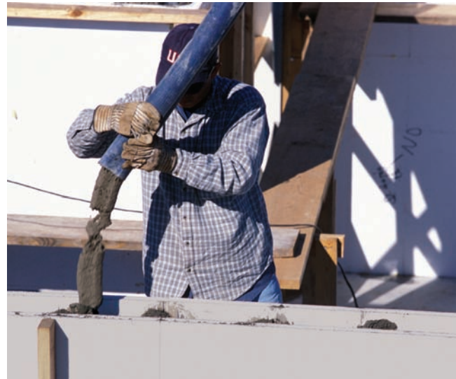
Figure 2-3. Insulating concrete forms (ICFs) provide thermal mass and high levels of insulation, key components for net-zero energy use buildings.
