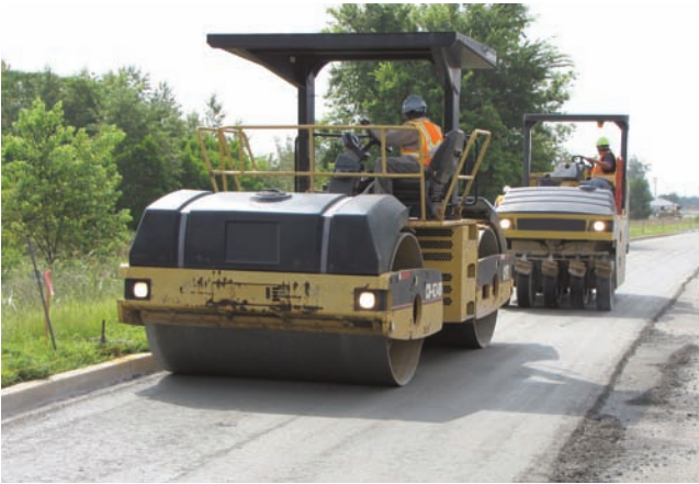
Figure 20-11. Vibratory rollers are used to compact roller-compacted concrete.
