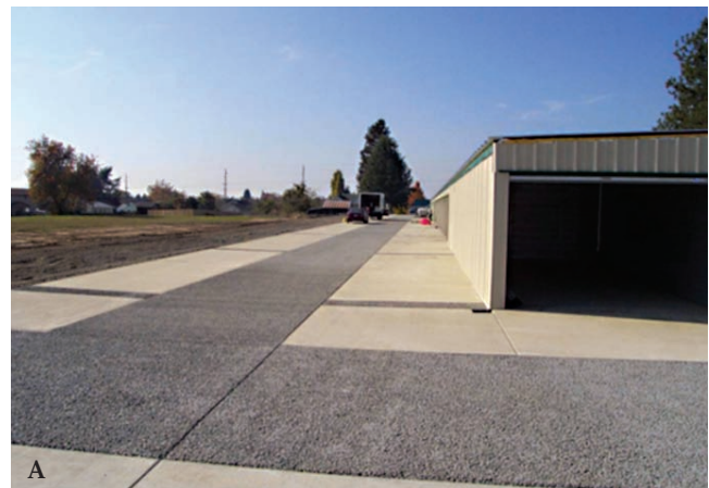
Figure 2-7. a) Pervious concrete allows for infiltration of water, reducing runoff from the site (Courtesy of B. Banka). b) Side view of water percolating through pervious concrete.
