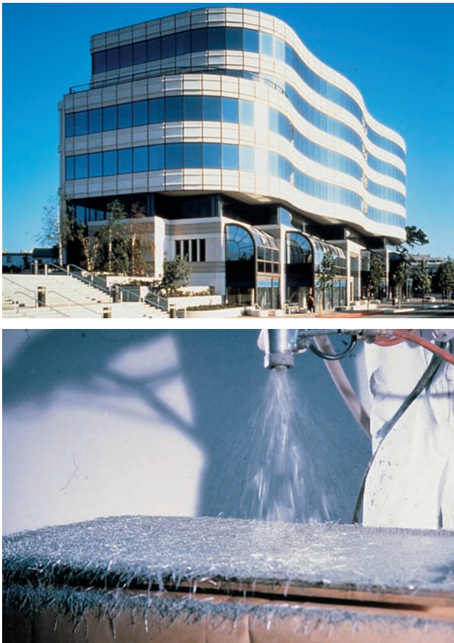
Figure 8-17. (top) Glass-fiber-reinforced concrete panels are light and strong enough to reduce this building's structural requirements. (bottom) Spray-up fabrication made it easy to create their contoured profiles.
