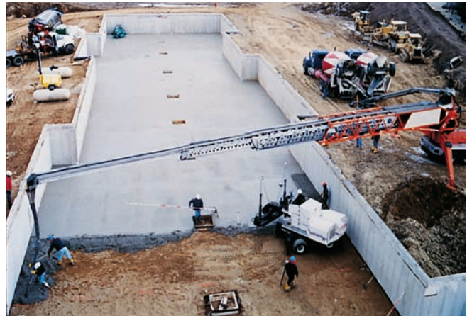
Figure 13-14. The conveyor belt is an efficient, portable method of transporting concrete.
