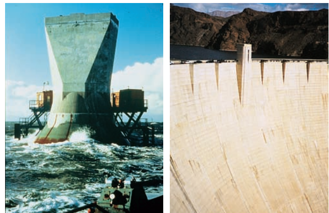
Figure 3-18. Moderate heat and low heat cements minimize heat generation in massive elements or structures such as (left) very thick bridge supports, and (right) dams. Hoover dam, shown here, used a Type IV cement to control temperature rise.
