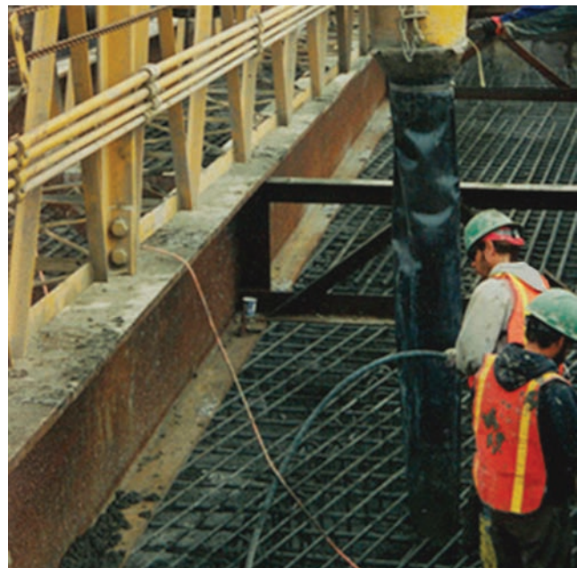
Figure 14-11. Dropchutes minimize the risk of segregation.
