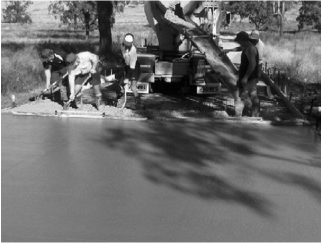
Figure 13.3 Placing of light pavement using geopolymer concrete.
