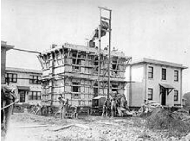
Figure 4.3 One of Edison's concrete houses under construction in 1919.
