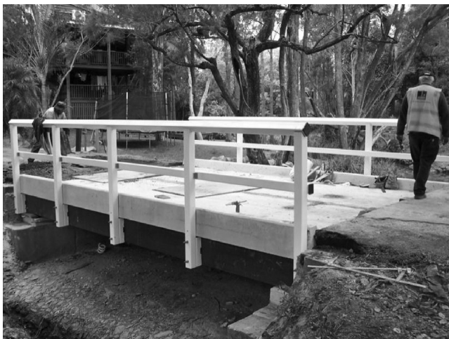
Figure 13.8 Composite pultruded girder and grade 40 geopolymer deck bridge in Brisbane.
