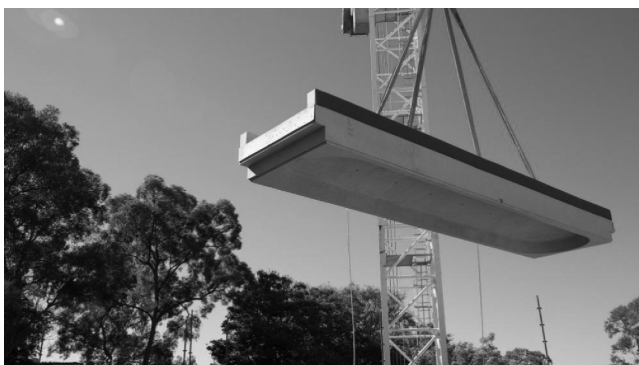
Figure 13.9 10.8 metre geopolymer beam with vaulted soffit being craned into position.
