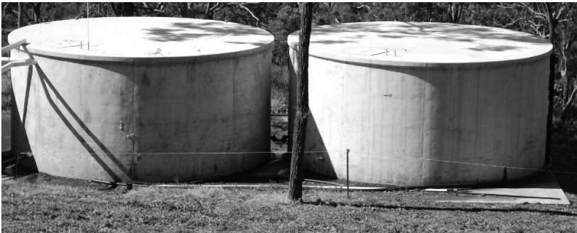
Figure 13.5 In situ water tanks cast with blended cement concrete (left) and geopolymer concrete (right).
