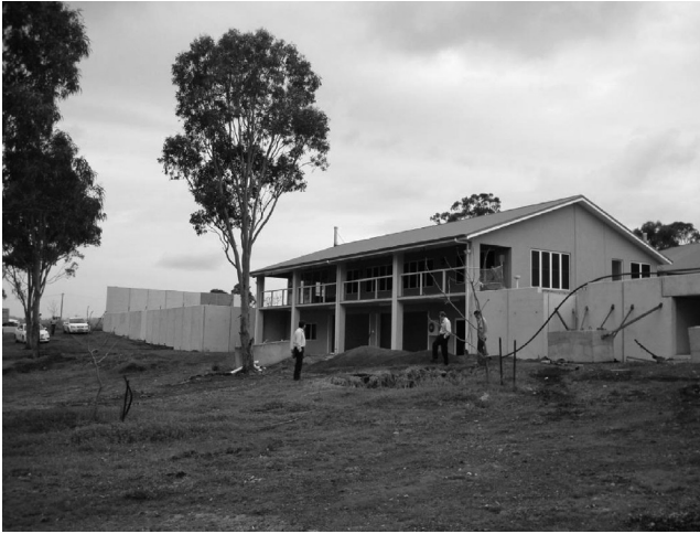
Figure 13.4 Precast geopolymer retaining walls for a private residence.
