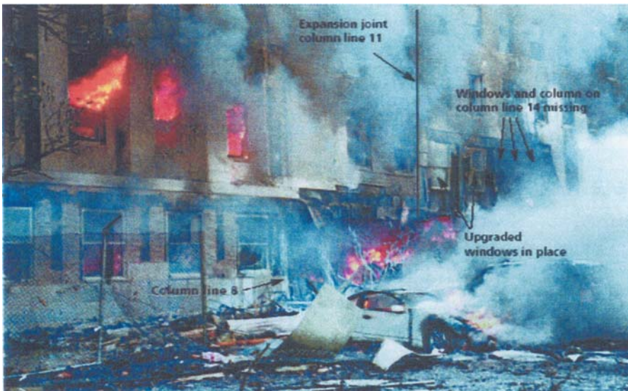
(b) (Color) Northern portion of impact area before collapse
