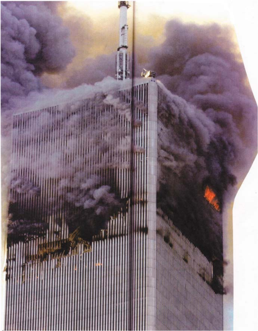
Fig. 1.13. WTC Tower with antenna-collapsed scenario: Tower I (courtesy: FEMA 2002, Washington, D.C.)
