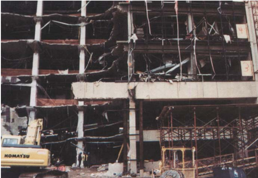
Fig. 10.37. Remains of the transfer girder
