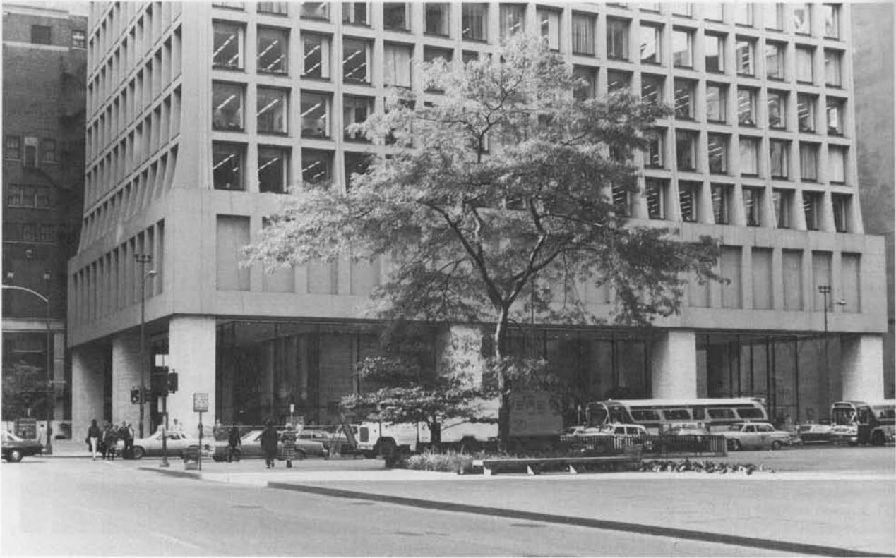
Fig. 17-26 Three-span deep beam, Brunswick building, Chicago. (Photograph courtesy of J. G. MacGregor.)
