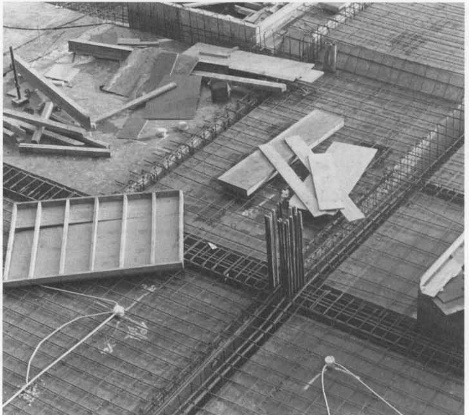
Fig. 5-22 Intersection of a column and two beams.
