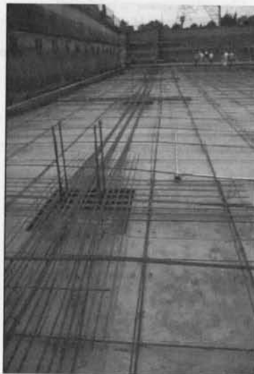
Fig. 13-103 Use of banded tendons in one direction and distributed tendons in other direction. (Photo courtesy of Kenneth Bondy)
