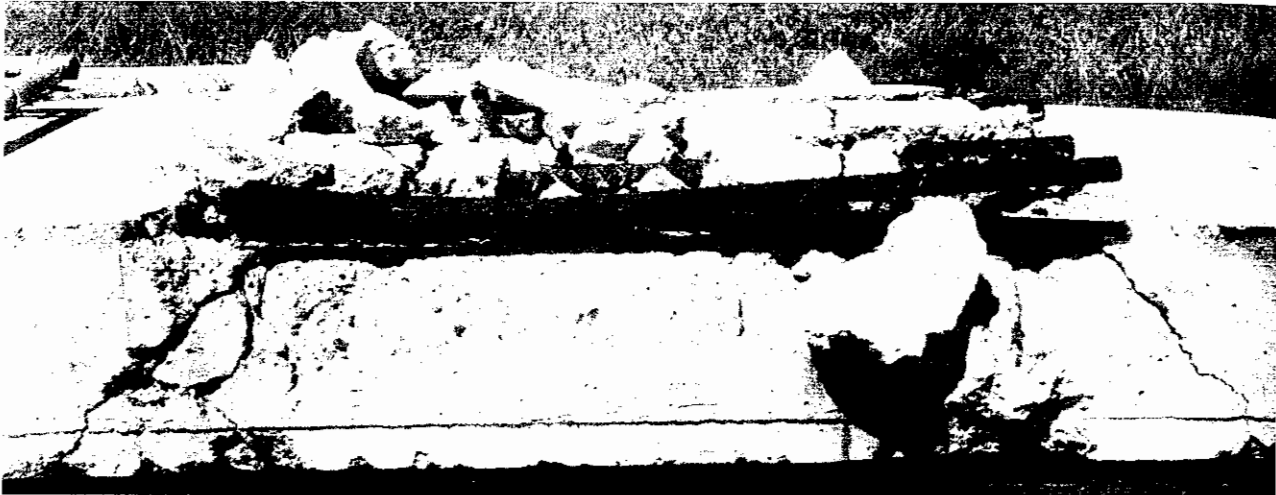
Fig. 8-32 Failure of a tension lap splice. (Photograph courtesy of J. G. MacGregor.)
