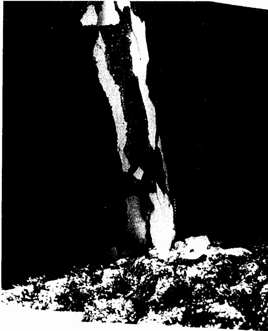
Fig. 11-7 Spiral column damaged by 1971 San Fernando earth- quake. Although this column has been deflected sideways 20 in., it is still carrying load. (Photograph courtesy of National Bureau of Standards.)
