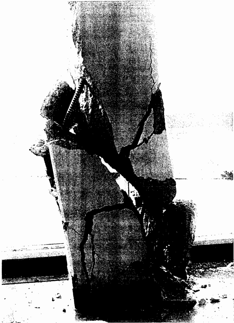
Fig. 6-41 Shear failure in a tied column, 1971 San Fernando earth- quake. (Photograph courtesy of U.S. National Bureau of Standards.)
