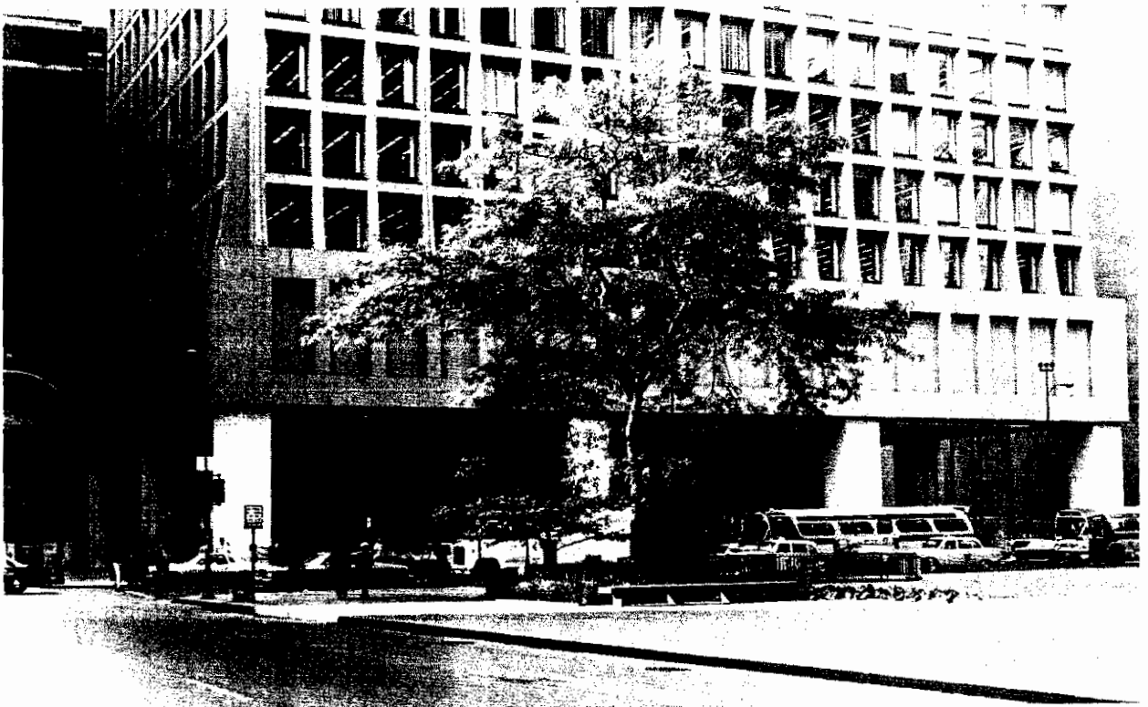
Fig. 18-28 Three-span deep beam, Brunswick building, Chicago. (Photograph by J. G. MacGregor.)
