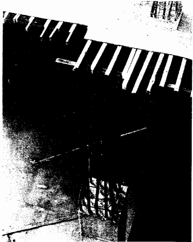
Fig. 11-1 Tied column under construction. (Photograph courtesy of J. G. MacGregor)
