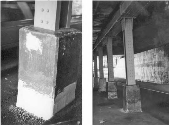
FIGURE 5.8 Concrete pedestals pretreated (left) and wrapped with a FRP fabric (right) (East Street Viaduct, West Virginia).
