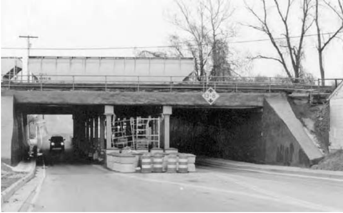
FIGURE 5.9 View of the restored wing wall, girder, and the abutment walls (East Street Viaduct, West Virginia).
