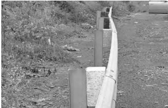
FIGURE 3.13 Field-installed highway guardrail offset blocks made of recycled polymers manufactured using a compression molding machine.
