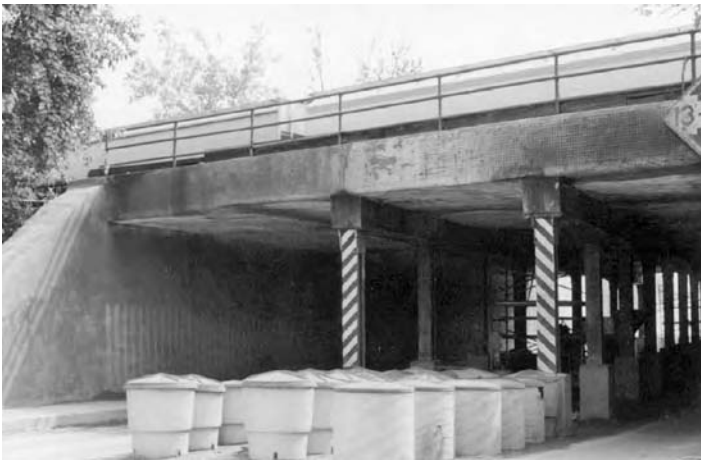
FIGURE 5.6 Wing wall and abutment being restored with GFRP (East Street Viaduct, West Virginia).
