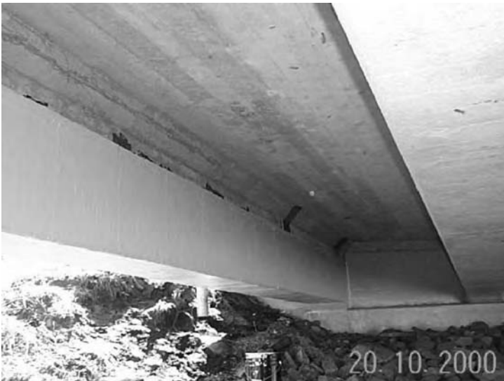
FIGURE 5.16 Finished interior of the external beam with carbon fabric and protective coating (Muddy Creek Bridge, West Virginia).
