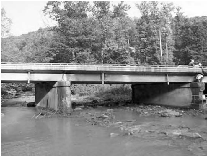
FIGURE 5.10 Muddy Creek Bridge (West Virginia) before wrapping.
