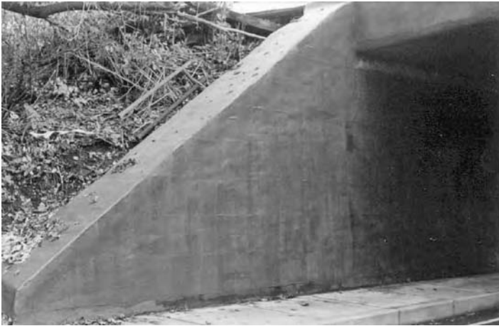
FIGURE 5.7 View of the restored wing wall (East Street Viaduct, West Virginia).
