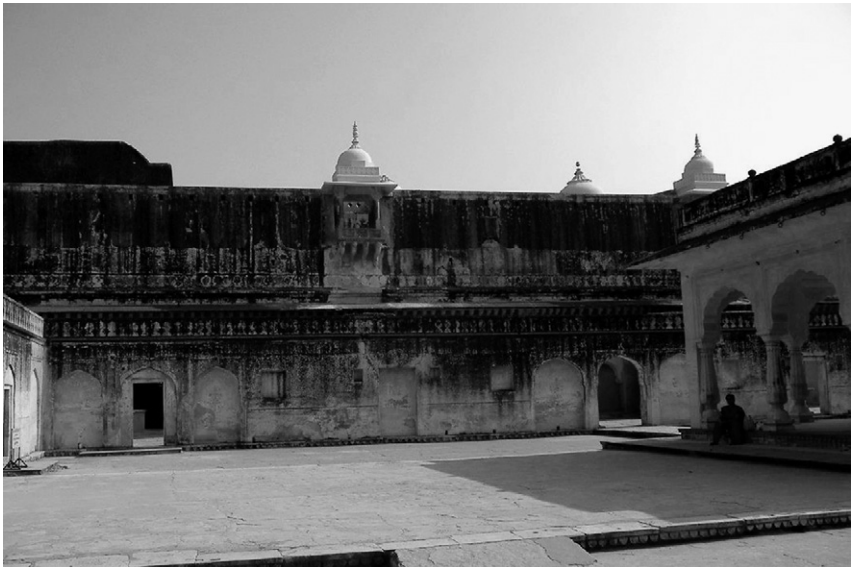
FIGURE 5.2 Black biofilms on the surface of the Ambar Fort in Jaipur, India.
