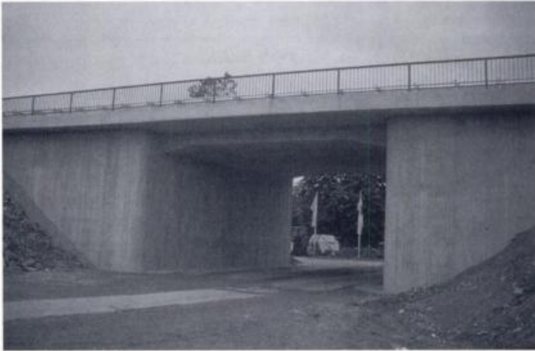
Fig. 2.2 Portal frame bridge
