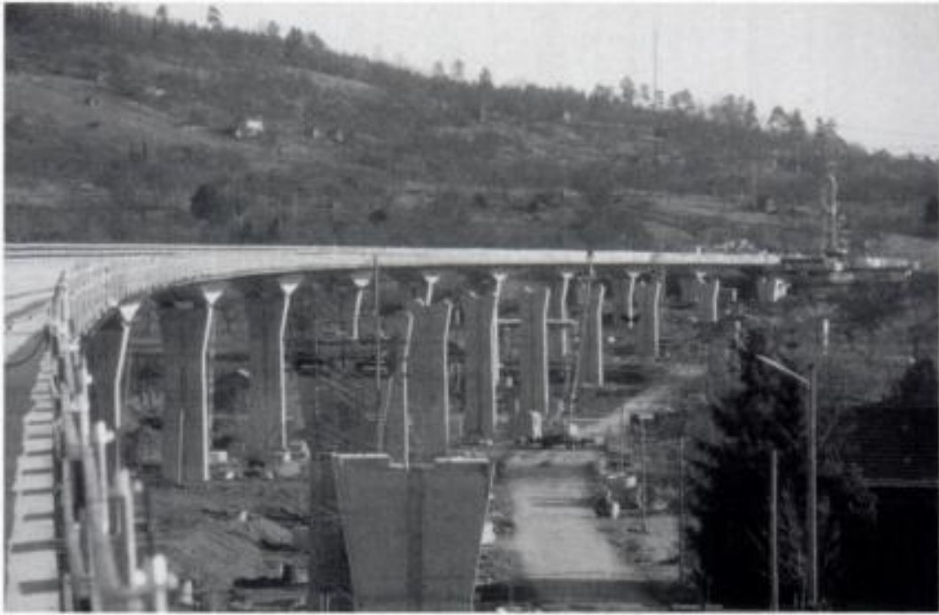
Fig. 2.39 Bridge during construction
