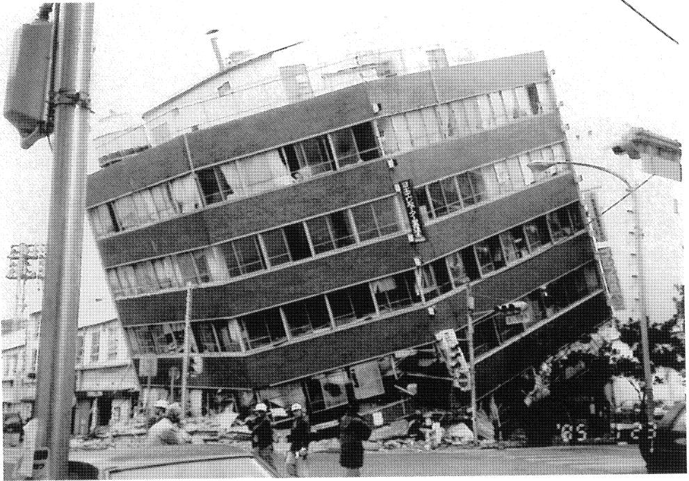
Example for the behaviour of buildings with reinforced concrete columns under the South Hyogo Earthquake of January 17, 1995 in Japan. The building collapsed up to the third storey.
