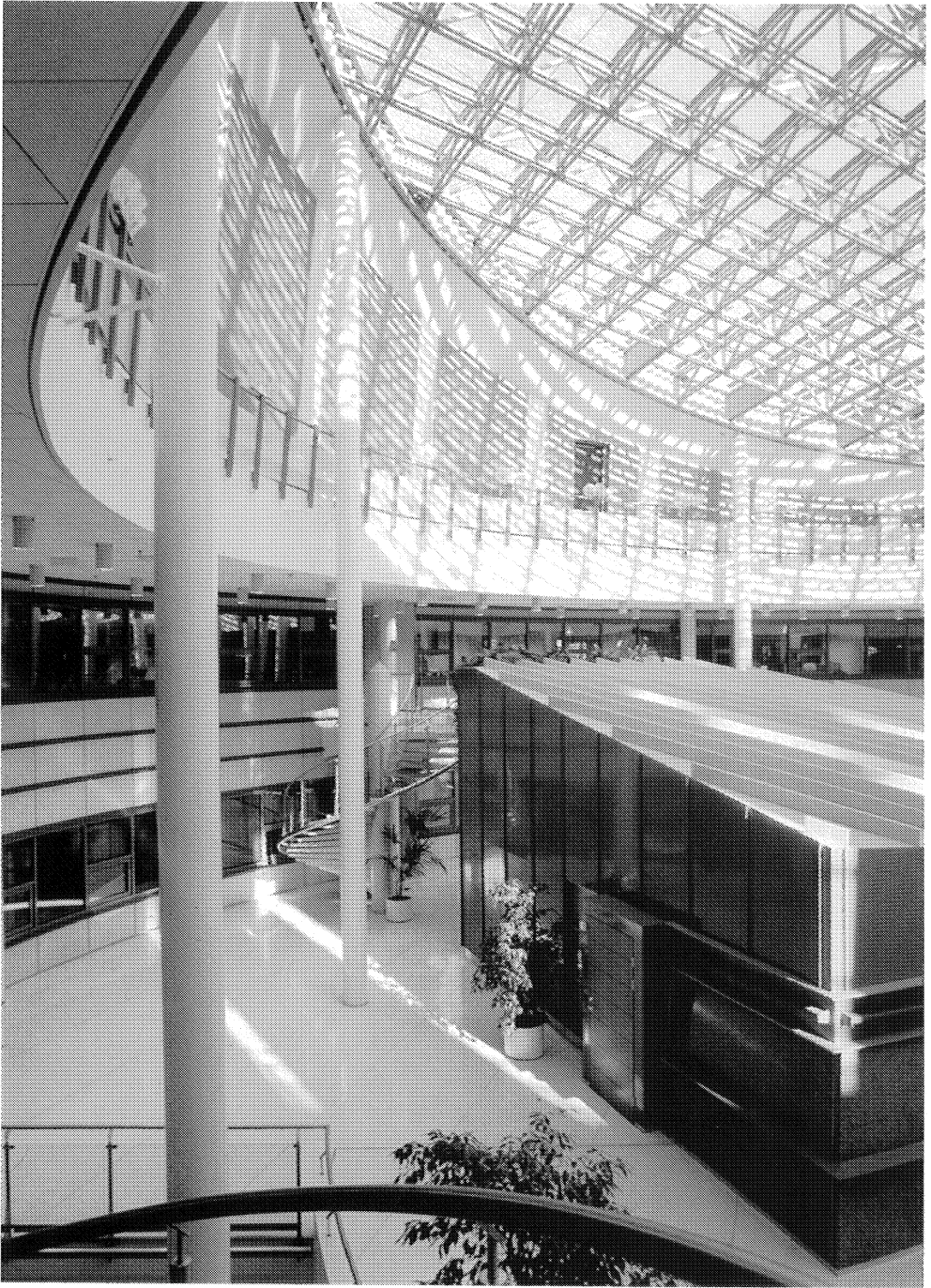
Concrete filled circular hollow section columns of the new head office building of the Finnish state oil company Neste (architect: Jauhiainen C/JN Ky). Under erection the loads were borne by the pure steel structure and after concreting the dead loads were borne, so that extremely short erection time was required.
