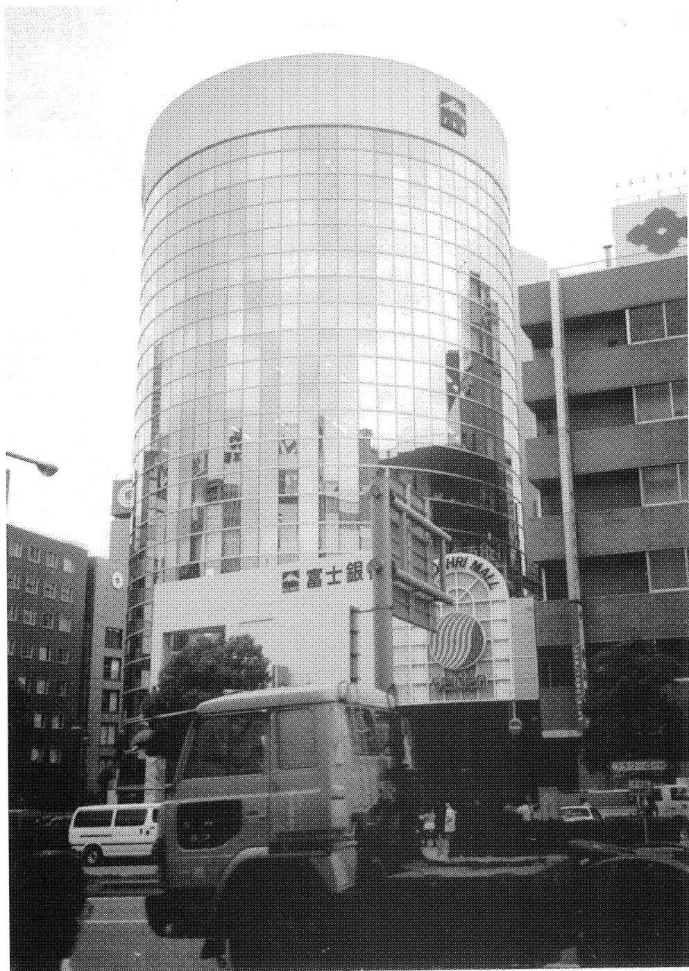
Branch bank office building in the central area of Kobe after the South Hyogo Earthquake of January 17, 1995 in Japan. Concrete filled hollow section columns were used for the peripheral columns. Although this building stands near the centre of the earthquake, it was not damaged. This and four other buildings with those columns demonstrate the superior resistance of concrete filled hollow section columns to earthquake.
