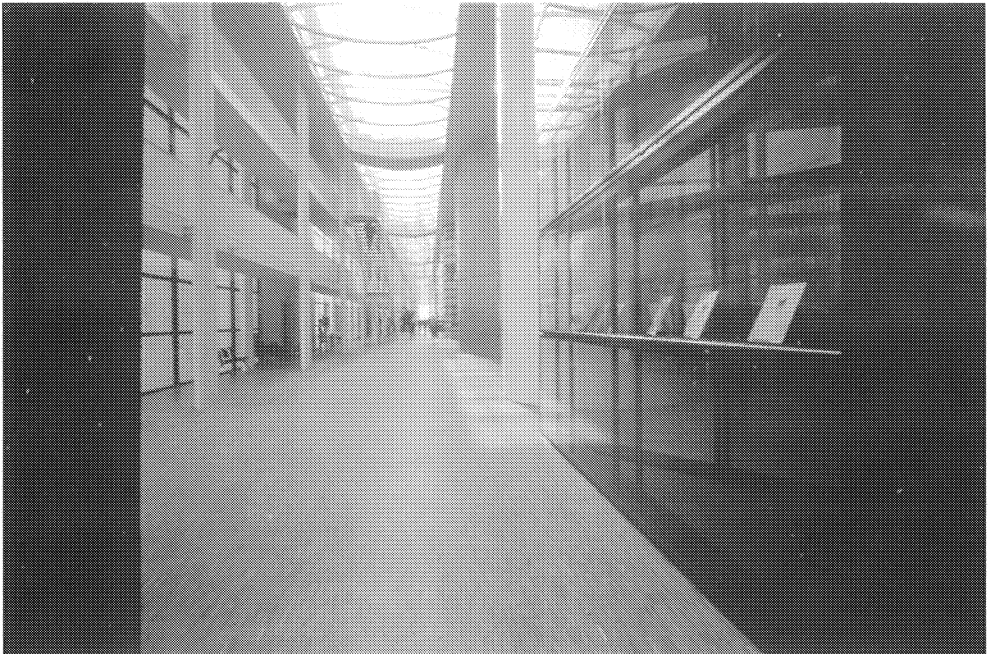
Higher school of electronics, electricity and computer science in Marne la Vallée, France (architect: Perrault). Circular concrete filled hollow section columns with 273 mm and 323.9 mm diameters.
