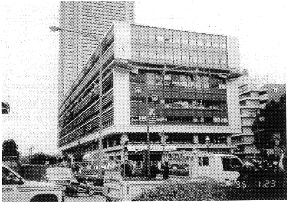
Typical collapse of a building with reinforced concrete columns in the South Hyogo Earthquake in Japan. One mid-story is totally destroyed.
