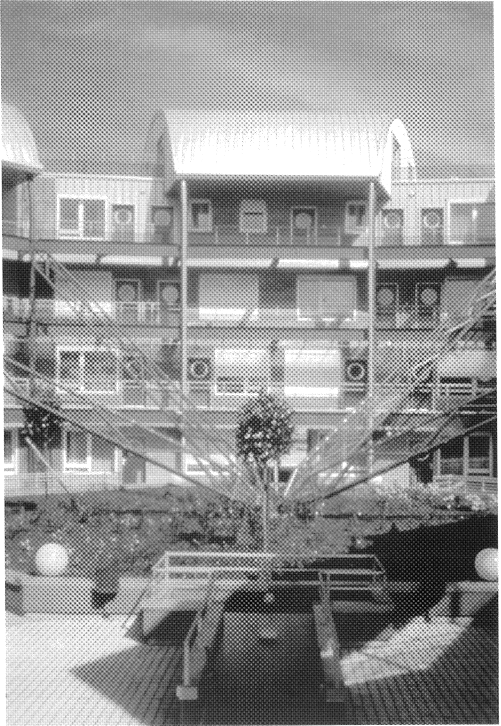
Residential building in Nantes, France (architects: Dubosc and Landowski). Concrete filled square hollow section columns with 200 mm width.
