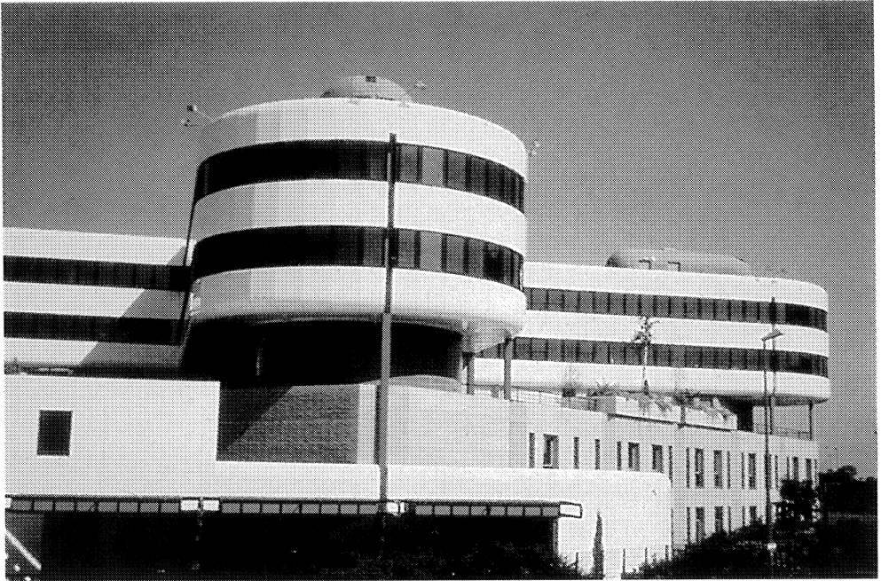
Office building in Toulouse, France (architects: Starkier und Gaisne). Concrete filled square hollow section columns with 250 mm and 300 mm widths.
