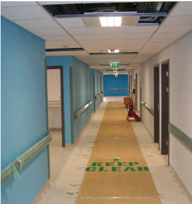
Figure 8.2 Keeping corridors clear during refurbishment
