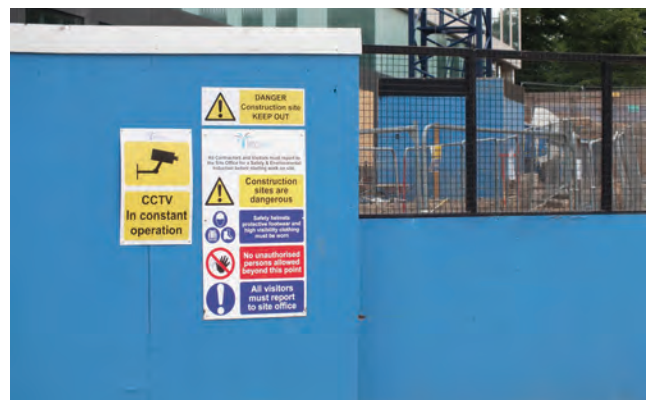
Figure 1.18 Rules at site entrance with viewing panel to see inside the site
