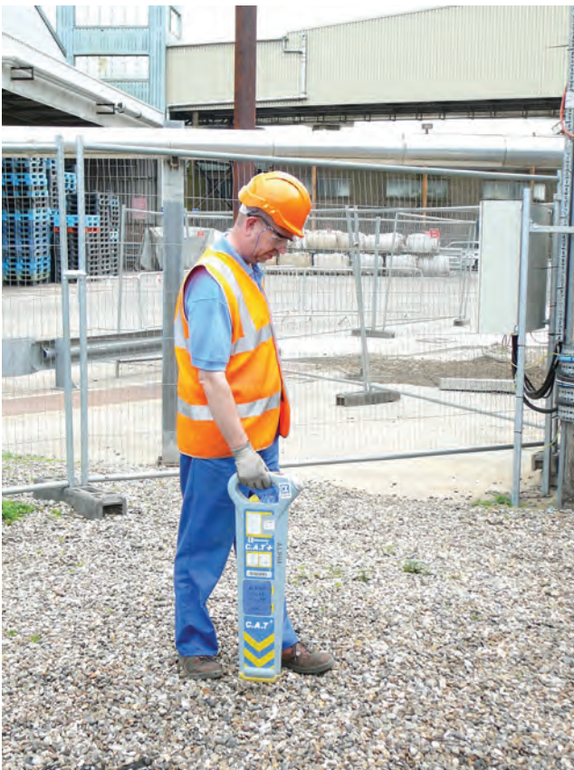
Figure 17.11 Using a cable detector
