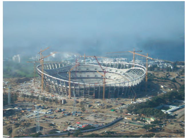
Figure 20.1 World Cup stadium under construction, Cape Town, 2009
