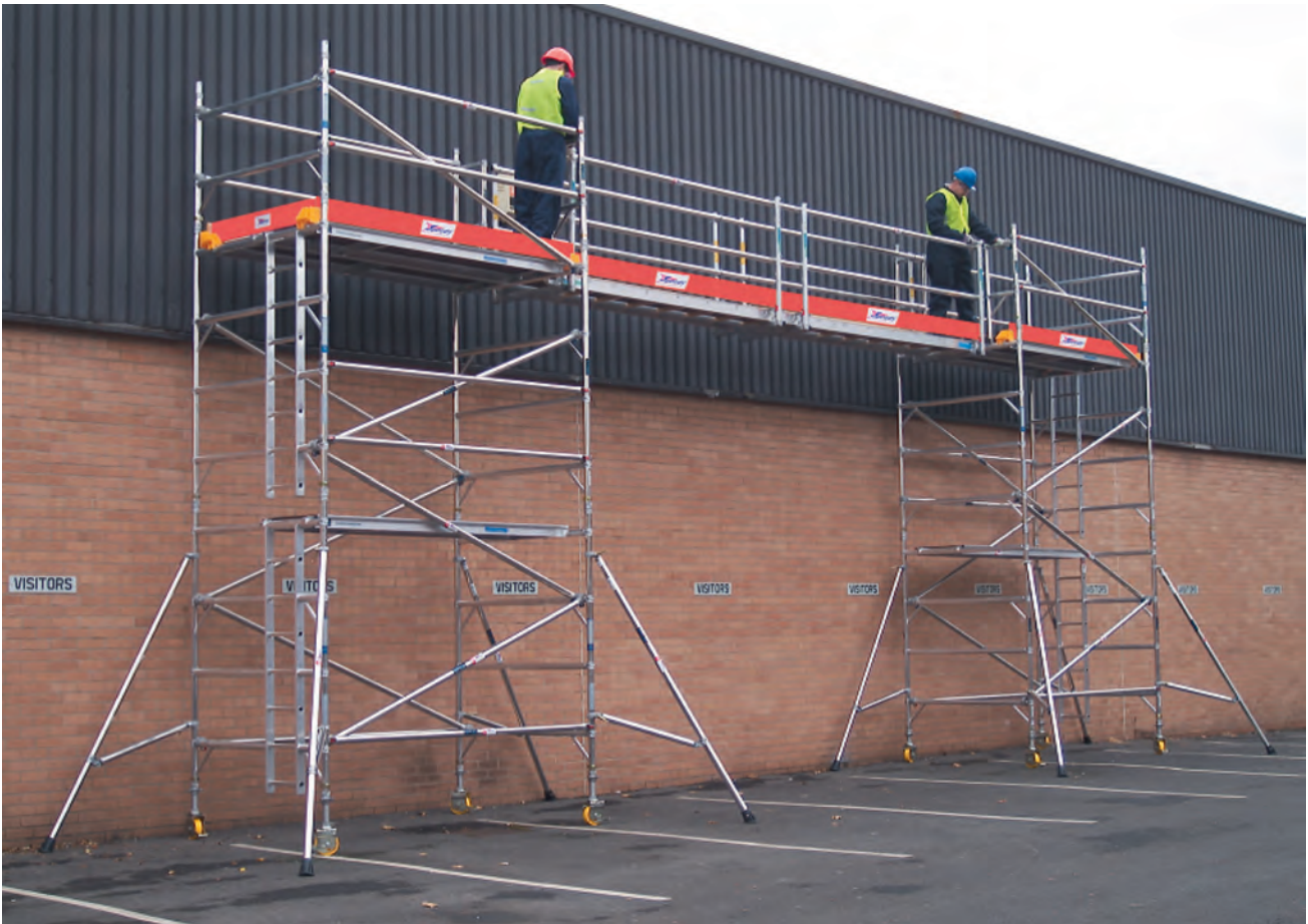
Figure 16.2 Working platform, pre-fabricated tower scaffolds and bridging unit
