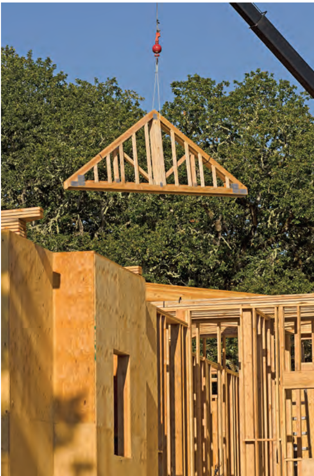
Figure 10.15 Lifting roof trusses
