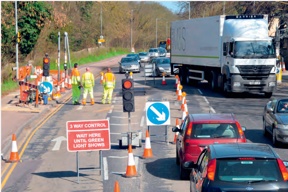
Figure 9.16 Traffic control by portable traffic signals
