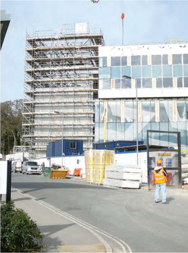
Figure 8.6 Working in or close to occupied premises
