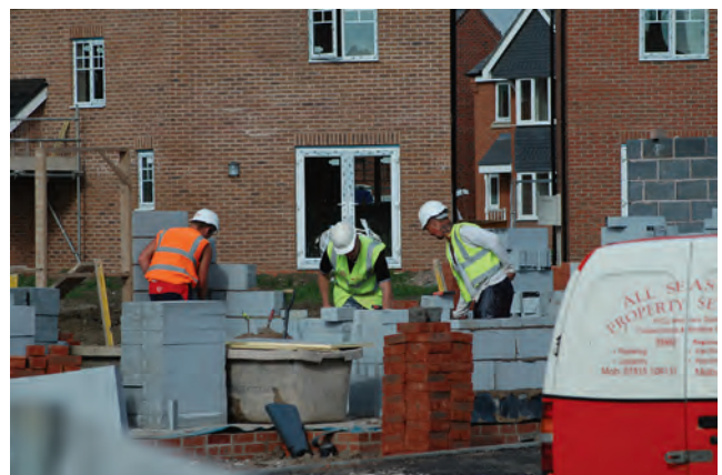
Figure 7.8 Contractors at work
