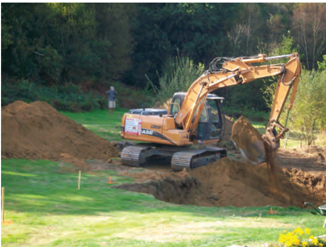
Figure 20.3 Excavator at work in France
