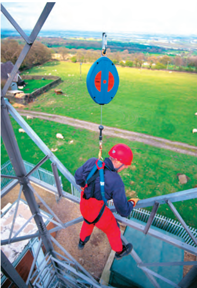
Figure 16.19 Fall arrest harness and device
