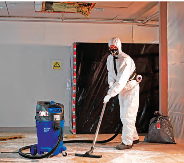
Figure 18.2 High hazard vacuum cleaner to clear up asbestos material
