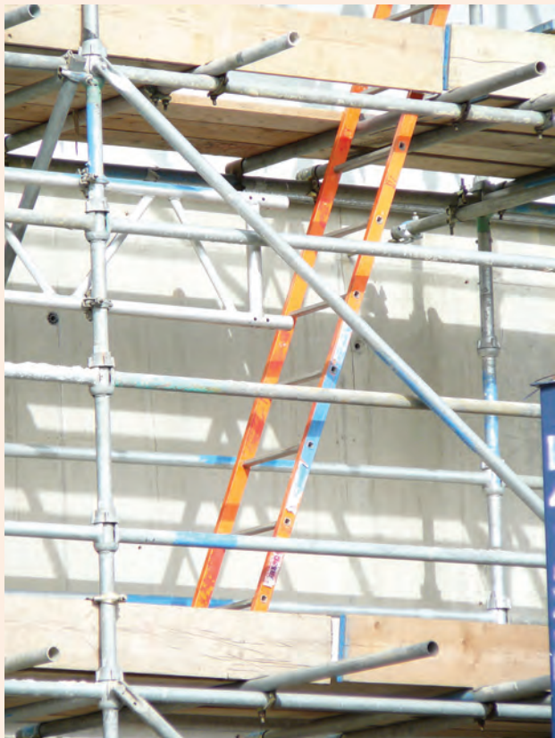
Figure 2.10 Ladders and scaffold maintained in good condition and frequently inspected
