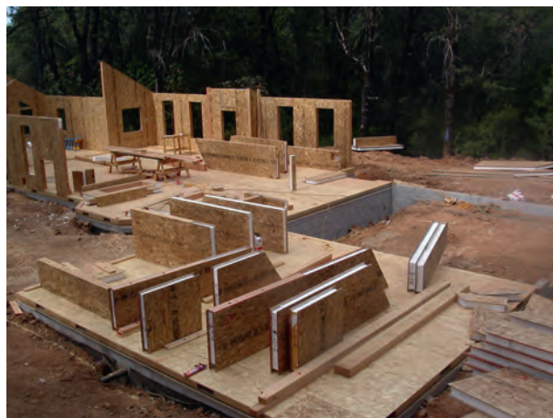
Figure 13.18 Insulated core panels
