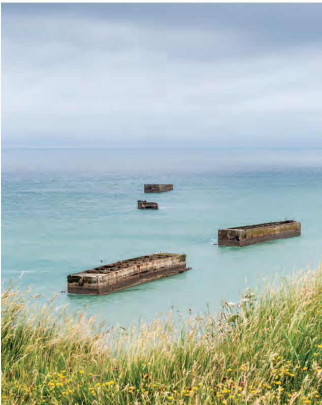
Figure 17.5 (a) Massive Second World War concrete caissons known as mulberry harbour units – hundreds were constructed in the UK and then towed to Normandy and sunk in position to form a harbour wall
