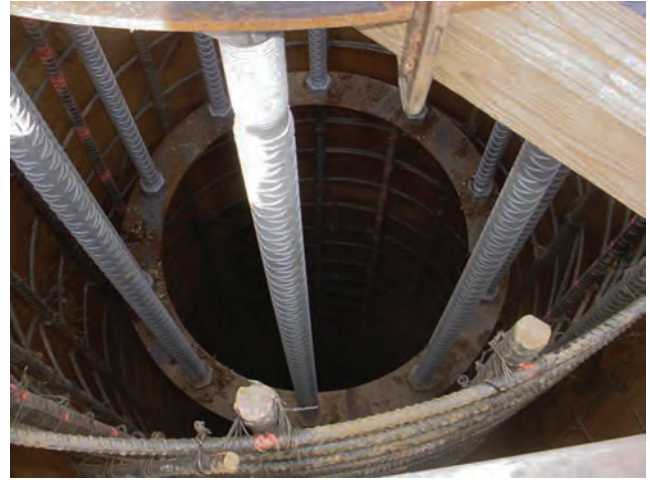
Figure 17.5 (b) Steel caisson being used in construction work
