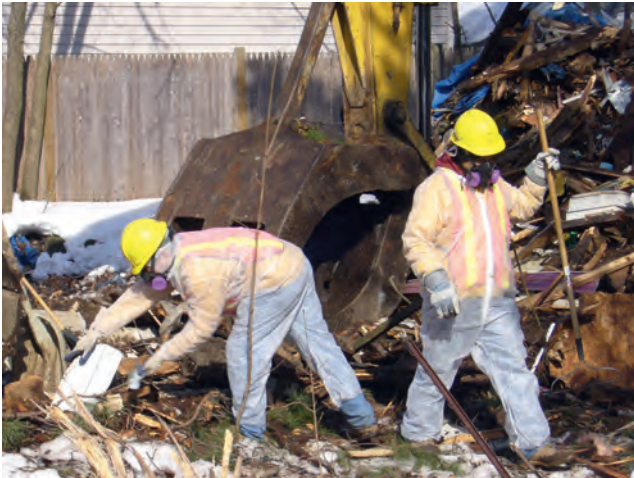
Figure 18.7 Clearing up asbestos-containing materials (hazardous waste) after demolition has started is very difficult and expensive
