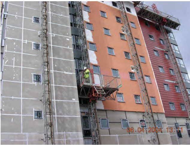
Figure 16.1 Working at height – mast climbing work platforms
