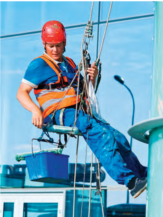
Figure 8.13 Cleaning must be done carefully to prevent slipping or falling using bosun's chair and rope support with trained worker
