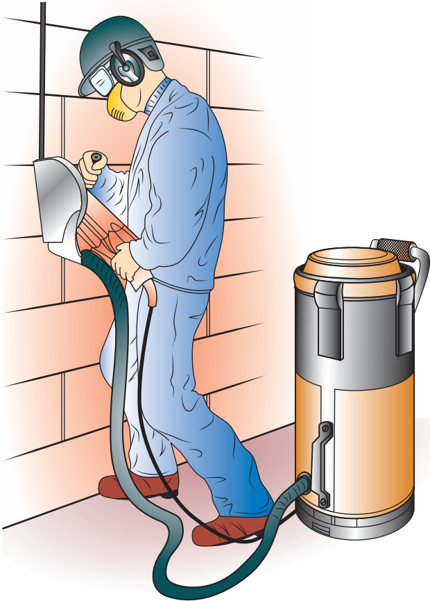
Figure 4.19 Good dust control for a chasing operation. A dust mask is still required for complete protection
