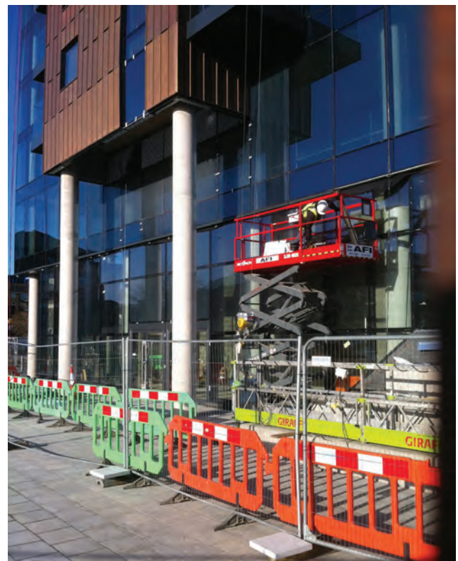
Figure 16.16 Mobile elevating work platform (MEWP) – scissor lift
