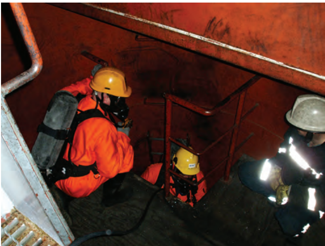
Figure 17.12 Entering a confined space with full breathing apparatus and watcher outside
