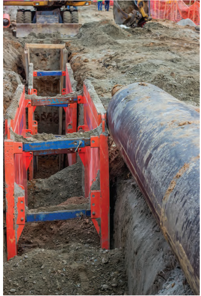
Figure 17.10 Trench box in use
