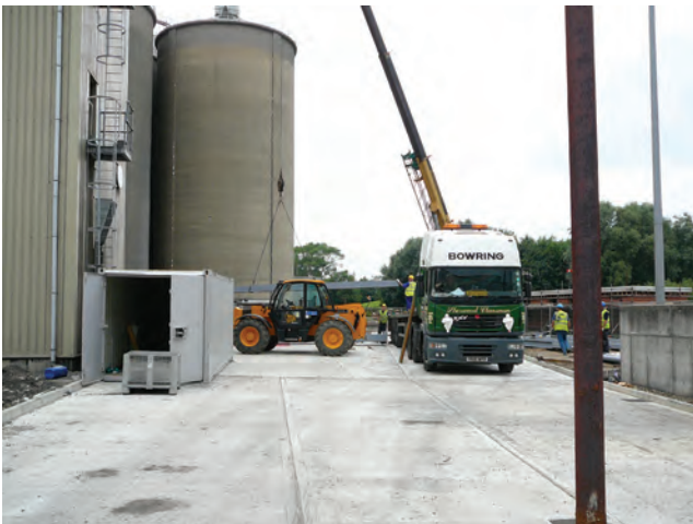
Figure 1.16 Contractors at work unloading steel beams
