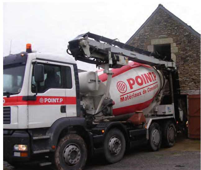
Figure 9.13 Concrete delivery by road
