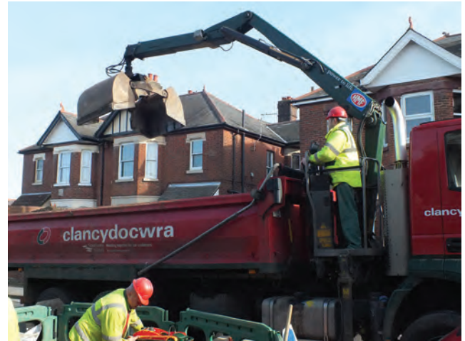
Figure 14.20 Removing waste from a roadside excavation by lorry-mounted loading grab
