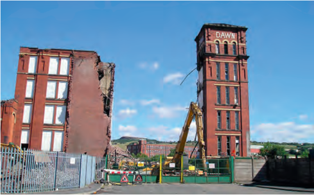
Figure 18.1 Demolition of old mill in progress
