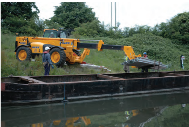
Figure 10.1 Loading pipes onto a barge using a teleporter lift truck
