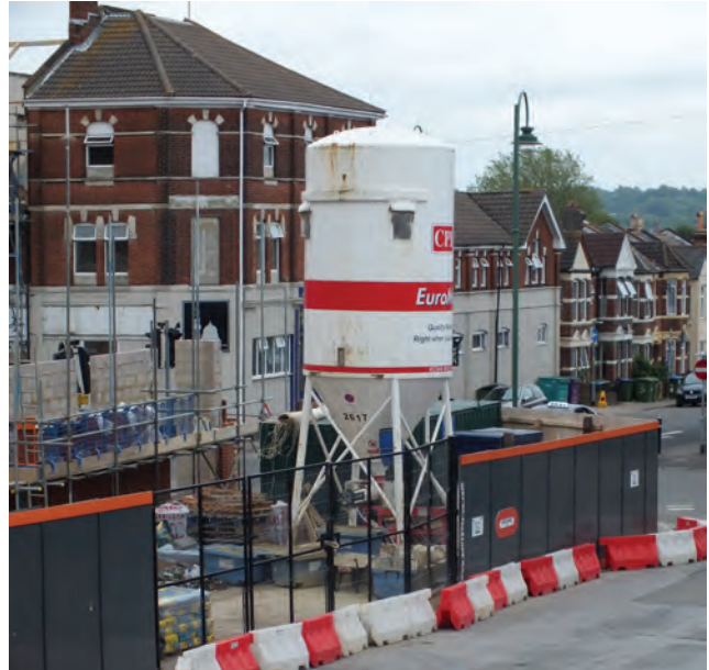
Figure 22.4 Large cement silo on a construction site
