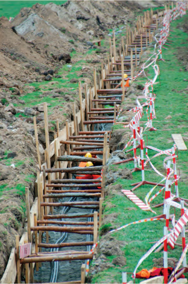
Figure 17.9 (b) A long timbered trench in soft ground
