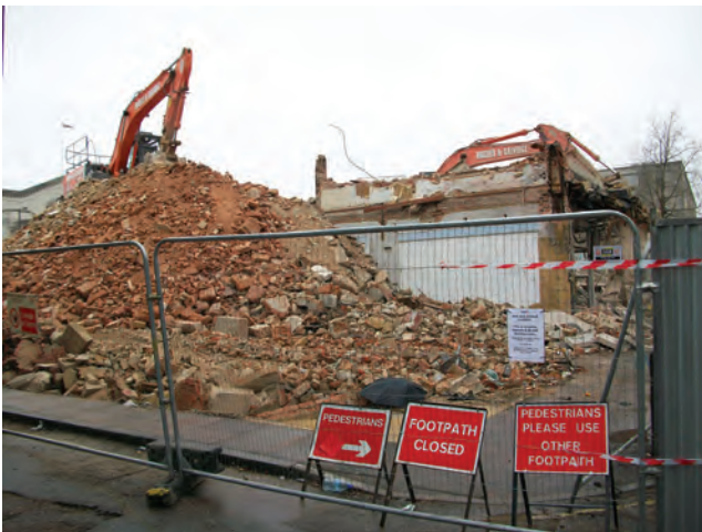
Figure 7.2 Demolition and ground clearance
