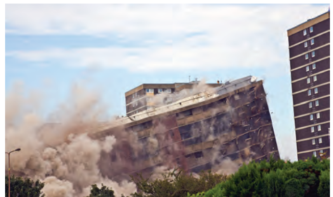
Figure 18.5 Controlled collapse
