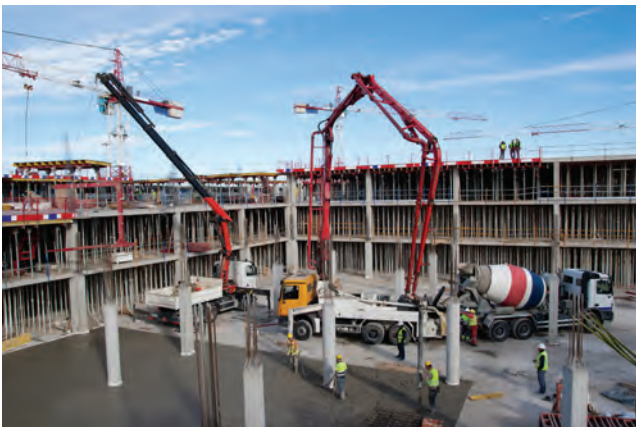
Figure 8.1 Concrete being pumped to upper floors on a large construction site
