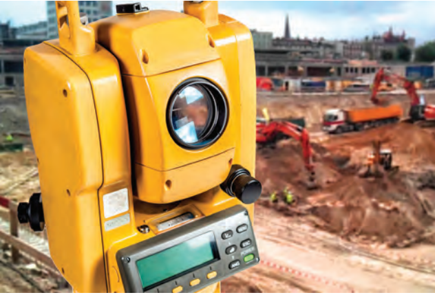
Figure 15.12 Low level laser beams extensively used for levelling and setting out in construction work
