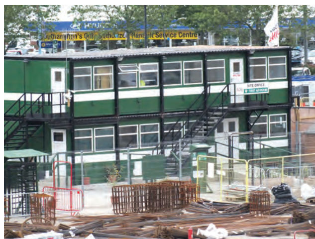
Figure 13.16 Multiple temporary accommodation units (TAUs) with external staircase
