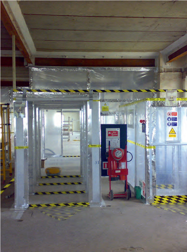
Figure 14.18 Asbestos removal enclosure
