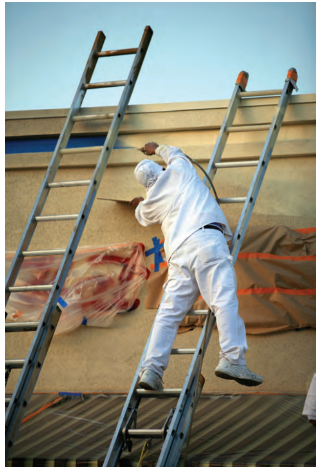
Figure 2.8 The policy might be good but is it put into practice – unsafe use of a ladder
