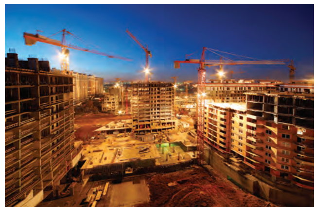
Figure 8.8 A large building site well lit at night
