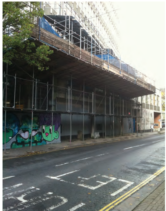
Figure 16.13 Fan scaffold to protect people and passing traffic
