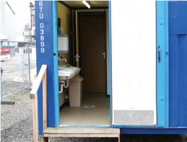
Figure 4.18 Welfare washing facilities: washbasin should be large enough for people to wash their forearms
