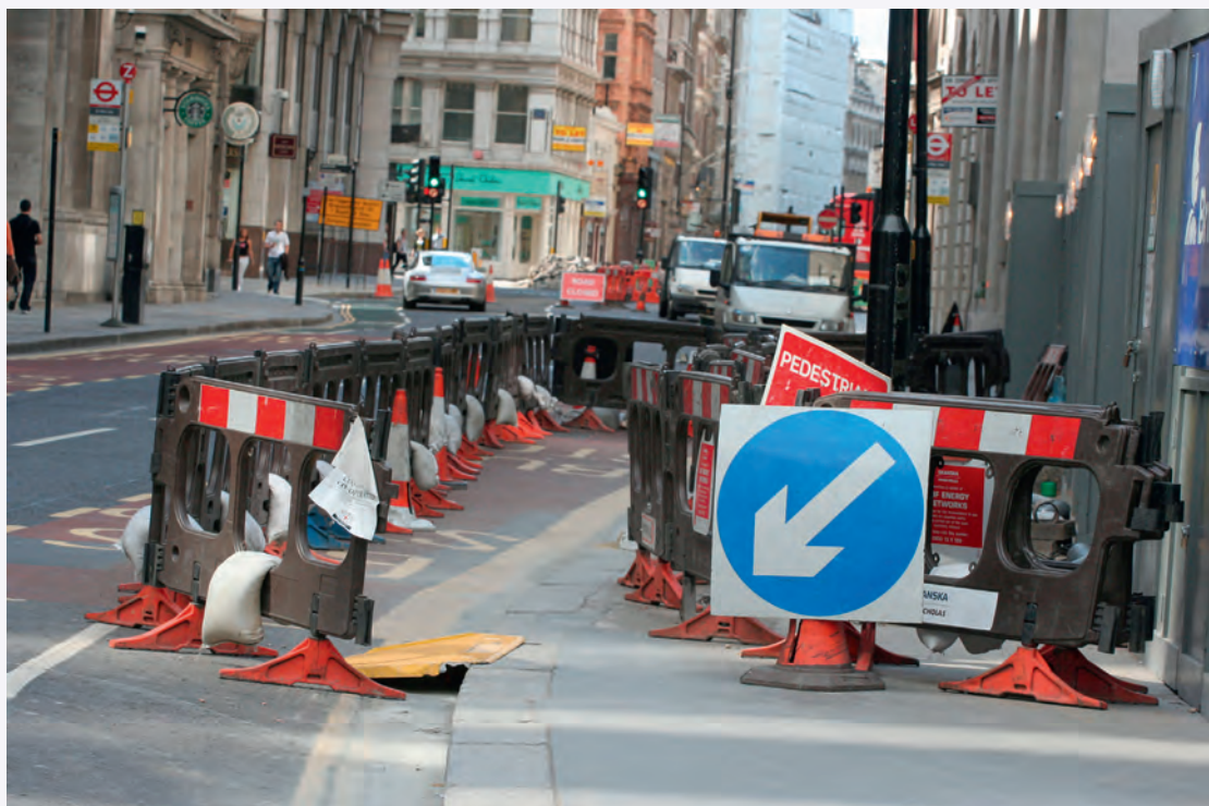
Figure 9.17 Works on footway with temporary footway in carriage
