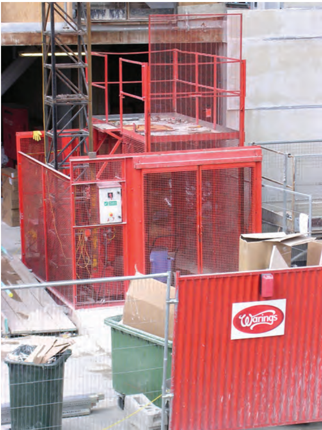
Figure 16.14 Hoist with interlocked gates
