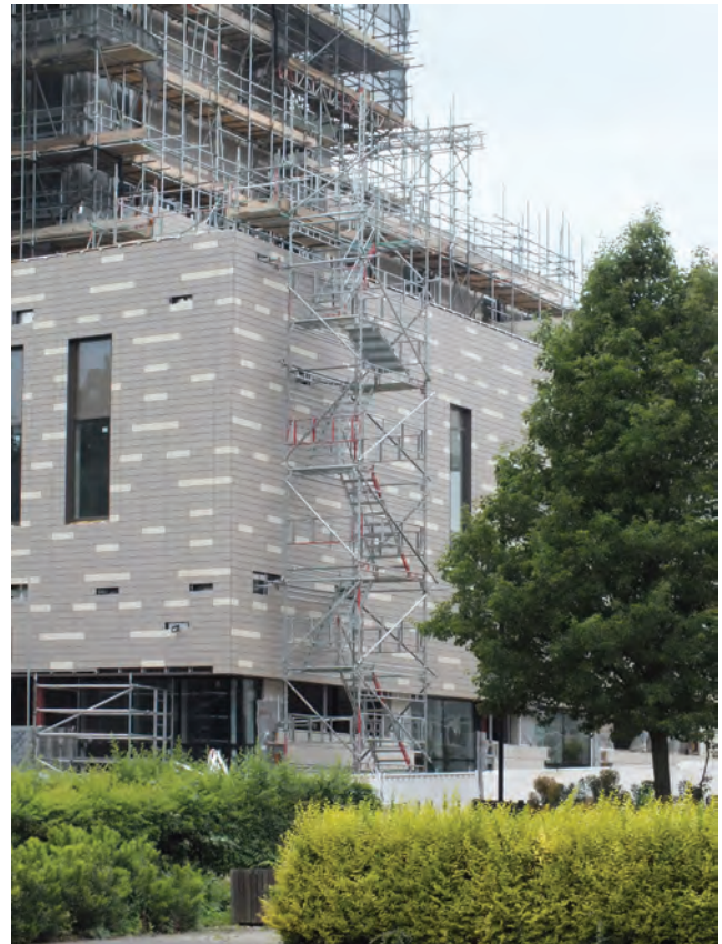
Figure 13.27 External access/fire escape in a large scaffold during building construction
