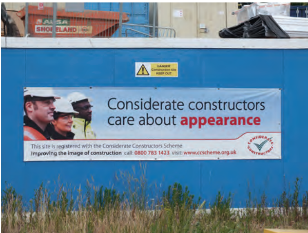
Figure 7.9 Barriers to prevent unauthorised entry – also advertising involvement with the Considerate Constructors Scheme
