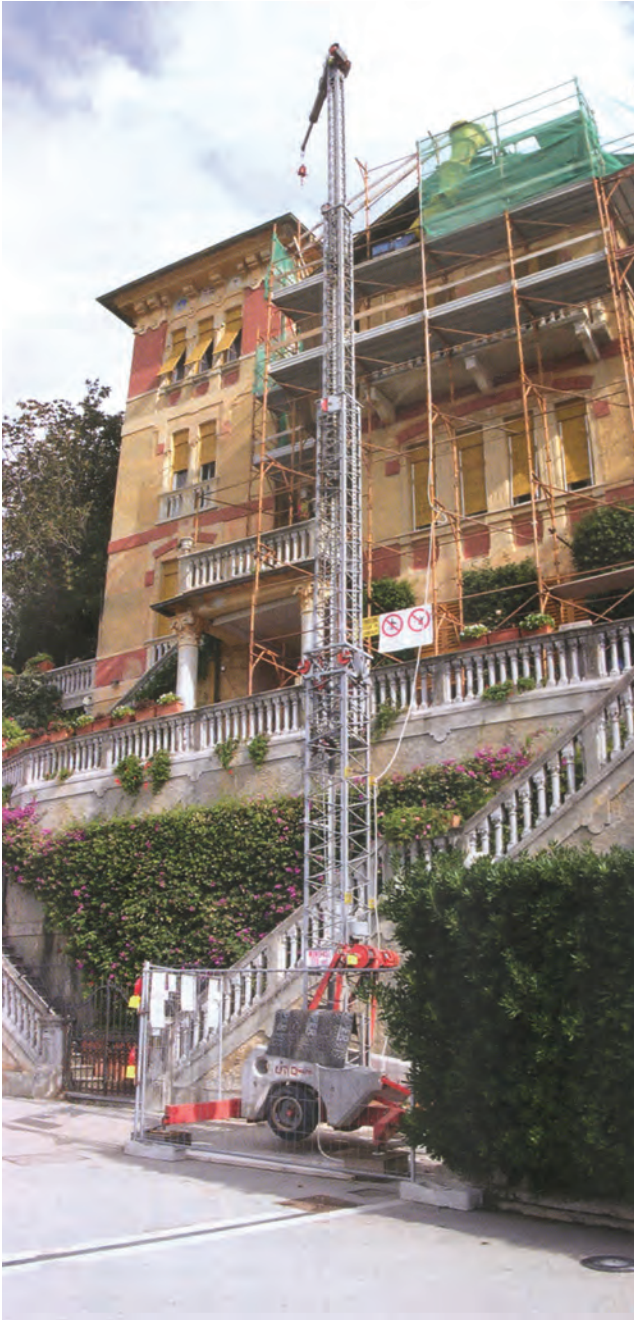
Figure 10.17 Mobile self-erecting tower crane
