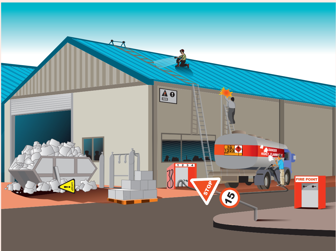
Figure 5.15 Roof repair and unloading flammable liquids
