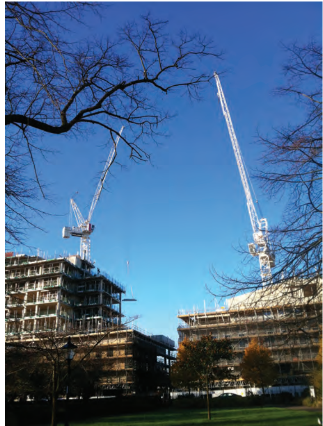
Figure 1.1 At work in Southampton 2015 – site operated well into the night
