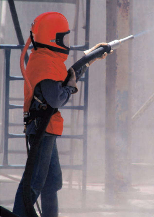
Figure 4.21 A lone worker – special arrangements required. Sand or shot blasting inside a tank with an air-fed helmet and vest
