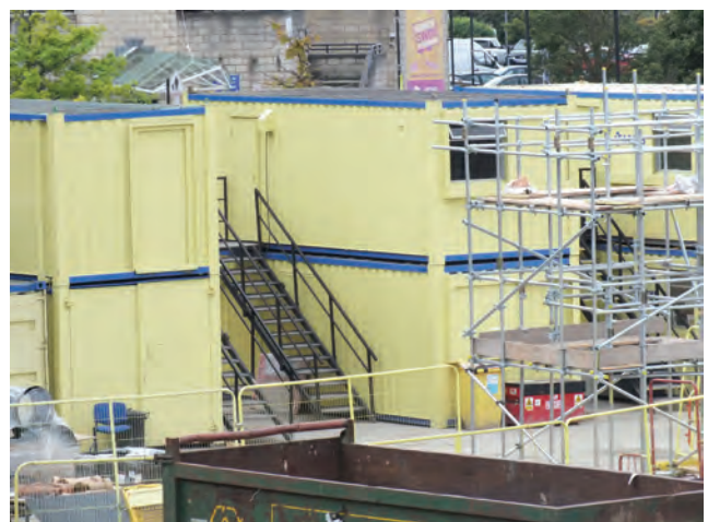
Figure 8.15 Good stairs with handrail leading from site accommodation
