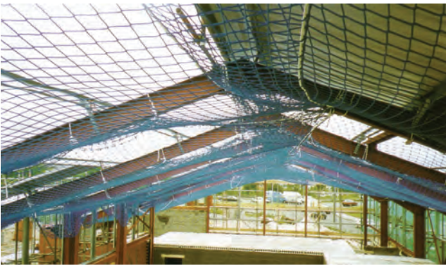
Figure 16.3 Industrial roof work with safety nets to arrest falls
