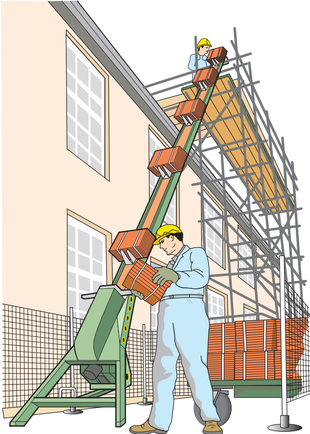
Figure 10.12 A brick elevator
