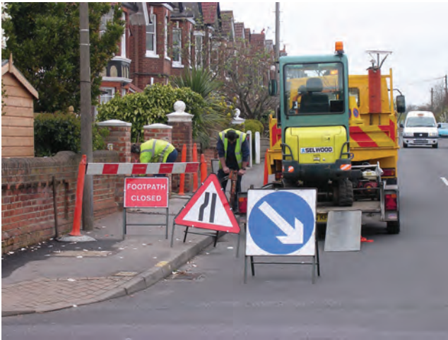
Figure 9.9 Road works sign for footpath closure. Could be improved with walkway for pedestrians beside track. But this is only minor road, and pedestrians can cross to a good pavement opposite
