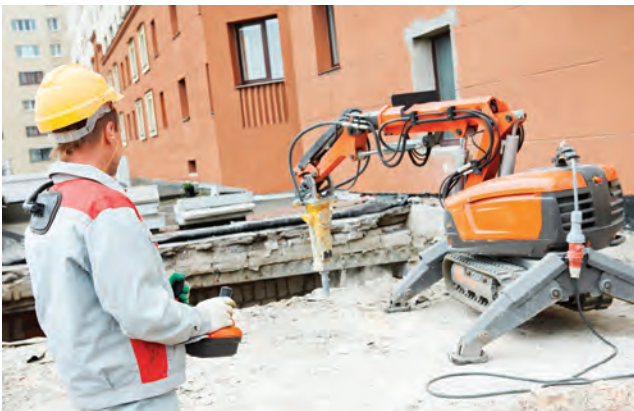
Figure 18.4 Remote-controlled hydraulic arm for pushing, nibbling or hammering
