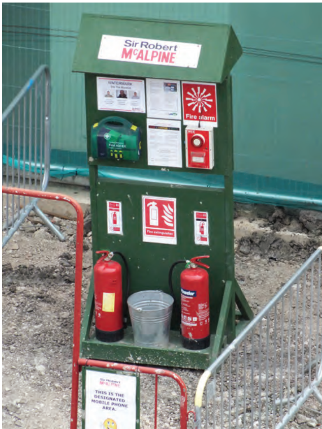
Figure 13.23 Fire point on large construction site
