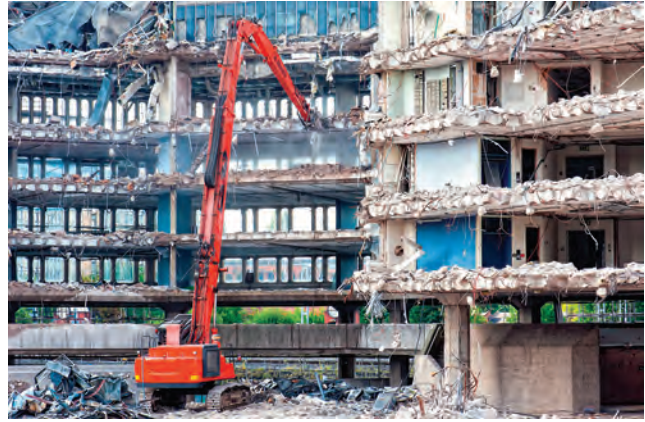
Figure 18.3 Long-reach hydraulic arm for piecemeal demolition
