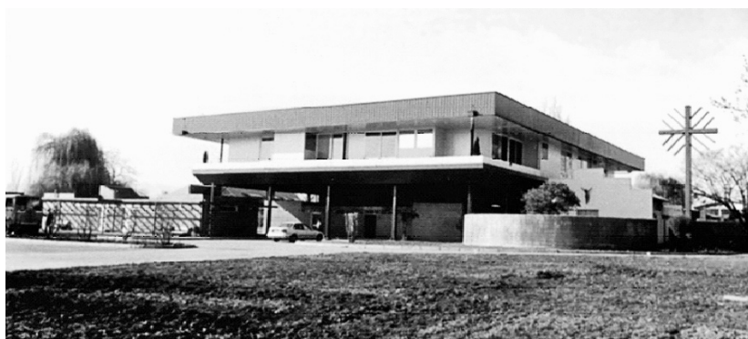
1.8 The Clinica Familia Hospice and Center for Palliative Care, Santiago, Chile, is located on the grounds of a medical center campus. The roof's deep overhangs provide shade for the inpatient bedrooms on the second level
