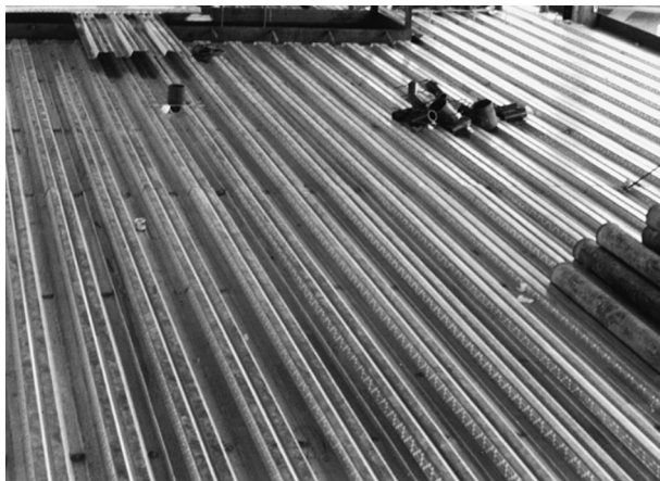
FIGURE 8.45 Flooring installed during steel erection
