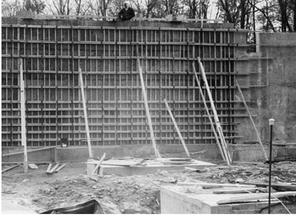
FIGURE 7.14 Formwork for cast-in-place concrete
