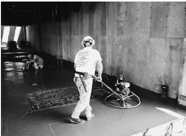
FIGURE 7.12 Worker using a powered trowel
