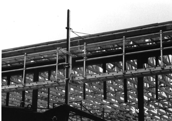
FIGURE 8.38 Pump jack scaffold
