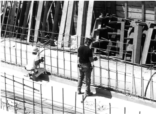
FIGURE 11.14 Construction workers tying rebar
