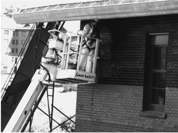
FIGURE 7.2 Aerial lift with worker wearing a safety harness
