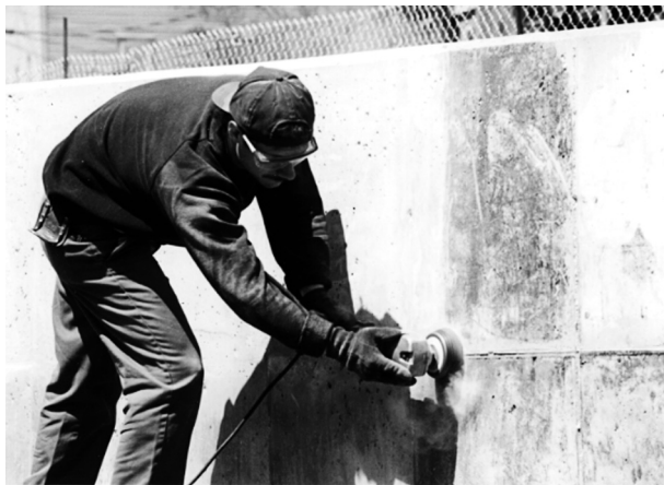
FIGURE 9.17 Dust containing silica is generated by concrete finishing
