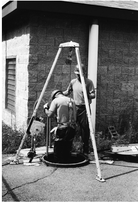
FIGURE 7.18 Confined space worker retrieval system with attendant
