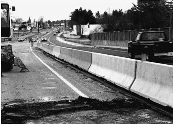
FIGURE 7.5 The use of jersey barriers as barricades
