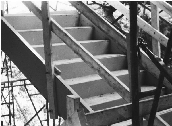
FIGURE 8.42 Stair pans filled with wood
