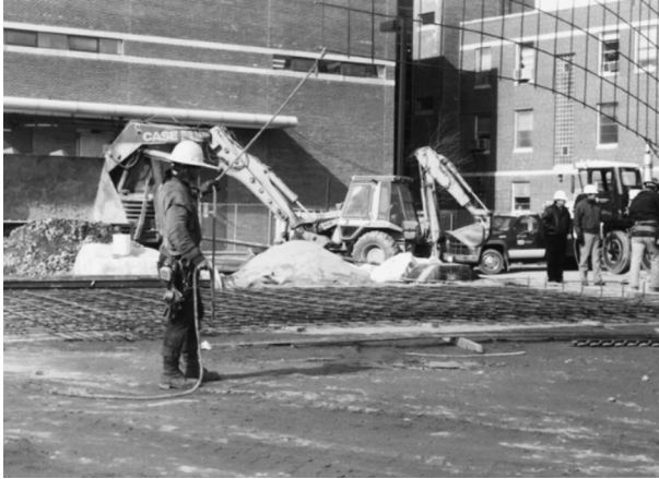
FIGURE 8.18 Worker using a tagline to direct a load
