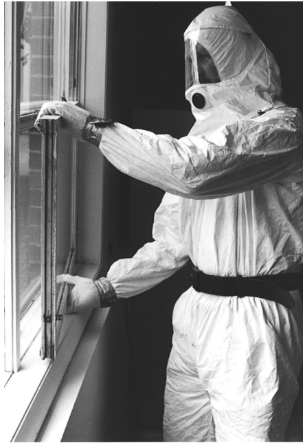
FIGURE 10.24 Powered air-purifying respirator used by a window contractor for potential lead dust exposure
