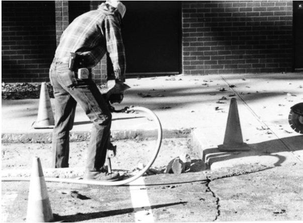
FIGURE 11.11 Worker using a pneumatic jack hammer
