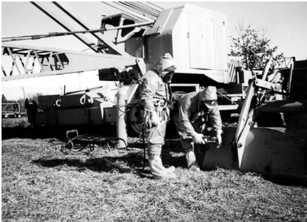
FIGURE 10.18 Chemical permeation must be considered for hazardous waste work. Courtesy of the Operating Engineers, Local #478, Meriden, CT
