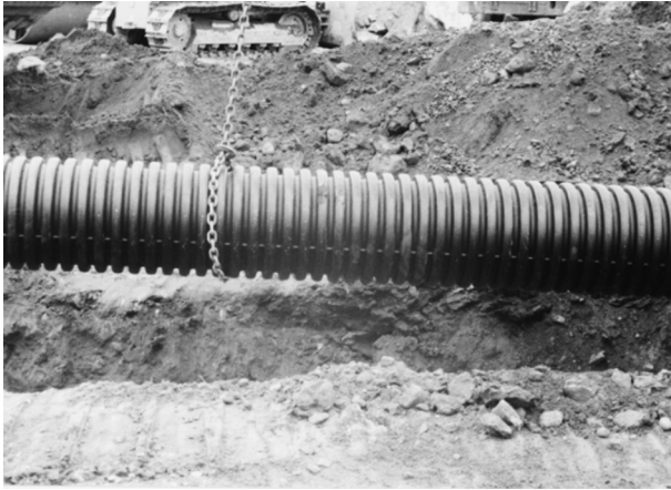
FIGURE 8.23 Chain using a choker hitch for lifting
