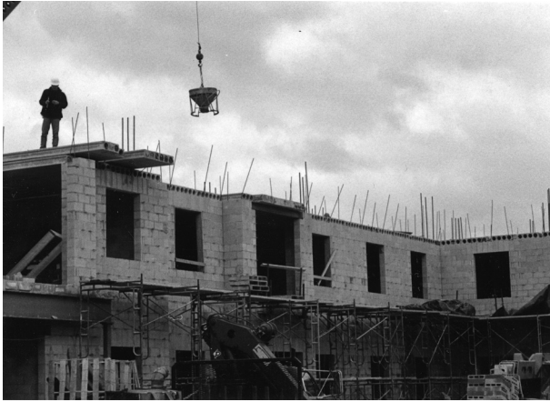
FIGURE 7.11 Concrete bucket in use on construction site
