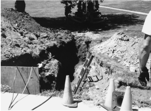
FIGURE 7.36 An open excavation with a ladder for egress
