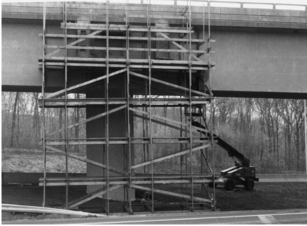
FIGURE 8.36 Example of a pole scaffold
