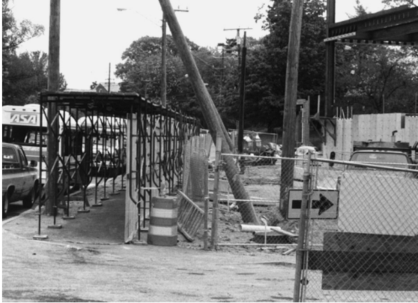
FIGURE 7.45 Canopy for overhead protection
