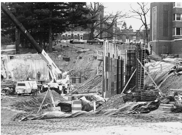
FIGURE 1.7 The always changing construction site
