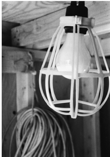
FIGURE 7.30 Protected temporary lighting
