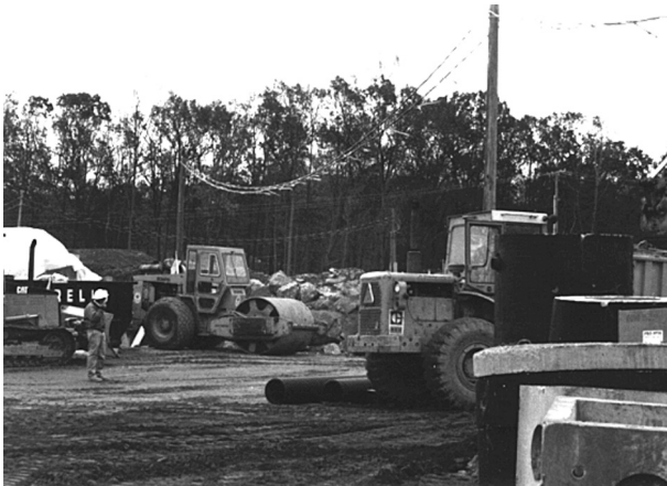
FIGURE 7.28 Conductors over a typical construction site
