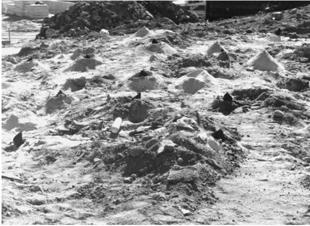
FIGURE 7.42 Drilled blasting area ready for loading
