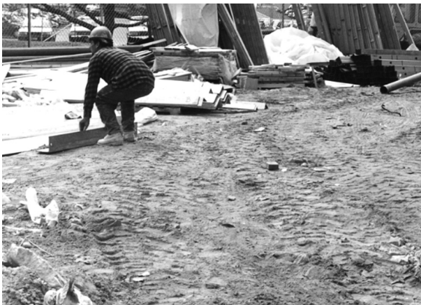
FIGURE 11.2 Laborer setting down a load using his legs
