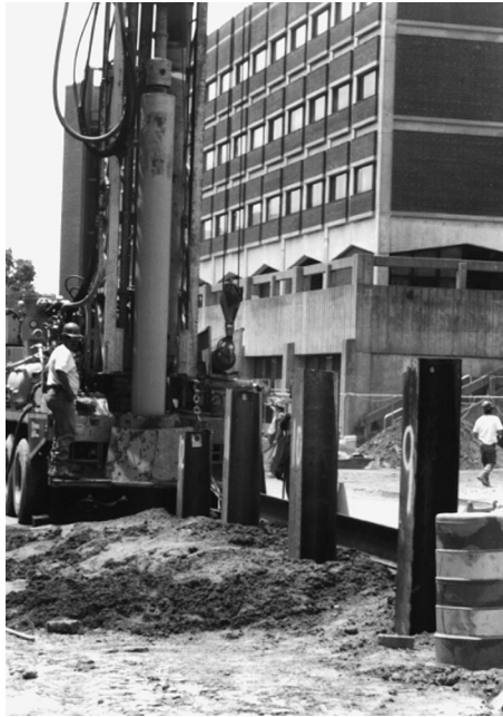
FIGURE 8.12 Example of piles being driven
