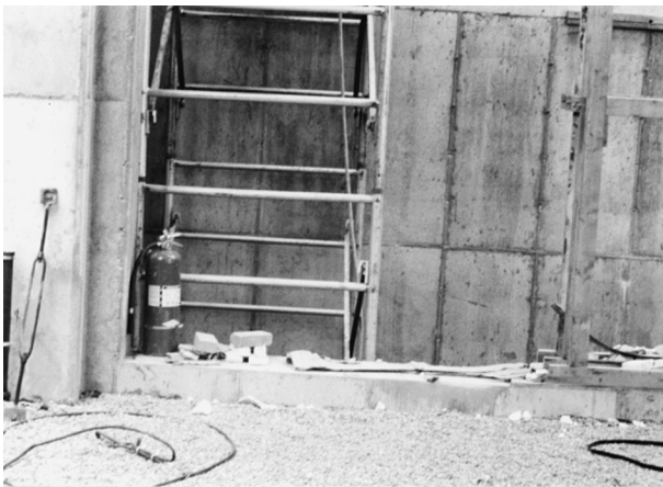
FIGURE 7.52 Typical fire extinguisher on a construction site
