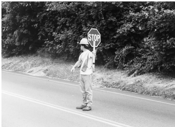
FIGURE 7.54 A flagperson directing traffic flow
