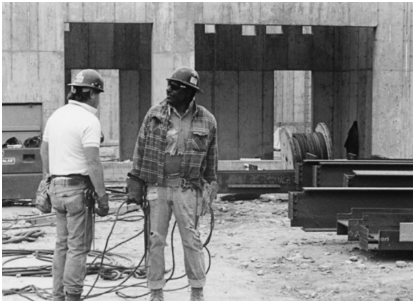
FIGURE 1.5 Ironworkers preparing to rig
