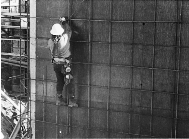
FIGURE 1.1 Ironworker tying rebar on a lattice
