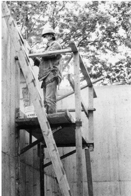
FIGURE 8.33 A full planked scaffold with guardrails
