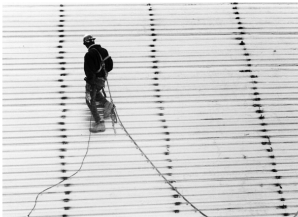
FIGURE 11.16 Roofer working on slanted surface
