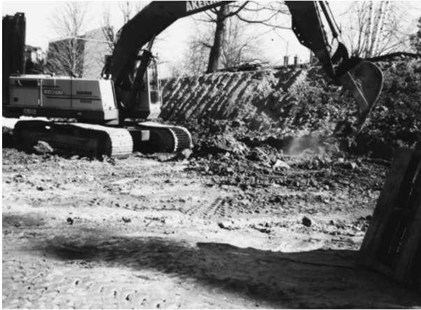
FIGURE 7.37 Example of sloping and excavation
