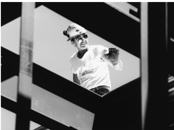
FIGURE 9.2 The construction site is constantly changing
