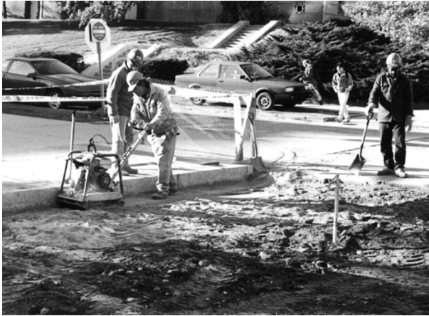
FIGURE 11.10 Example of a vibrating tamping tool
