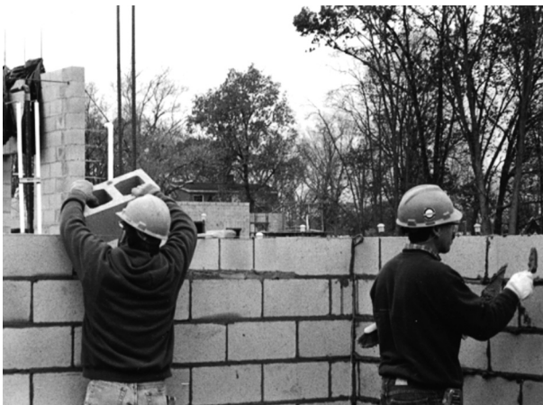
FIGURE 11.8 Mason laying block above shoulder height
