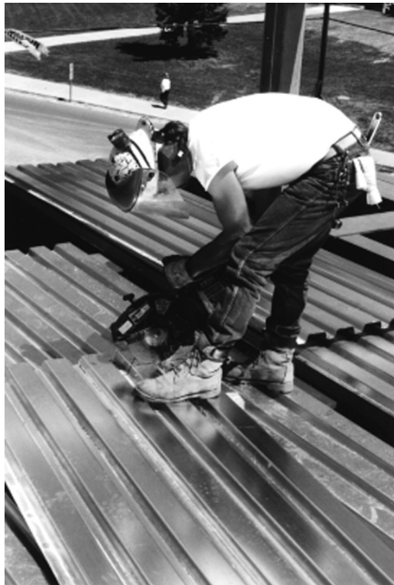
FIGURE 9.4 Saws are normally generators of high frequency noise
