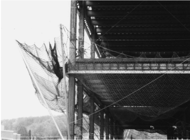
FIGURE 8.31 Perimeter safety nets in use to protect steelworkers involved in erection
