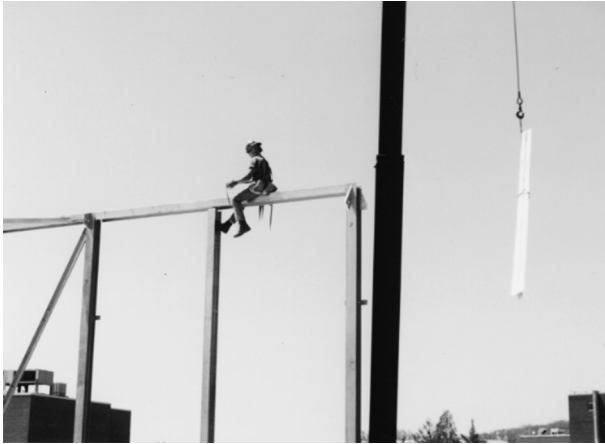
FIGURE 8.44 A steel worker's precarious perch
