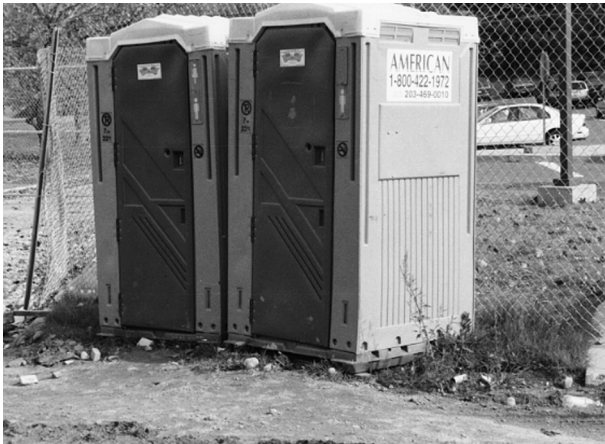
FIGURE 8.48 Typical toilets found on construction jobsites
