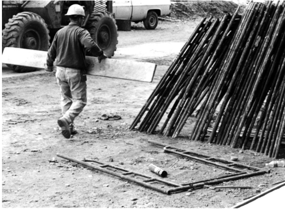
FIGURE 11.3 Carpenter carrying a board with his back straight and load close to his body
