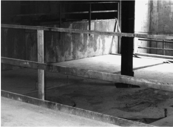
FIGURE 8.47 3½ inch toeboard on a guardrail system
