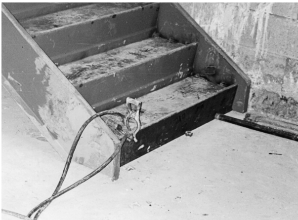
FIGURE 7.4 Grounding for an arc welder
