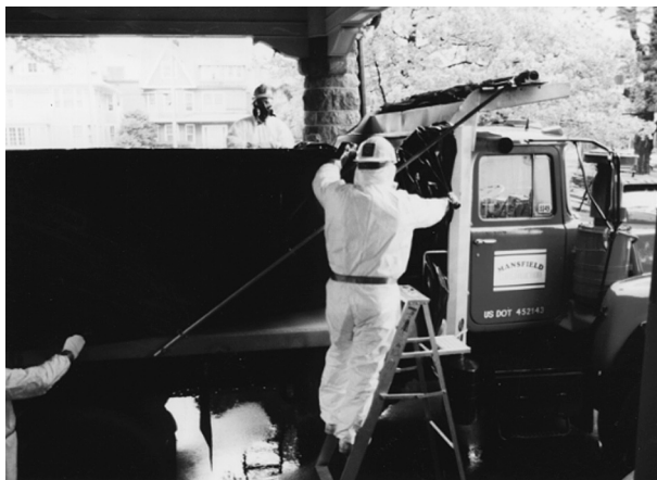
FIGURE 7.57 Trained workers doing hazardous waste work
