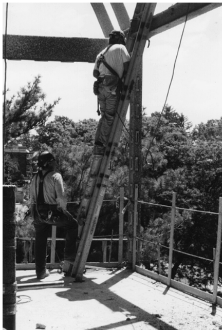
FIGURE 8.3 Safe use of an extension ladder by using an extra person to prevent displacement
