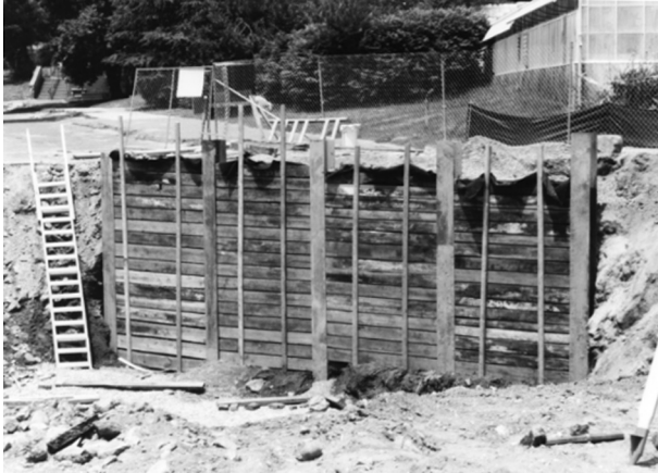
FIGURE 7.38 A timber shored wall of an excavation
