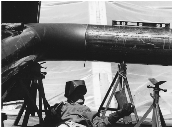
FIGURE 10.8 Eye and face protection for welding
