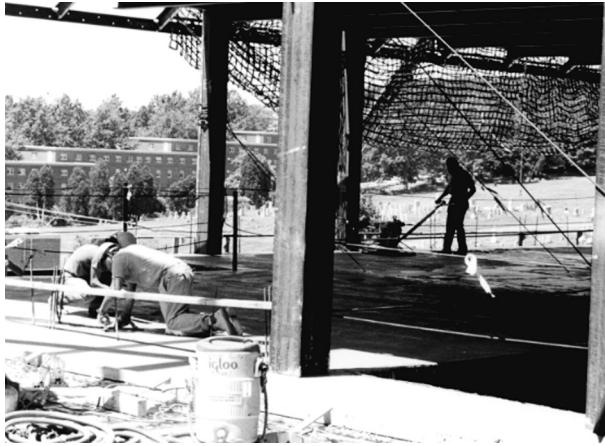
FIGURE 11.15 Workers performing hand troweling while worker in the background uses a mechanized trowel
