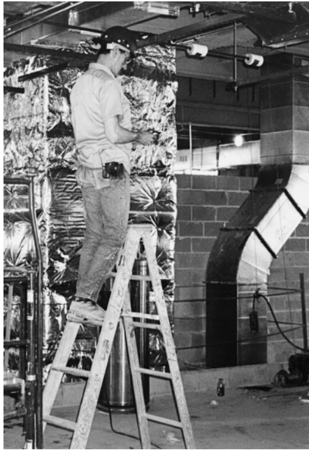
FIGURE 8.1 The safe use of a stepladder is standing no higher than the second step from the top
