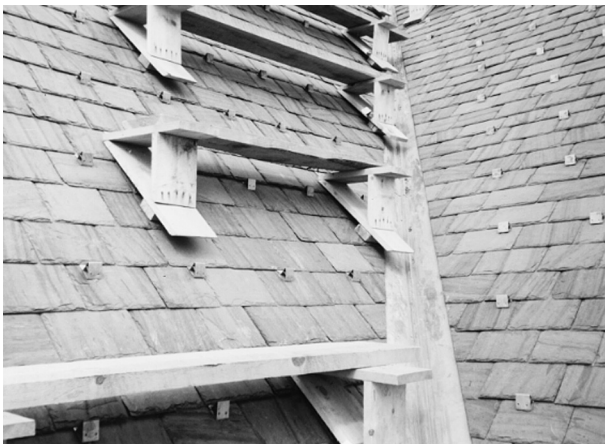
FIGURE 8.37 Example of roof bracket scaffolds
