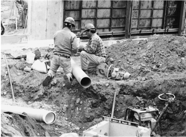
FIGURE 2.1 Typical construction workers laying pipe
