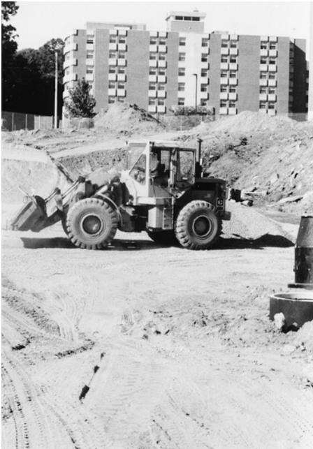
FIGURE 8.11 Front-end loaders are bidirectional and required to have a back-up alarm
