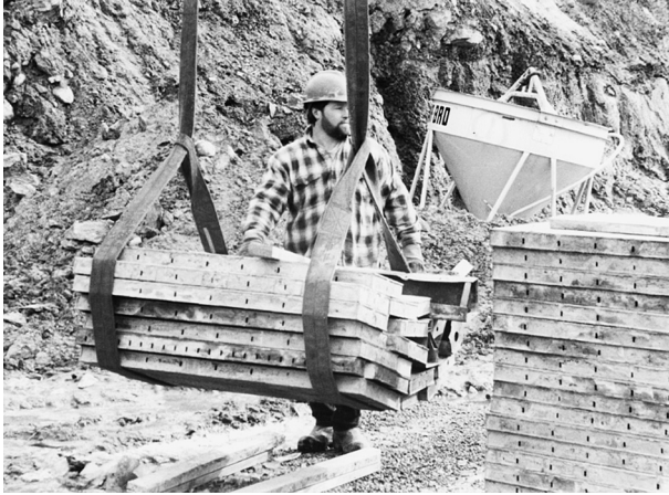
FIGURE 8.27 Web sling being used on construction site
