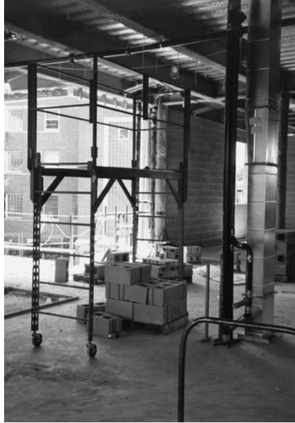
FIGURE 8.39 Example of a mobile scaffold
