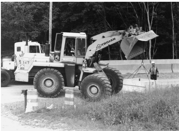
FIGURE 8.22 Using a multiple leg sling for lifting
