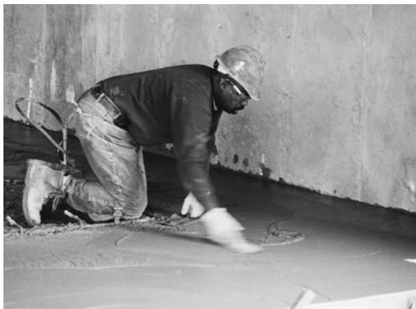
FIGURE 10.9 Protective clothing and equipment specific for the job
