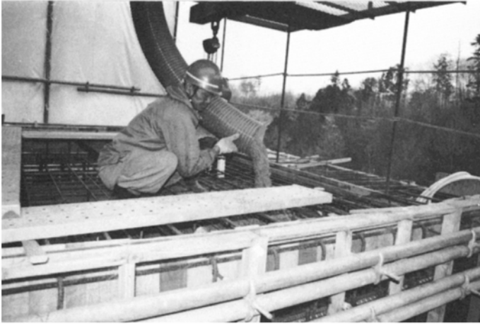
Photograph 3 Concrete placing
