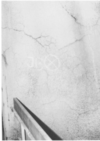
Fig. 4. Typical shrinkage cracking in shotcrete at the Jordan dam.
