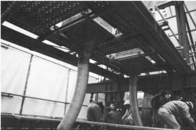
Photograph 2 Concrete placing apparatus
