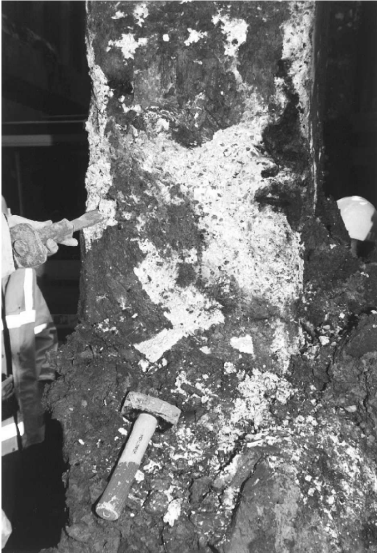
Figure 8.14 Extreme example of TSA in a Tredington–Ashchurch Bridge column exposed to wet, reworked Lower Lias Clay.
