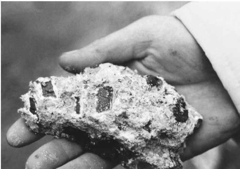
Figure 8.15 Hand specimen of deteriorated Tredington–Ashchurch Bridge foundation concrete showing the white haloes of thaumasite around the dolomite coarse aggregate particles.
