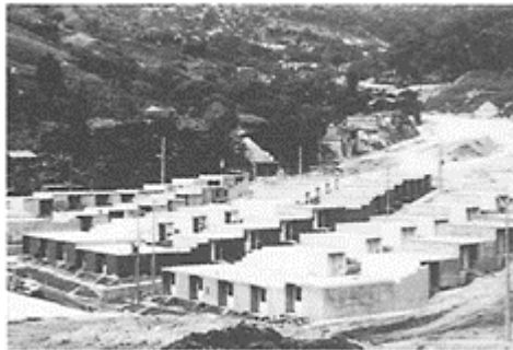
Figure 2. Low-income one-floor housing project (concrete walls), as built. Medellín, Damato, 1984.
