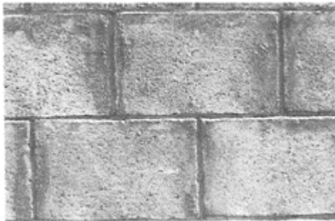
Figure 10. 250×400 mm “tall blocks” used for low to medium cost housing
