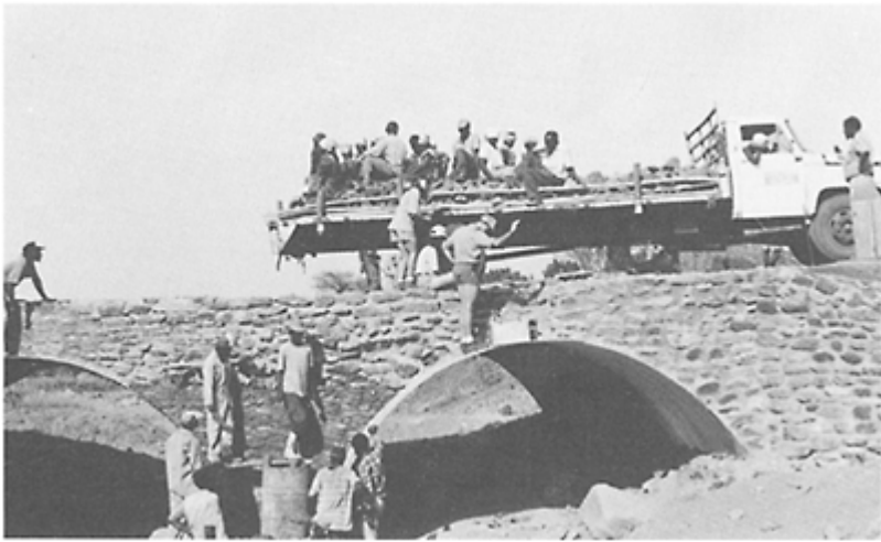
Figure 4 Live-load-induced strain test
