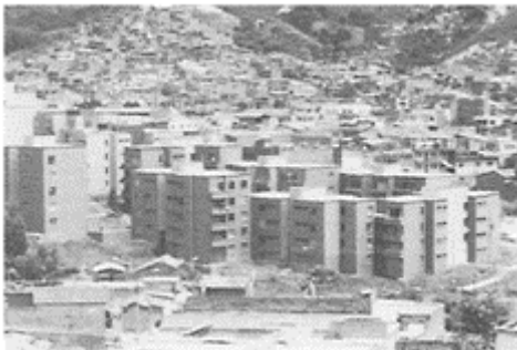
Figure 17. “Nueva Andalucía”. 5-floor apartment buildings. Medellín, Bravo- Restrepo, 1978.
