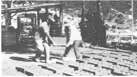
Figure 11. “Altos de la Villa”. On-site production of concrete blocks. Medellín, PSI, 1993.
