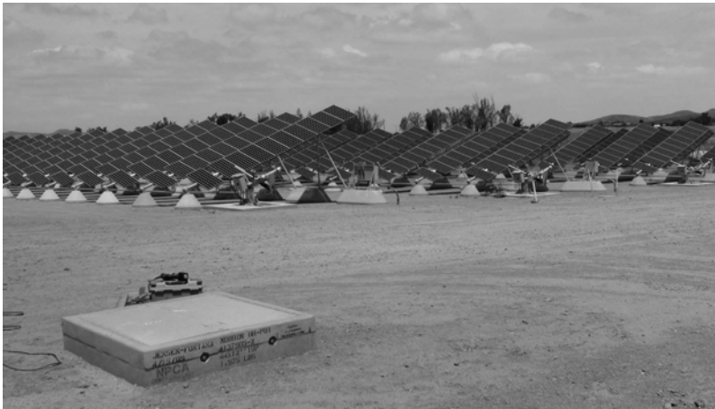
Figure 3.16. A single axis tracking solar power system
