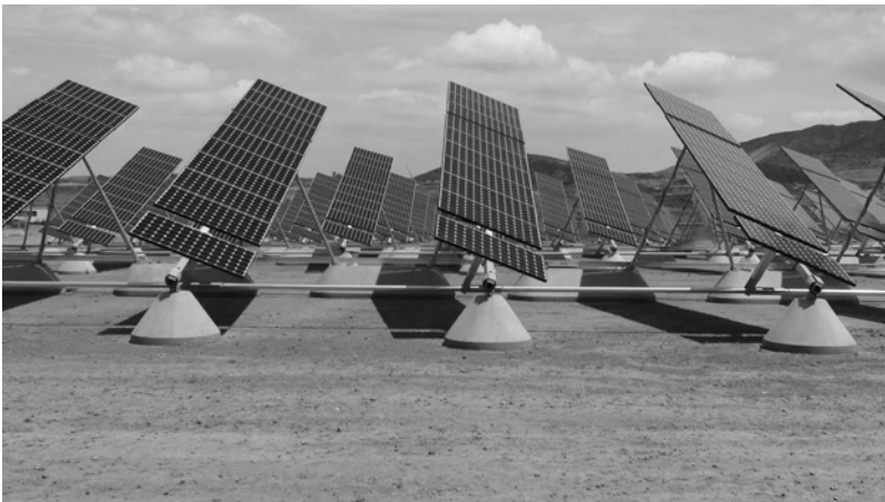
Figure 8.21. A single axis solar power system.
