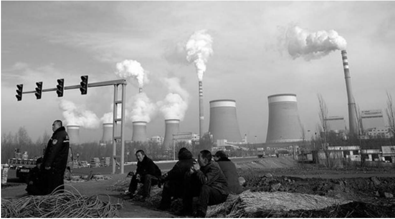
Figure 9.1. Carbon dioxide emission from coal fired electrical power generation plants.
