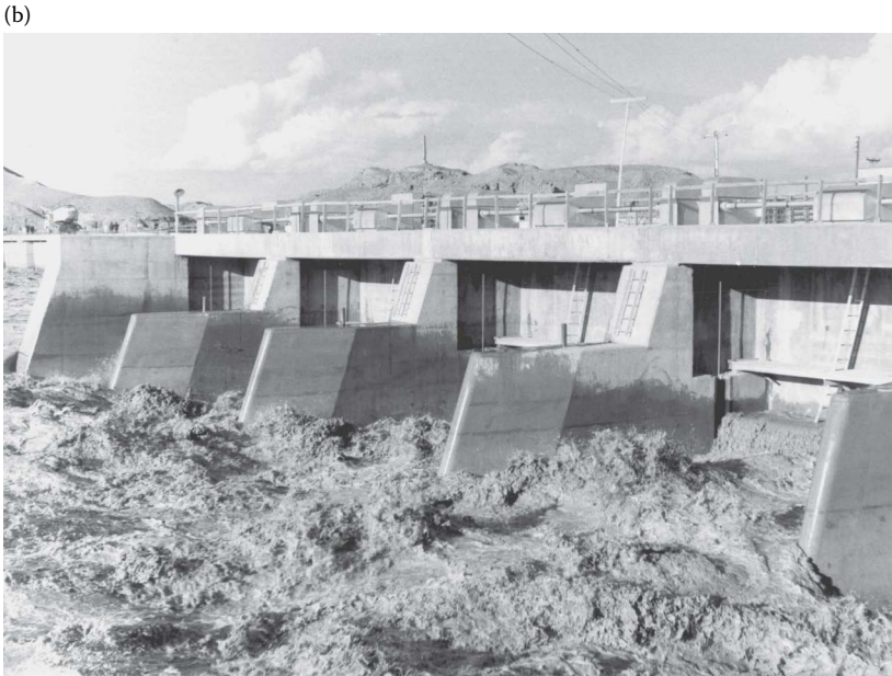
Figure 5.4 Using energy and continuity. (a) 'Free' flow under a sluice gate. (b) Sluice gates controlling discharge into irrigation canal, Iraq.
