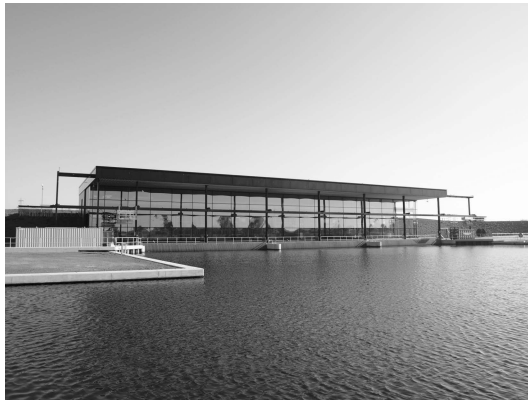
Figure 8.1 St Germans land drainage pumping station in Norfolk, UK.
