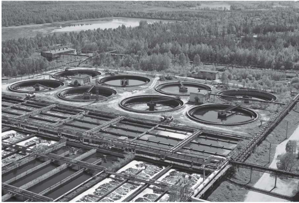
Figure 8.4 Typical layout of sewage treatment works.
