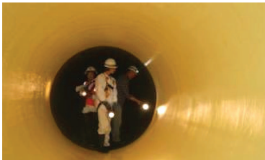
Fig. 5-18. Final appearance of top-coated FRP liner
