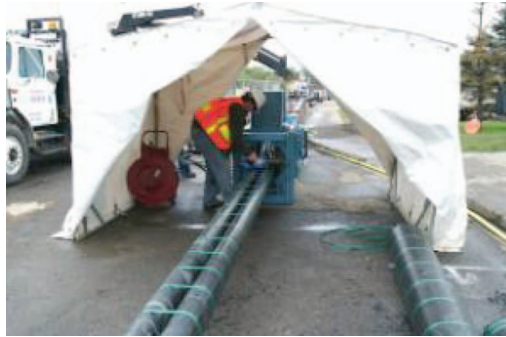
Fig. 5-12. Site-folded HDPE liner
