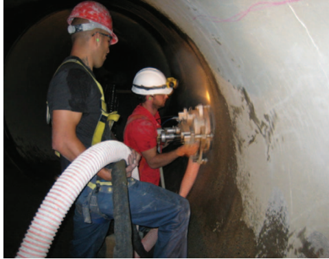
Fig. 5-15. Surface preparations on concrete substrate: cleaning using ultra-high-pressure water blasting
