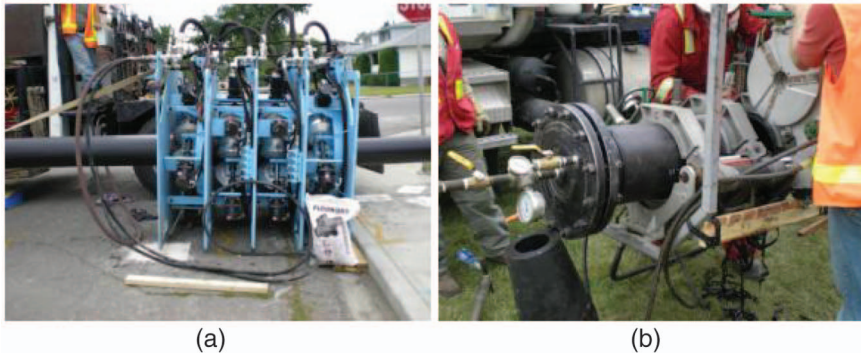
Fig. 5-11. (a) Roller-based symmetrical reduction liner machine; (b) fusing expansion head for symmetrical reduction process
