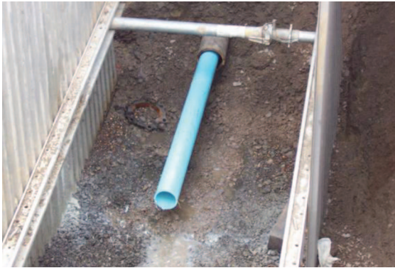
Fig. 5-13. Starting stock inserted in host pipe
