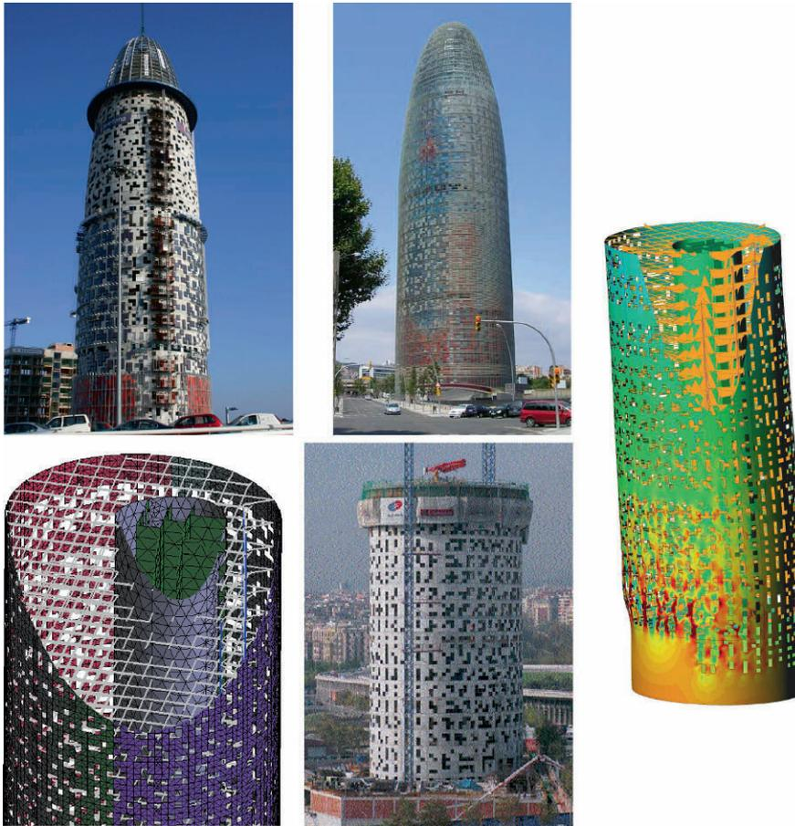
**Fig. 1.6** FEM analysis of the Agbar tower (Barcelona). Actual structure and discretization into shell and 3D beam elements. Deformed mesh (amplified) under wind load. Images are courtesy of Compass Ingeniería y Sistemas SA, [www.compassis.com](http://www.compassis.com) and Robert Brufau i Associats, S.A. [www.robertbrufau.com](http://www.robertbrufau.com)
