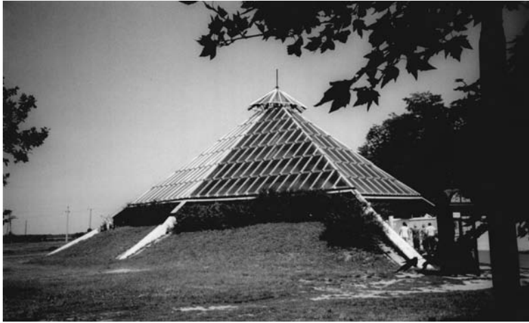
Fig. B5.2 A whole shelter/building and its specific but generic details. Remember the archetypal details and their inherent rules and you can check this example by bringing them into relation with each other.
