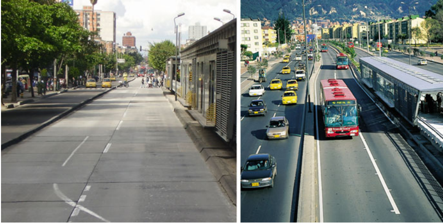
Fig. 10.4 Pictures show two lanes for transmilenio buses and two and three lanes for cars
