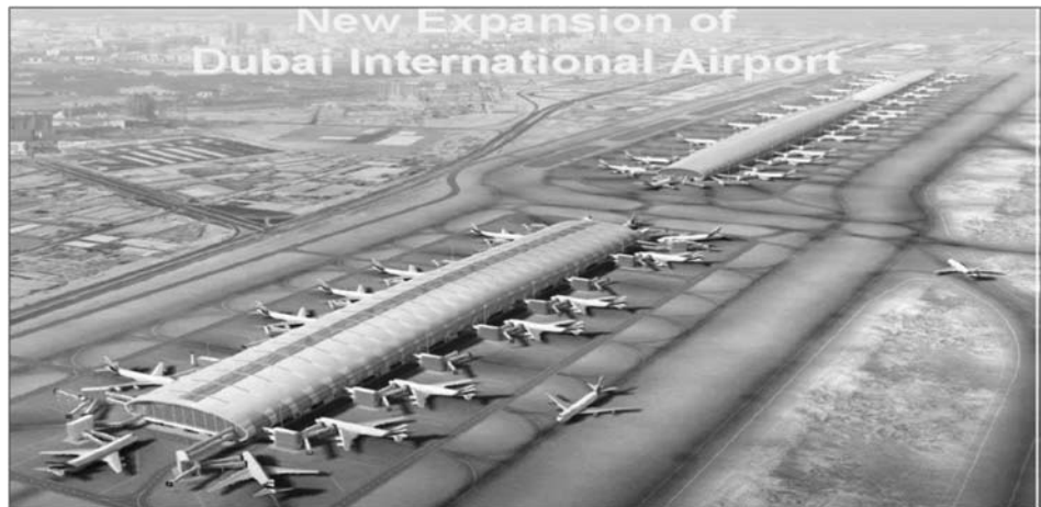
Figure 16.27 Concourses 2 and 3 of Dubai International Airport (13).
