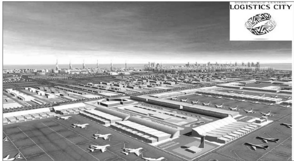
Figure 16.32 DWC Logistics City and Commercial City in the back (13).
