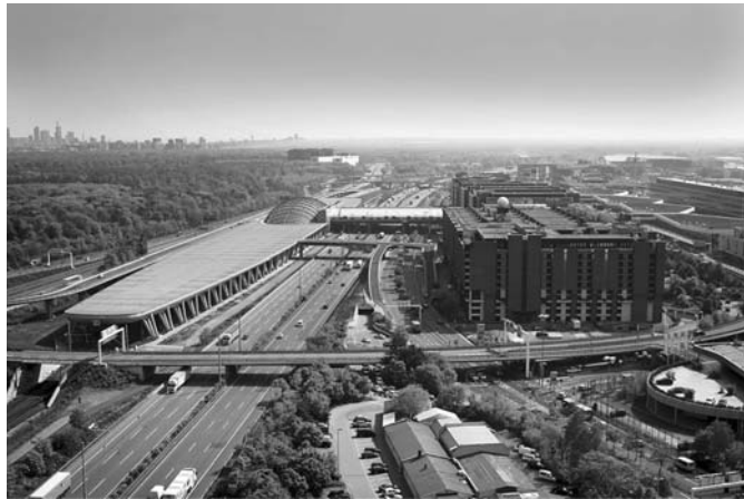
Figure 13.15(a) Landside access layout showing Fernbahn Station—Frankfurt Airport. (Courtesy of FRAPORT, Flughafen Frankfurt/Main AG.)
