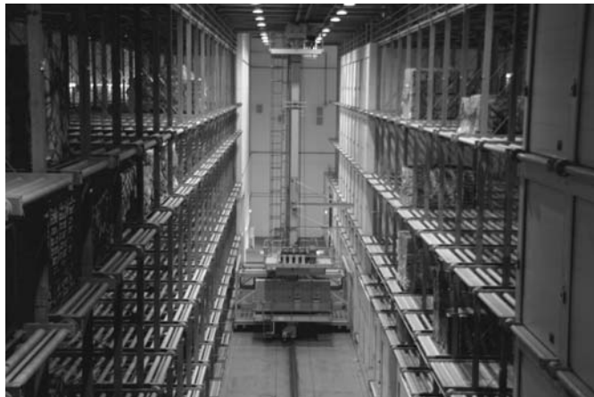
Figure 11.2 Modern ETV system. (Courtesy of ICM Airport Technics.)
