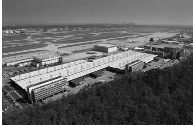
Figure 11.5 Lufthansa cargo center Frankfurt. (Courtesy of Lufthansa German Airlines.)
